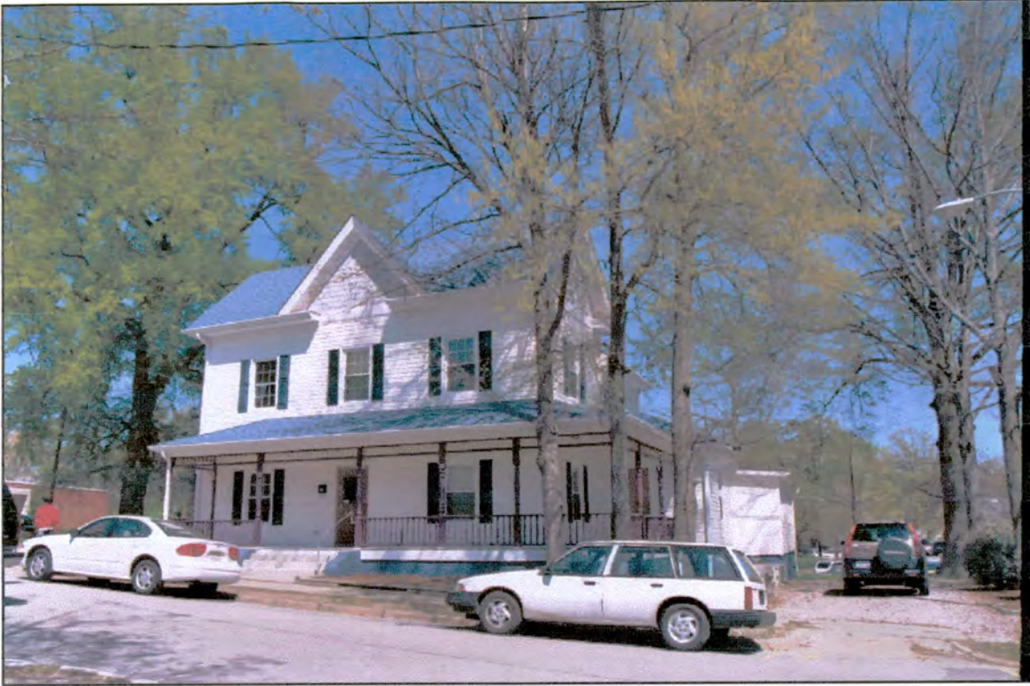
12. Reddick House, 8 Ferndell Street
