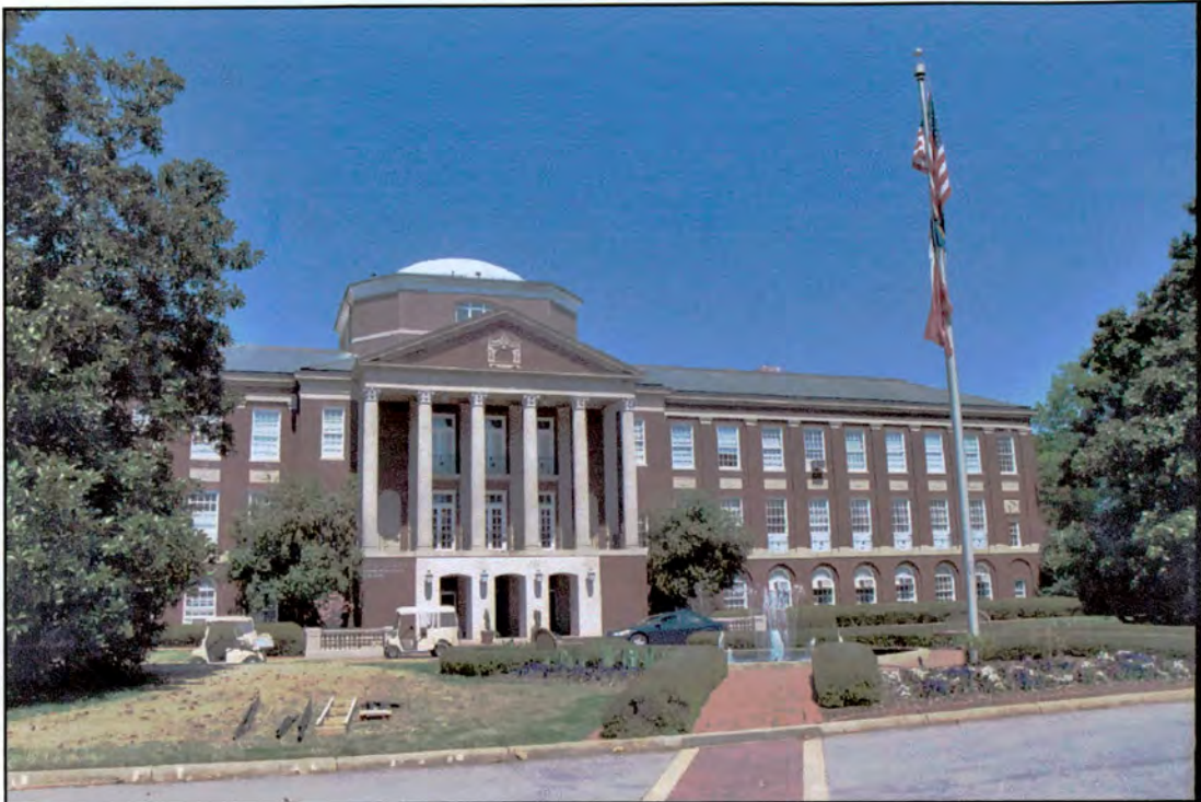
Meredith College Quadrangle, Johnson Hall facade (south elevation)
