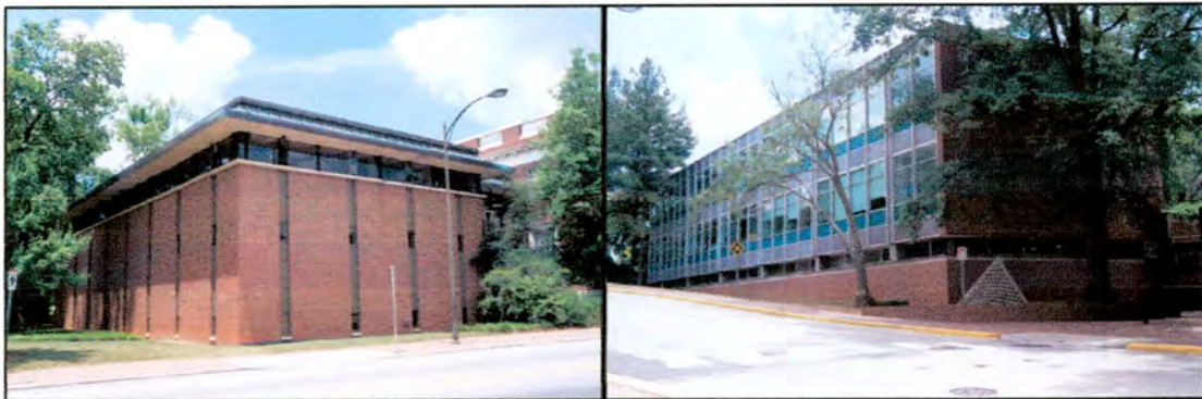
L. Brooks Hall (top), with south addition (lower left) and north addition (lower right)
