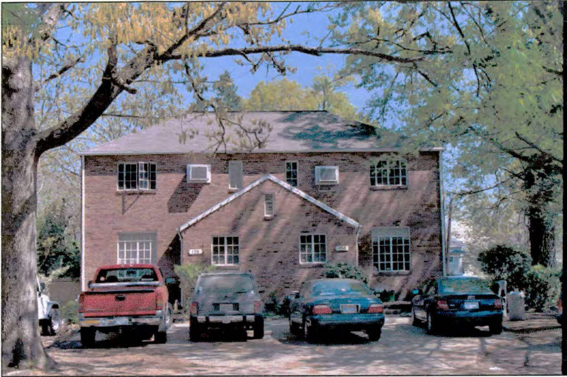
18. Duplex, 126-128 Groveland Avenue
