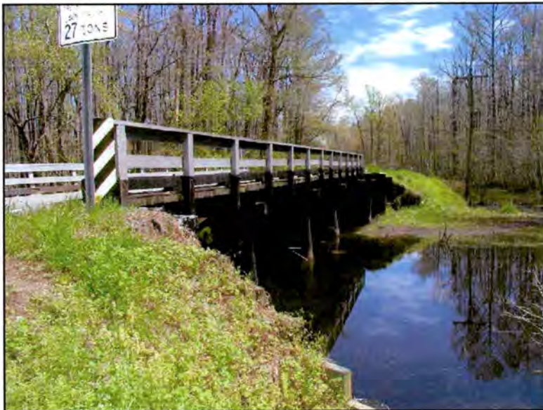
Figure 22. Bridge No. 32 on SR 1100 over Trotman Creek.
