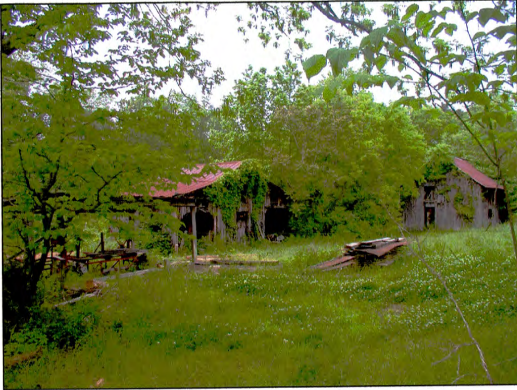
Figure 18. Springer sawmill shed (C), feed barn (D), and barn (E), looking northwest.
