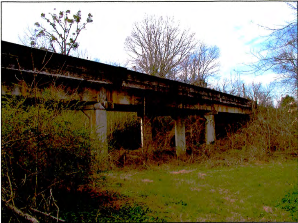
Figure 3. Bridge No. 307 looking northwest.
