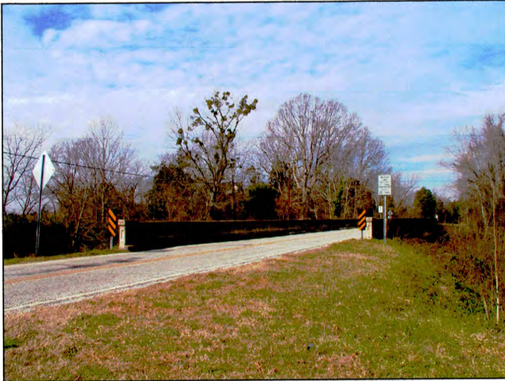
Figure 5. Bridge No. 307 looking northwest.
