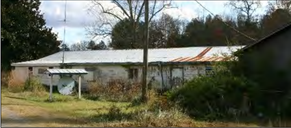
Figure 6: McKenzie Millwork and Machinery Company, front elevation with signage. Courtney Foley, NCDOT, November 2008.
