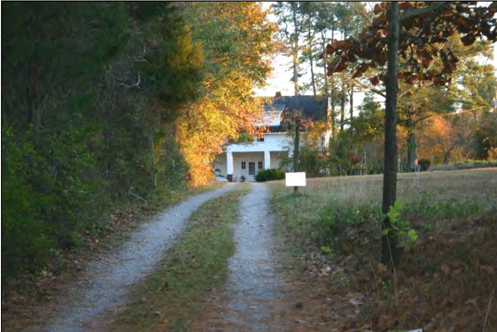
Figure 8: Frye House, 3895 US 15-501. Penne Sandbeck NCDOT, November 2008
