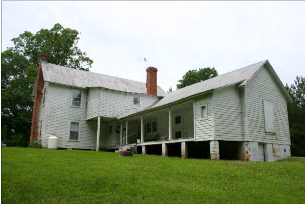
Figure 13: North and east elevations, Fields-Callaway House (upper shed on poles is early 20 th century bathroom, no longer used)
