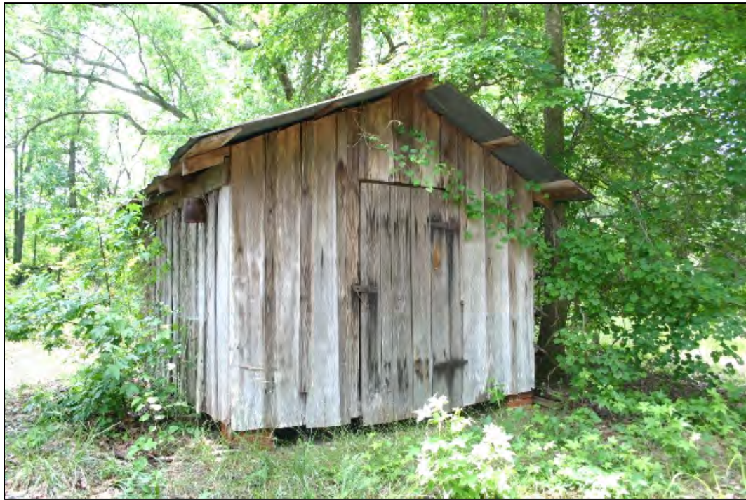
Figure 56: Tenant house smokehouse
