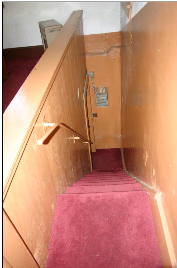
Figure 34: Stairs to basement from sanctuary
