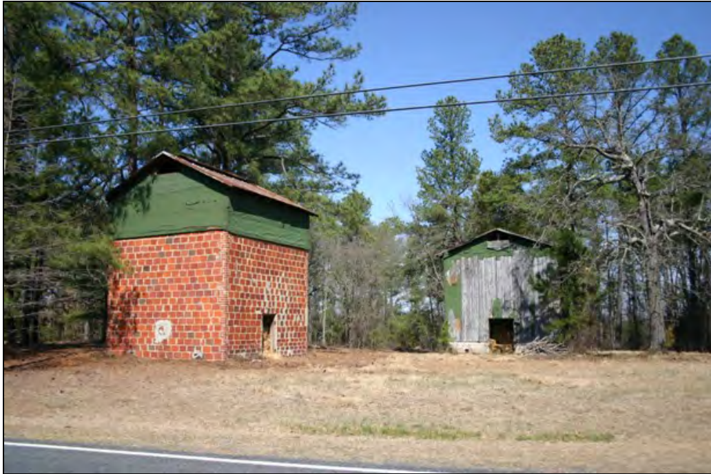
51. Stage Road, no address (across road and .1 mile W of 595 Stage Road) PIN 858804801170
