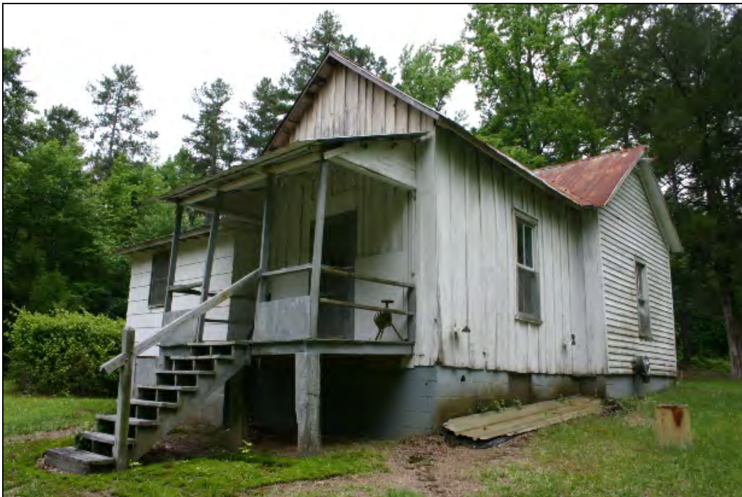
Figure 75: Kelly-Muse Tenant House, rear (east) elevation
