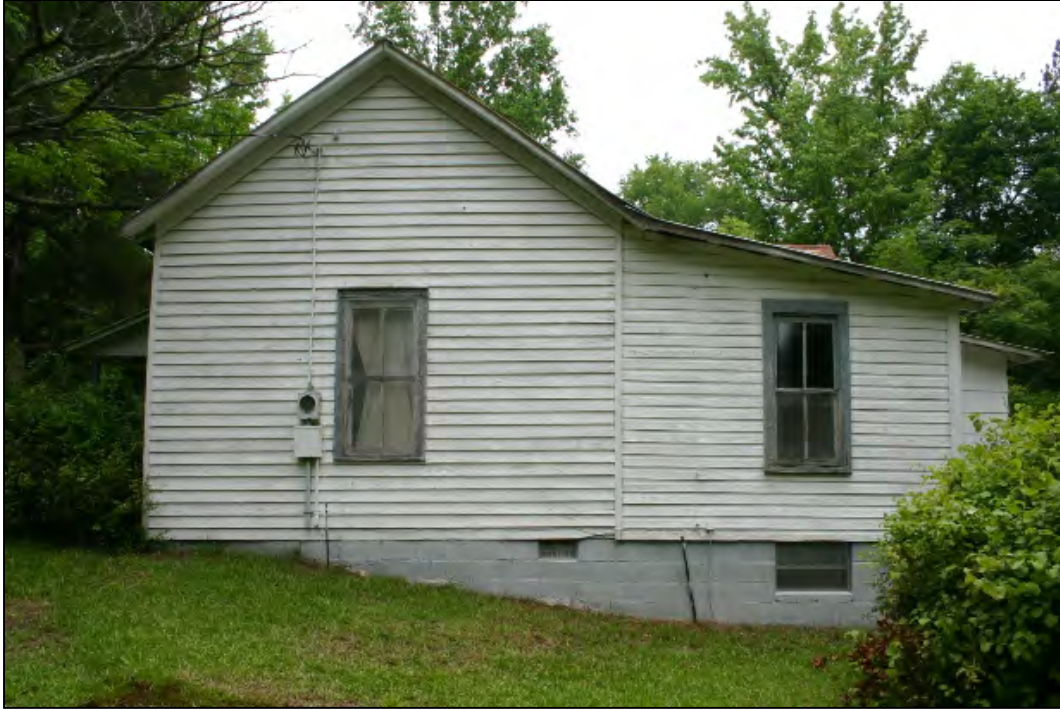
Figure 76: Kelly-Muse Tenant House, south elevation
