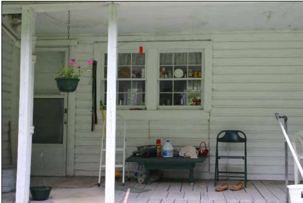
Figure 19: Fields-Callaway House, detail of ell-kitchen porch
