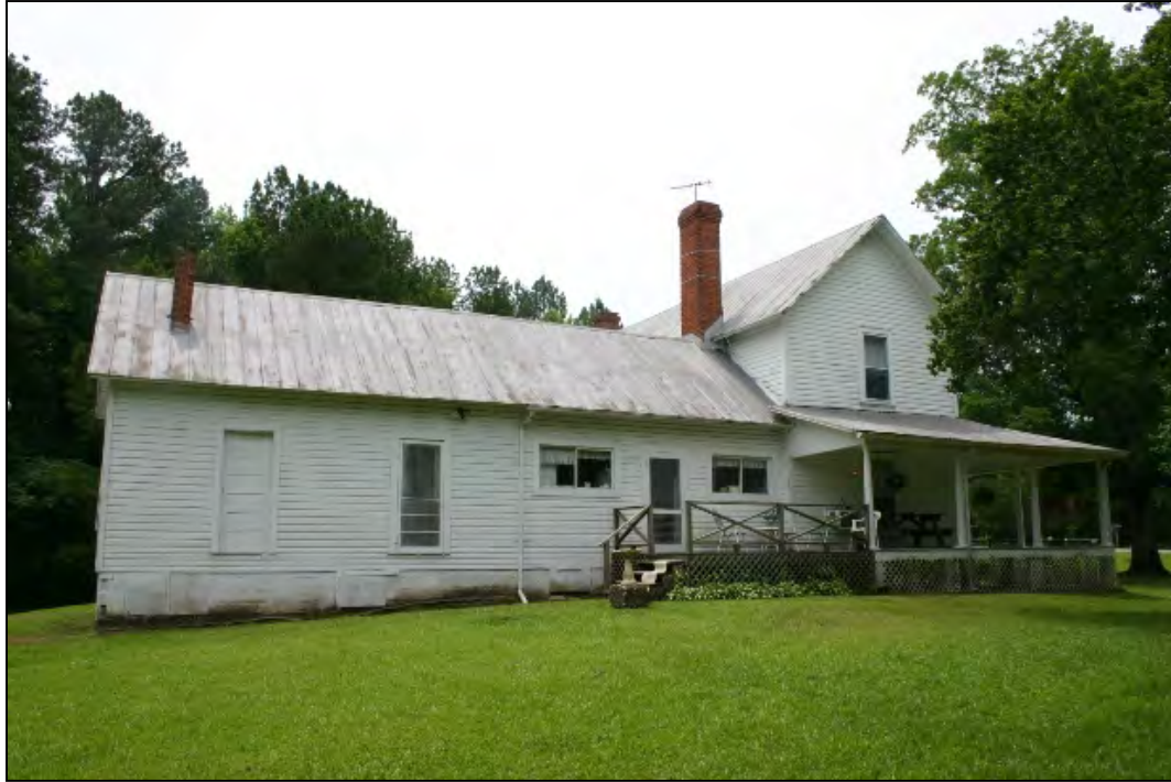
Figure 15: Fields-Callaway House, west elevation
