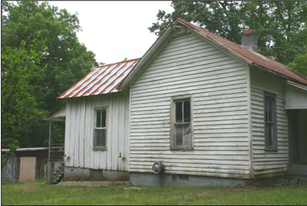
Figure 74: Kelly-Muse Tenant House, north elevation
