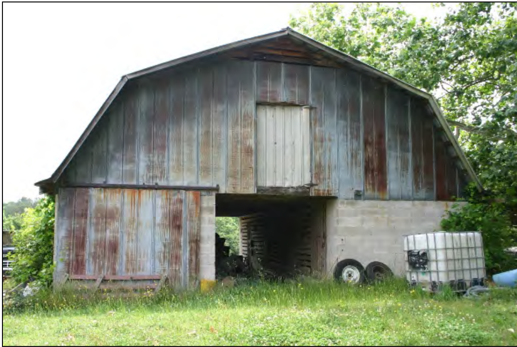
Figure 47: Shields Farm, Dairy barn
