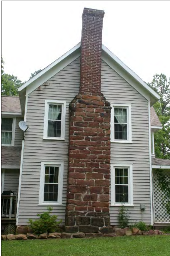
Figure 61: Kelly-Muse House, South elevation chimney
