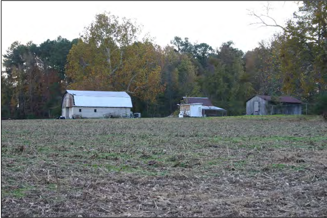
Figure 57: Shields Farm, overall view showing dairy barn, packhouse, and shed from fields
