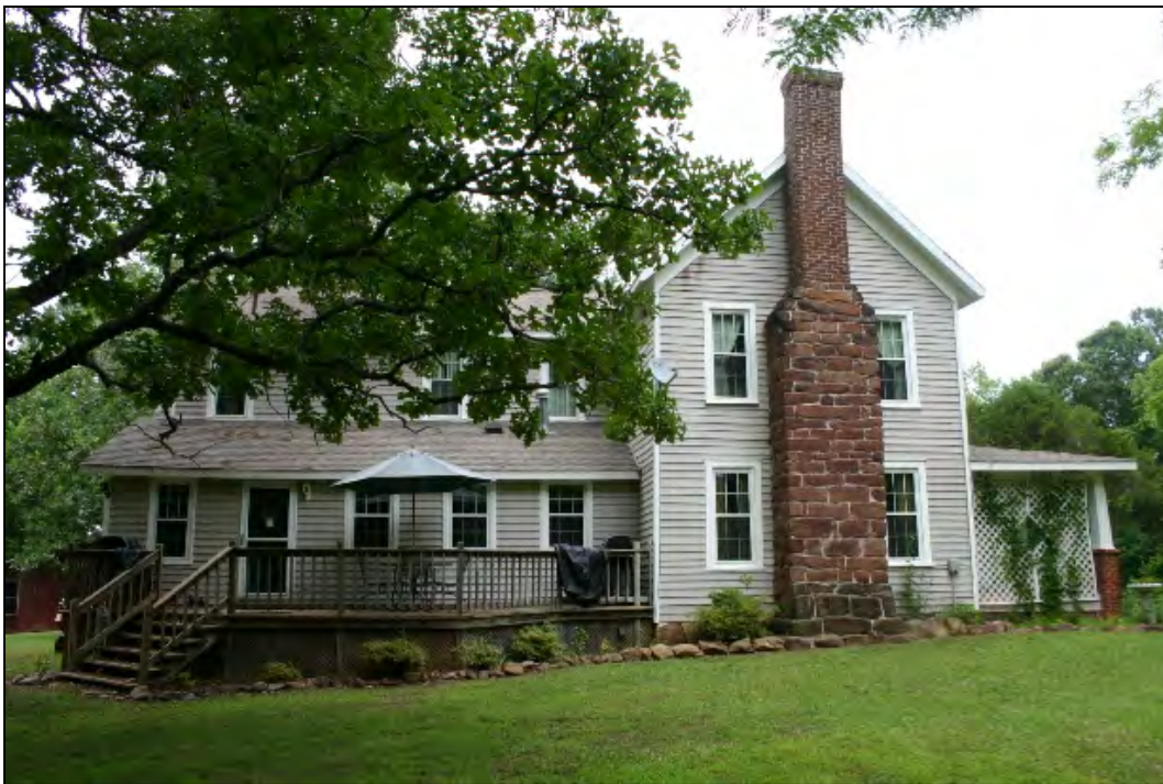
Figure 58: Kelly-Muse House, south elevation
