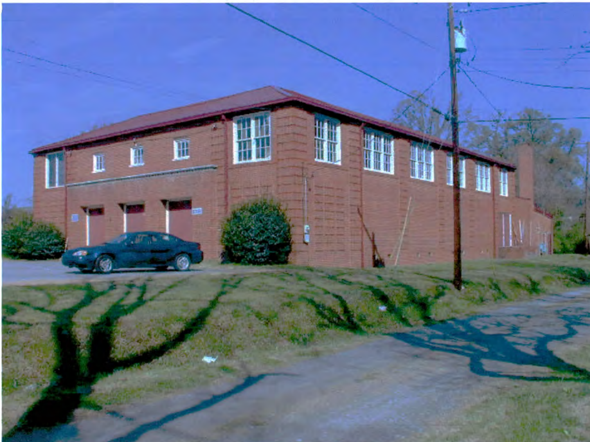
#4 Derita School Gymnasium 6115 Rumple Rd.
