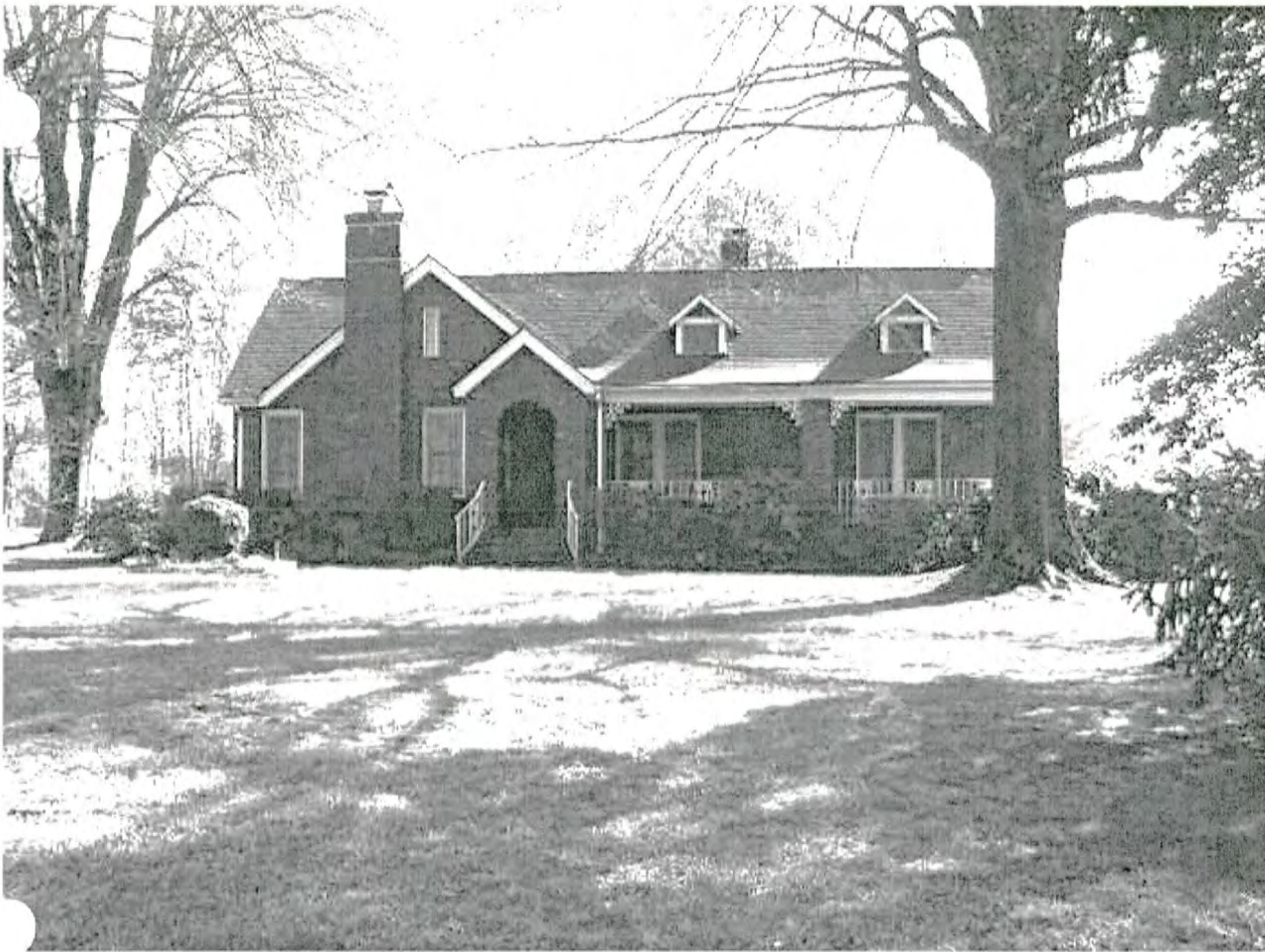
#3 House 2208 Sugar Creek Rd.
