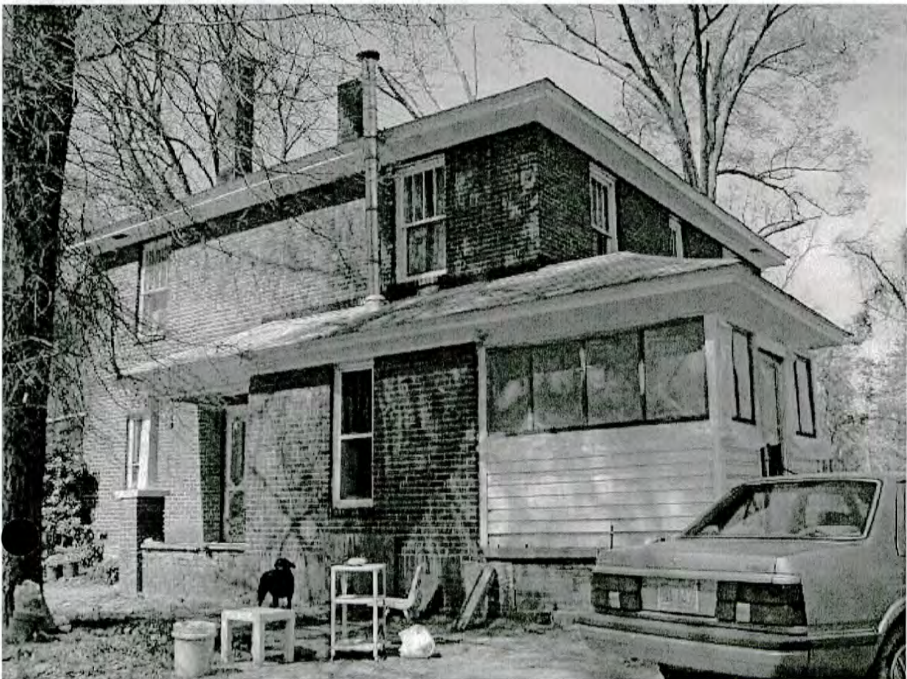
#31 House 6604 Mallard Creek Rd. Determined Not Eligible 04-05-2004
