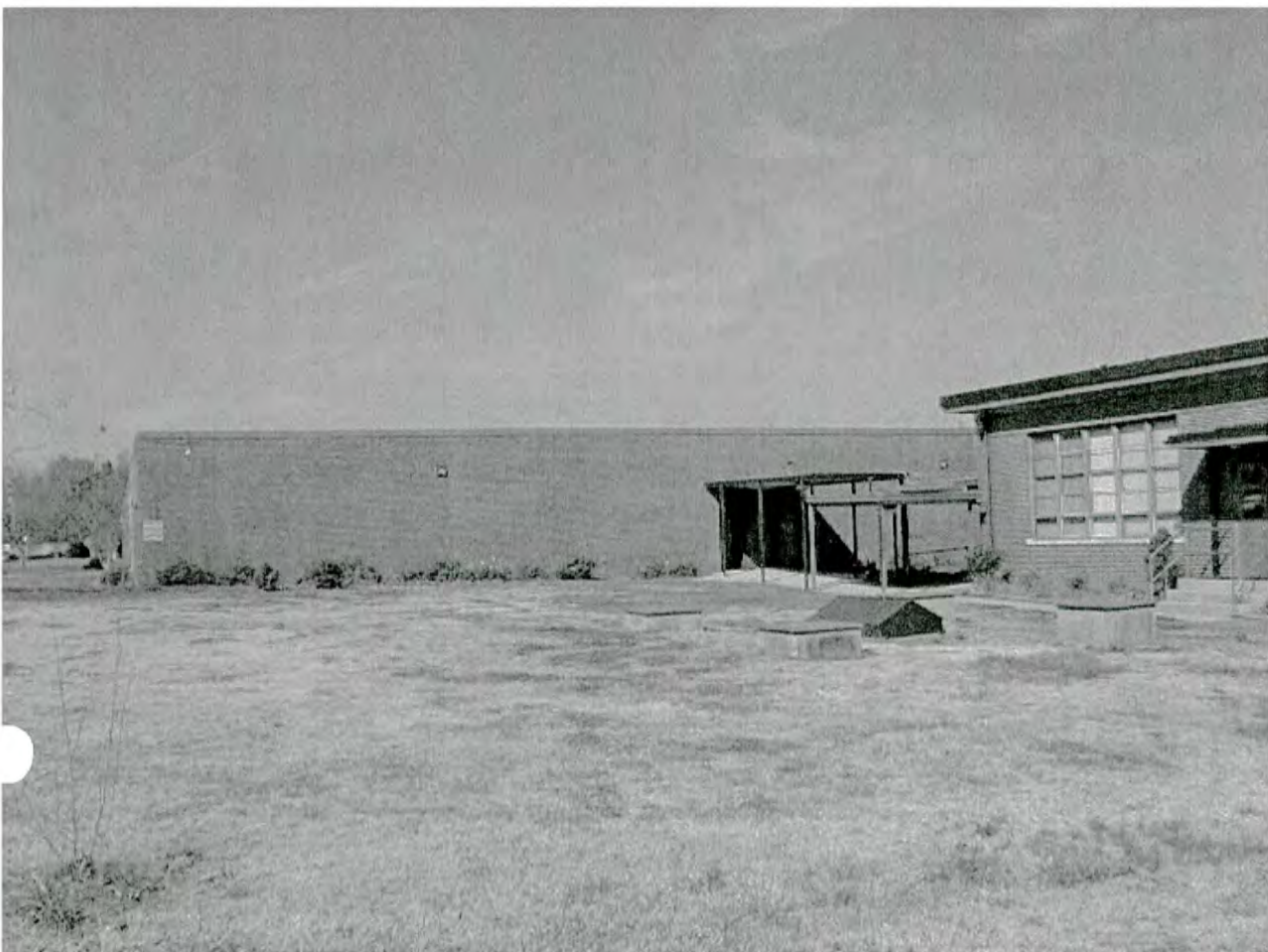
#4 School: Main Bldg. Rumple Rd.
