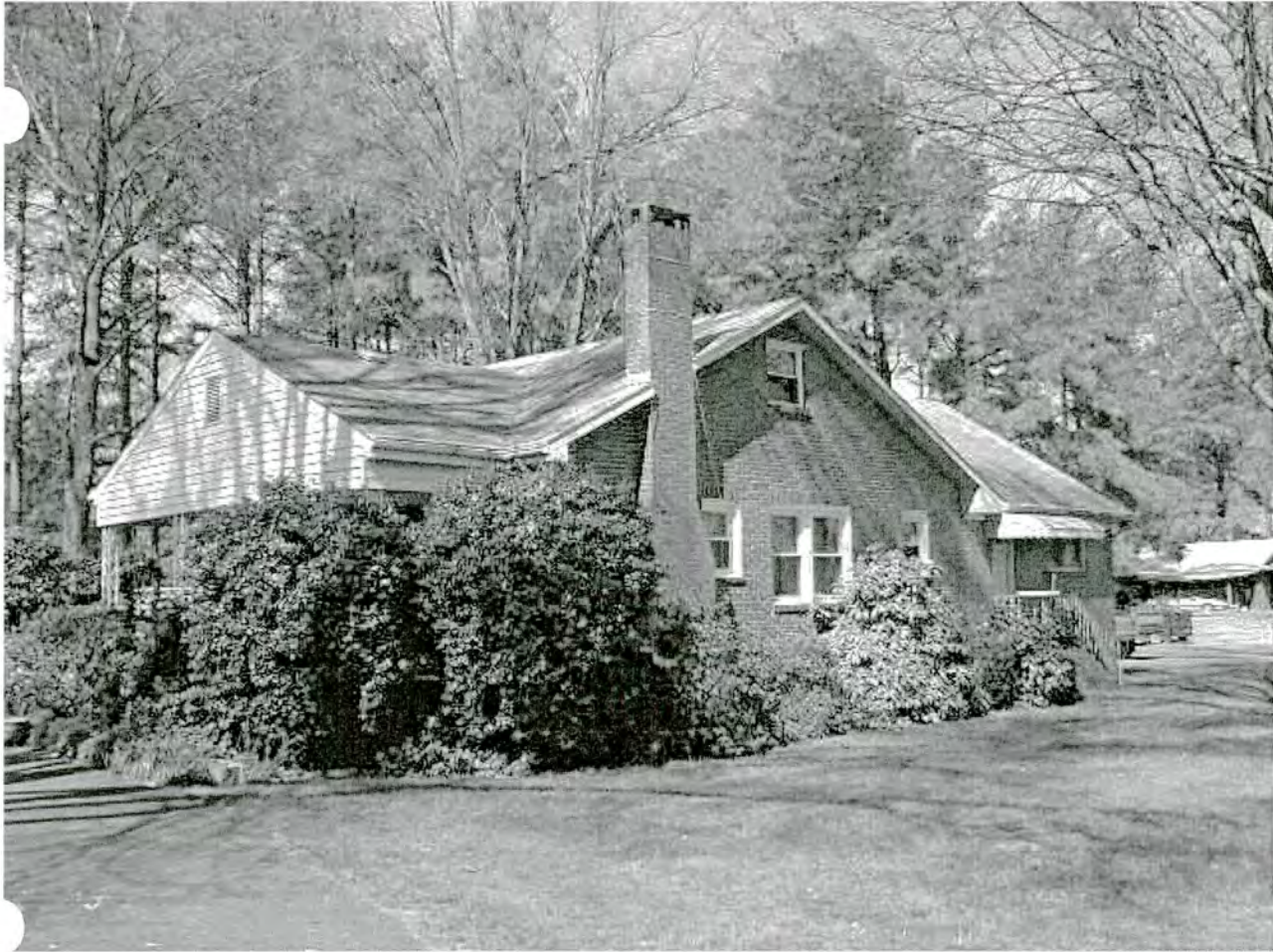
#38 House 7539 Mallard Creek Rd. Determined Not Eligible 04-05-2004
