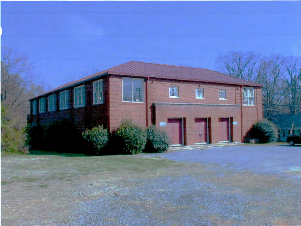
#4 Derita School Gymnasium 6115 Rumple Rd.
