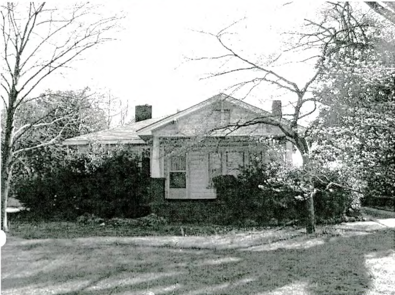
#2 House 2200 Sugar Creek Rd.
