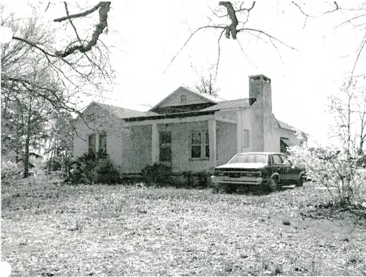
#37 House Mallard Creek Rd.
