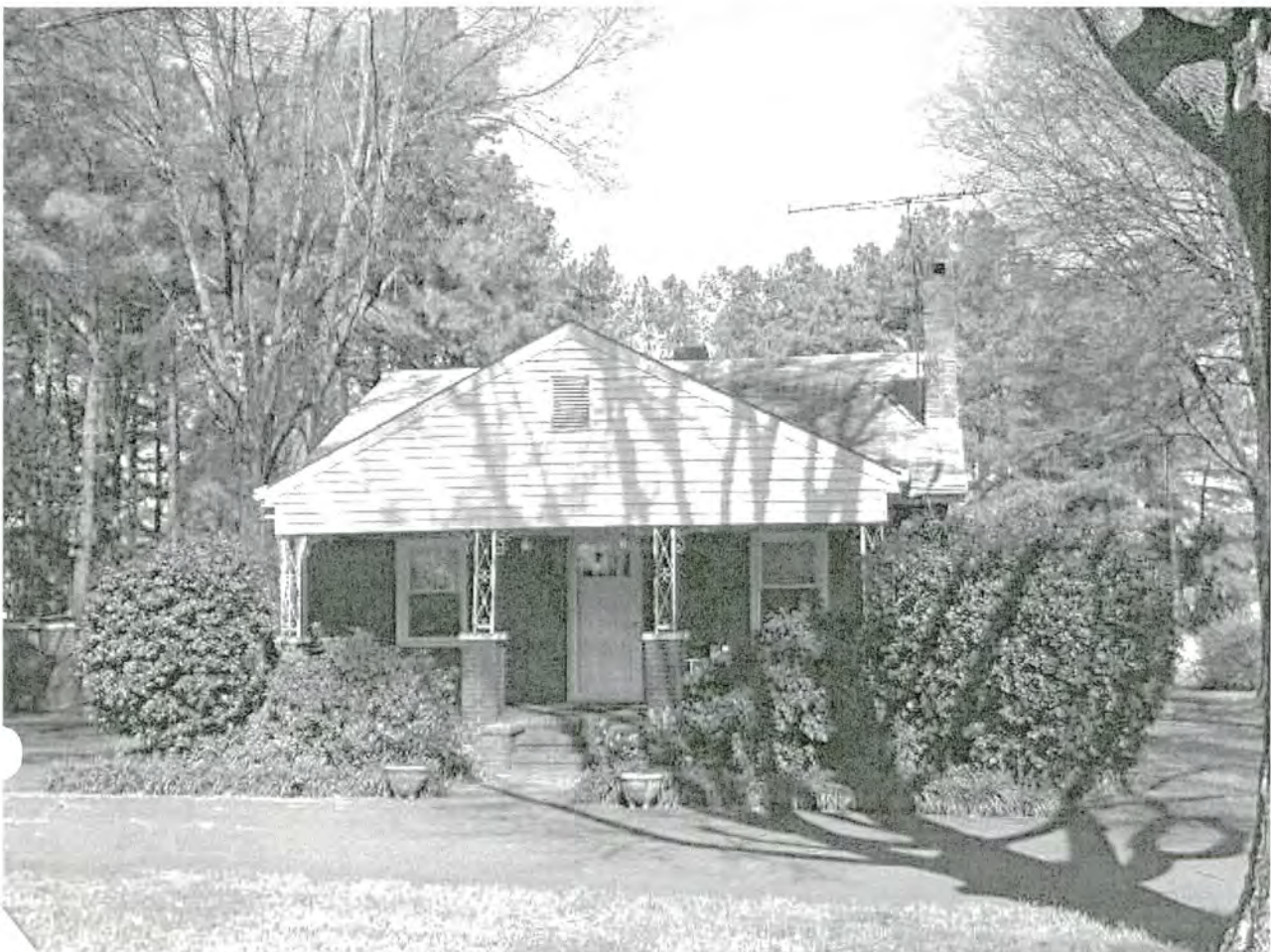
#38 House 7539 Mallard Creek Rd. Determined Not Eligible 04-05-2004
