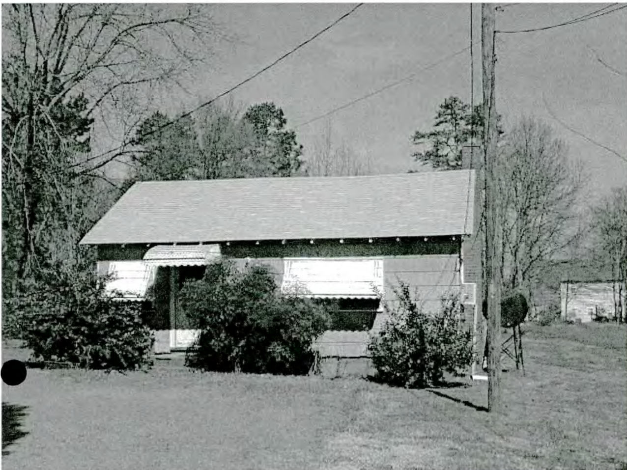
#36 House Mallard Creek Rd.
