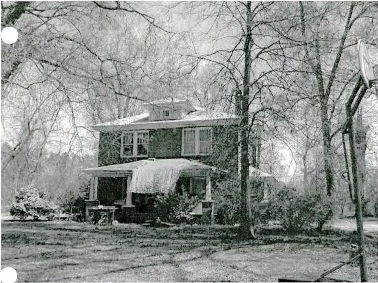
#31 House 6604 Mallard Creek Rd. Determined Not Eligible 04-05-2004
