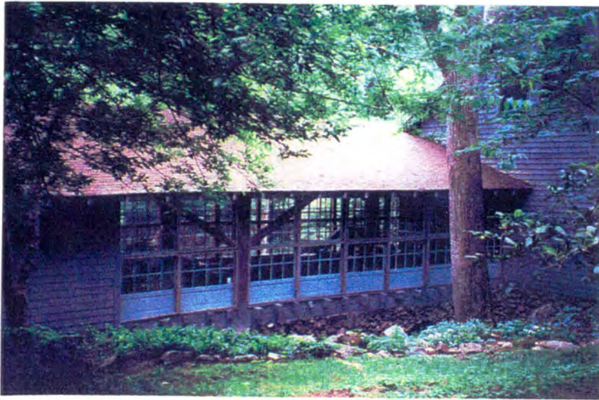
1b Northwest facade of former saw room
