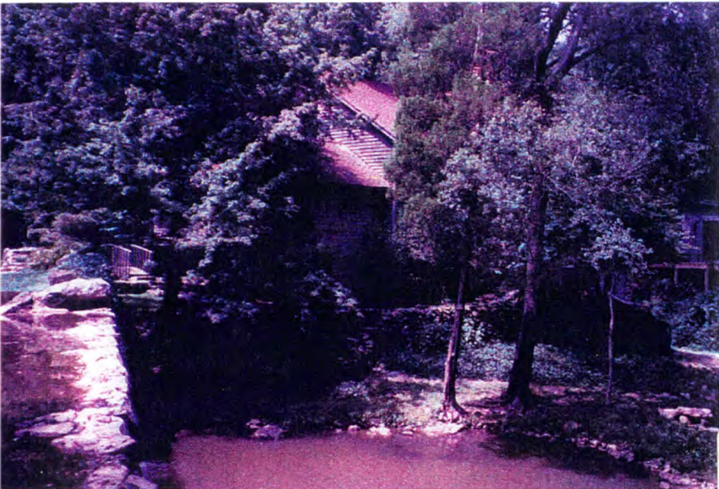
5b Rear (southeast) facade as seen from dam
