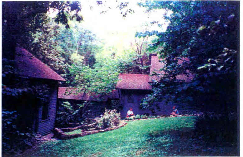
2b Northeast facade of guest house and porch room addition
