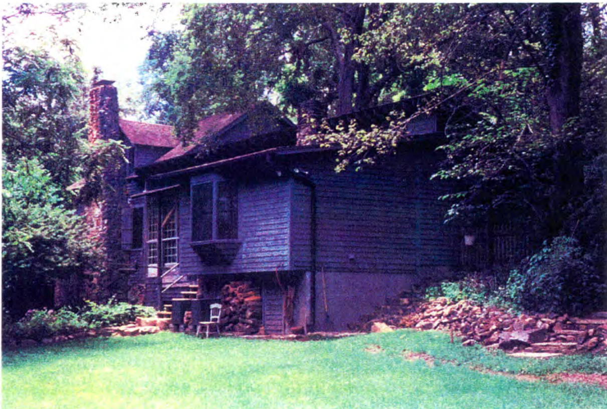
4b Rear (southeast) facade and northeast facade of breakfast room addition
