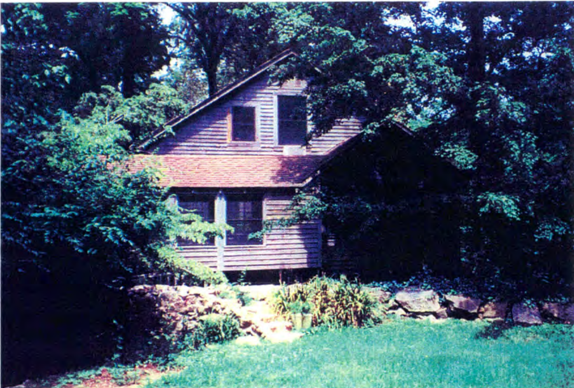
2c Southwest facade of former assembly building and porch room addition
