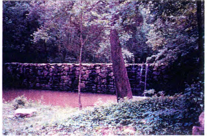
5c Stone dam wall
