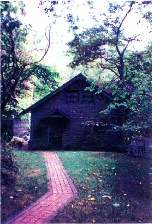
2a Front (northwest) facade of guest house
