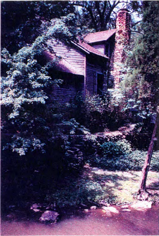
5a Rear (southeast) facade and stone chimney as seen from dam
