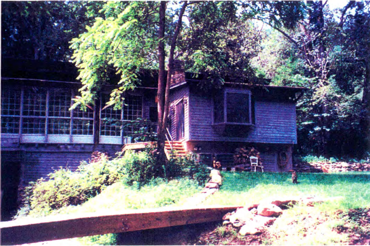
4a Rear (southeast) facade of former saw room and breakfast room addition
