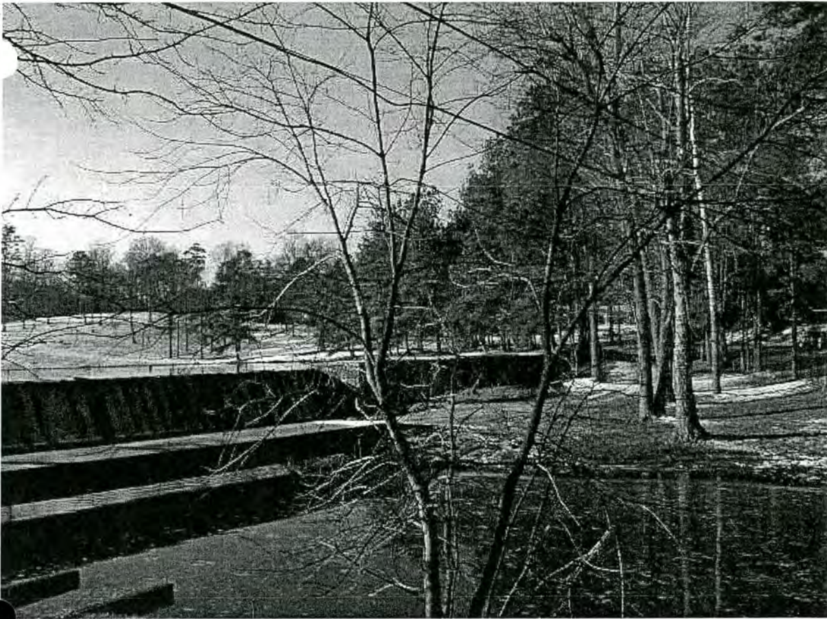
Property #2 Lake Neuseoca Dam
