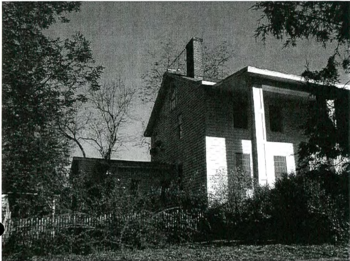
1.4 Sunnyside: Façade and side additions
