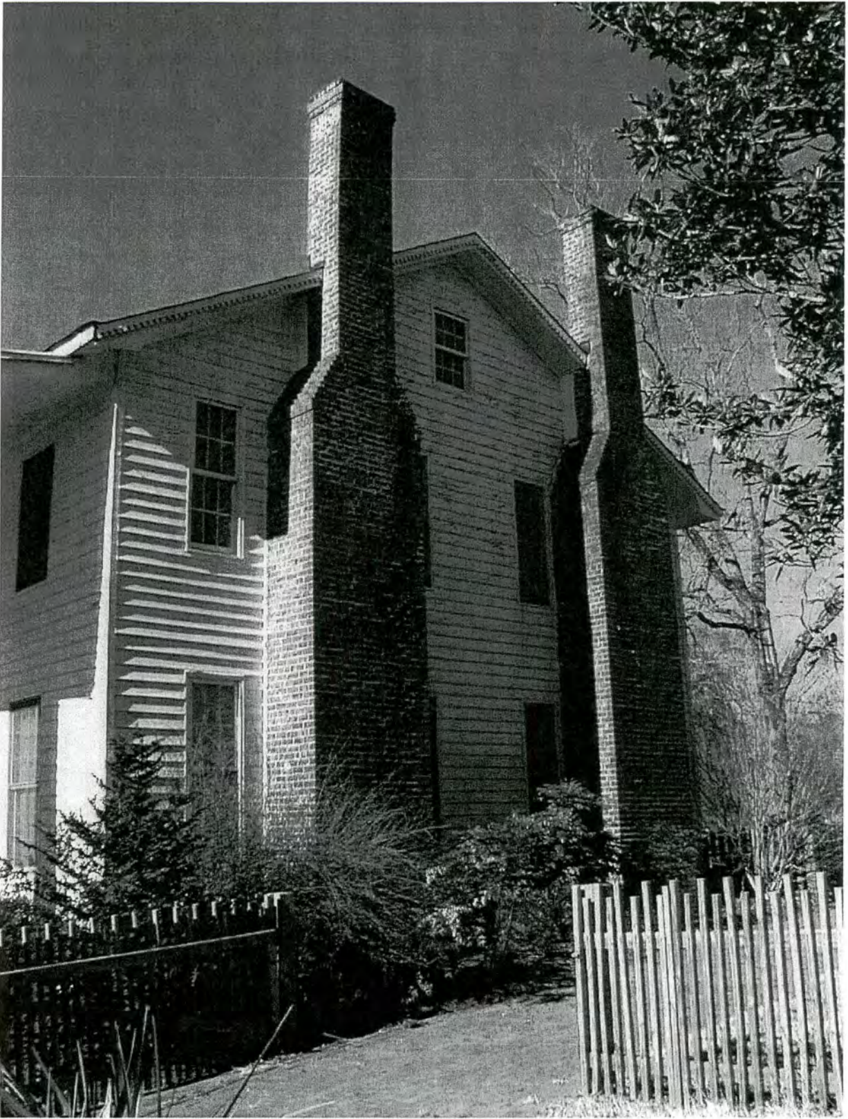
1.7 Side Elevation with end chimneys
