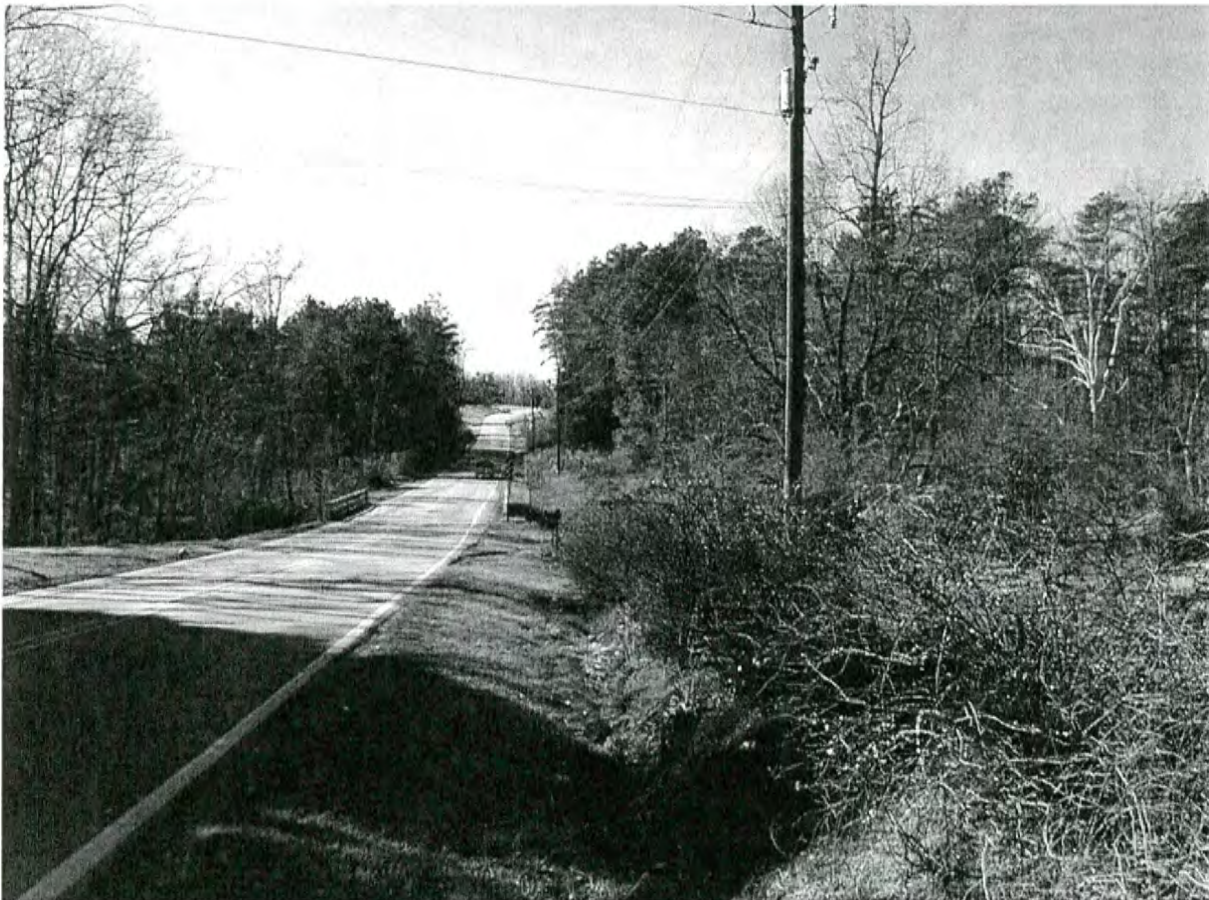
1.2 View of Bridge from Sunnyside property
