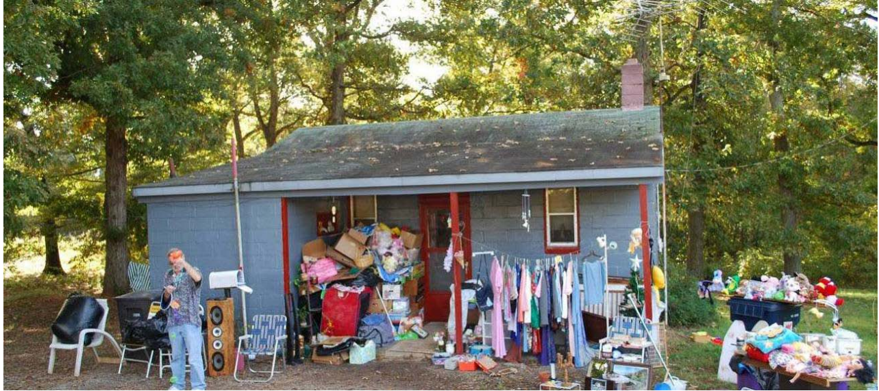
Tenant House, circa 1950s, 1437 Simonton Road, north elevation, looking south Contributing Building
