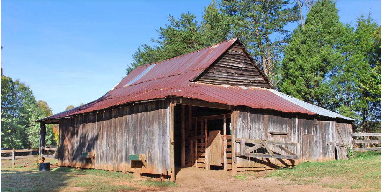
Barn, third quarter of the nineteenth century, Contributing Building southeast oblique view, looking northwest
