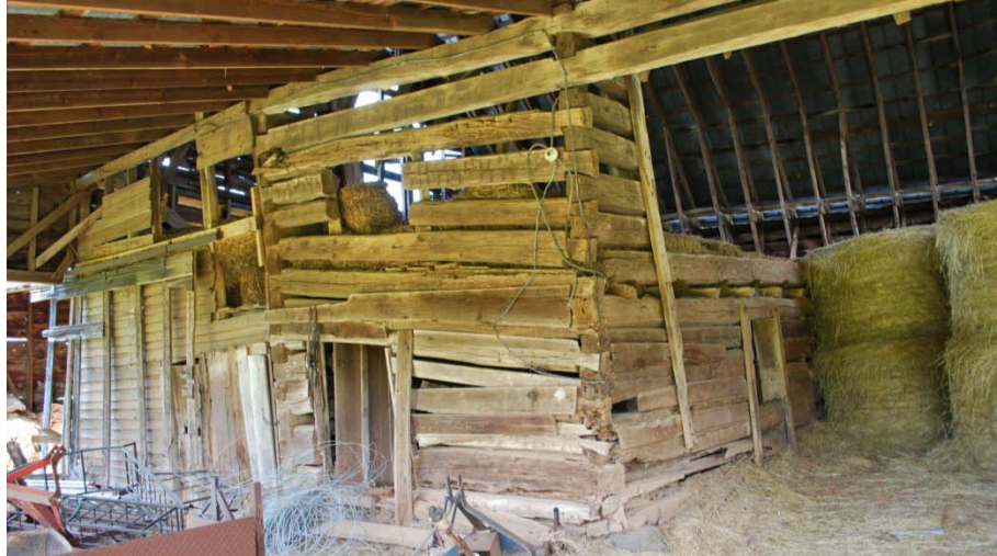
North section of the double-pen log barn on the Goodman-Wilkinson-White Farm (RW 1743)
