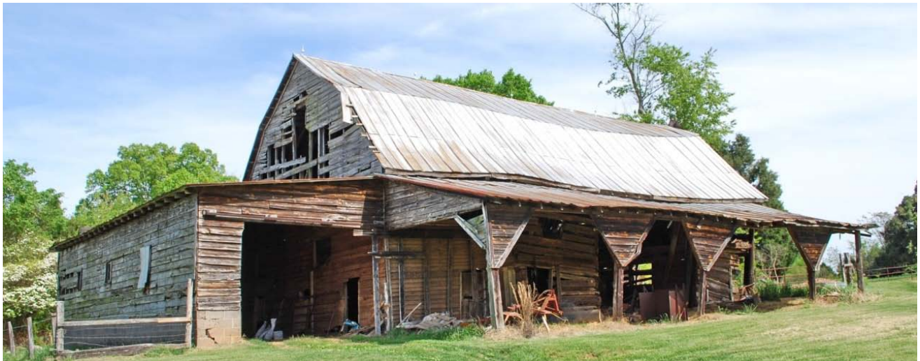
Mid-nineteenth-century double-pen log barn on the Goodman-Wilkinson-White Farm (RW1743) at 1430 Back Creek Church Road in the Mount Ulla vicinity
