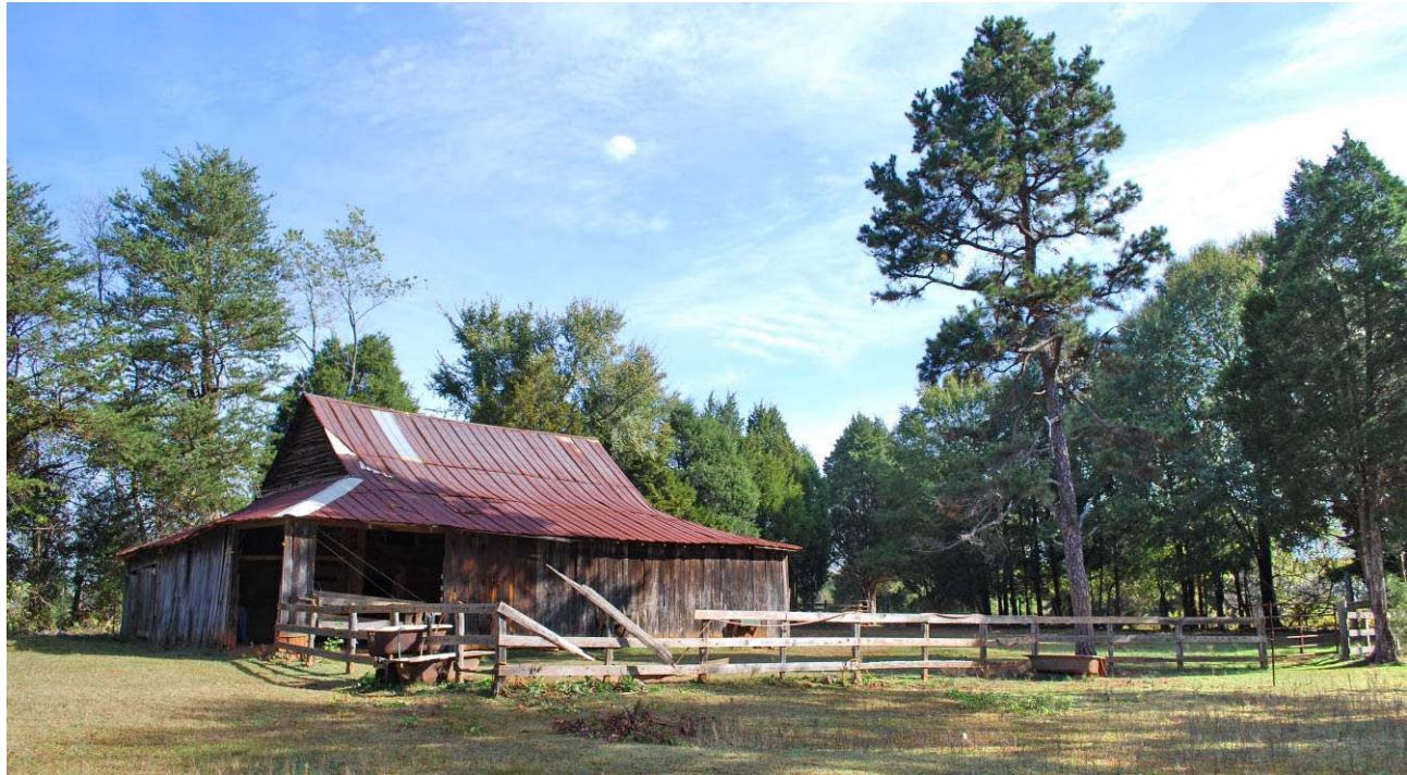
Log Barn and Pasture, looking northeast
