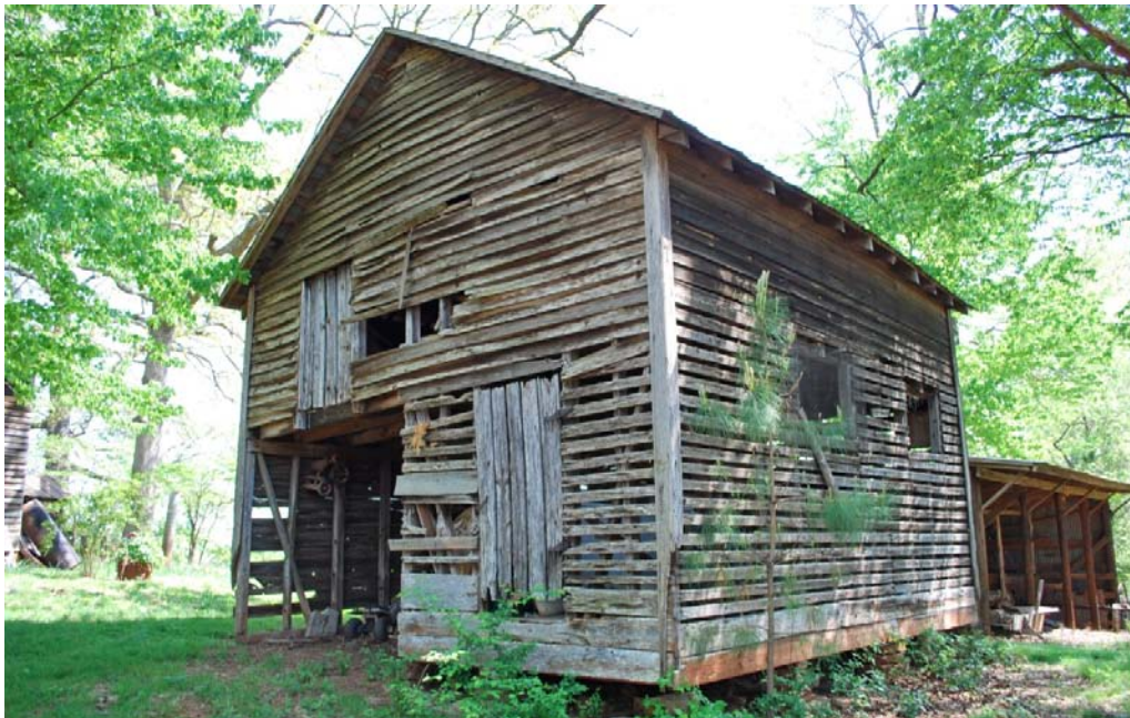
Circa 1920s corncrib/granary/equipment shed (ID1082), Farm, 289 Ford Farm Road, Central vicinity
