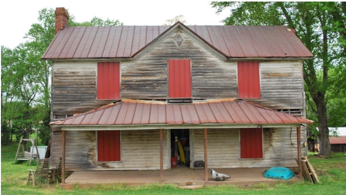
A. C. Plyler House (ID1076), 1915, 650 Shiloh Road, Statesville vicinity
