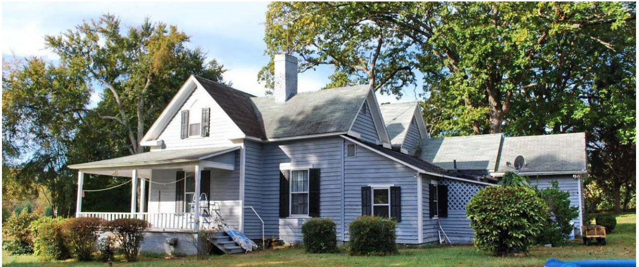
northeast oblique, looking southwest
