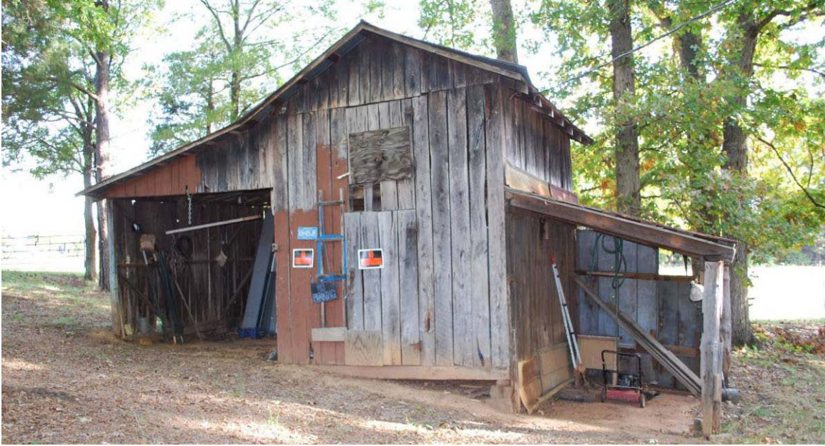
Shed, circa 1930s, southwest oblique, looking northeast, Contributing Building
