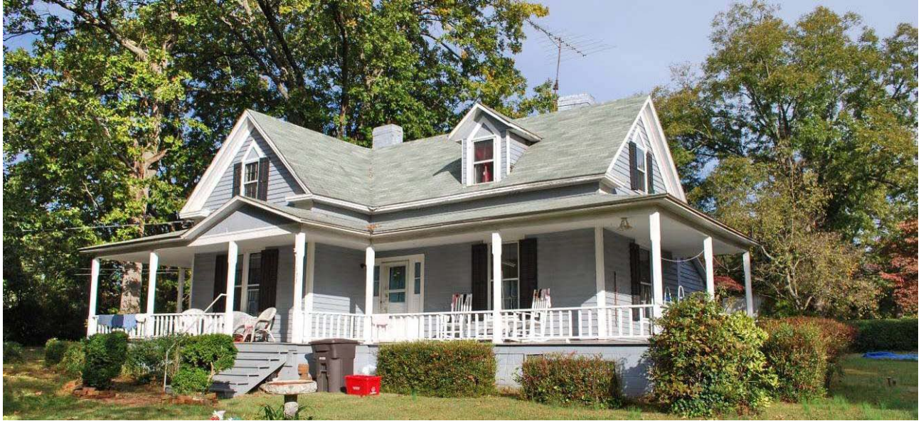
Ramsey House, ca. 1883, 1853 Norwood Drive, southeast oblique, looking northwest Contributing Building
