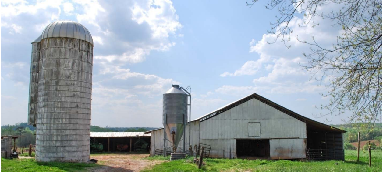
Concrete and metal silos on Cartner Farm (ID1085), 123 Cartner Road, Harmony vicinity
