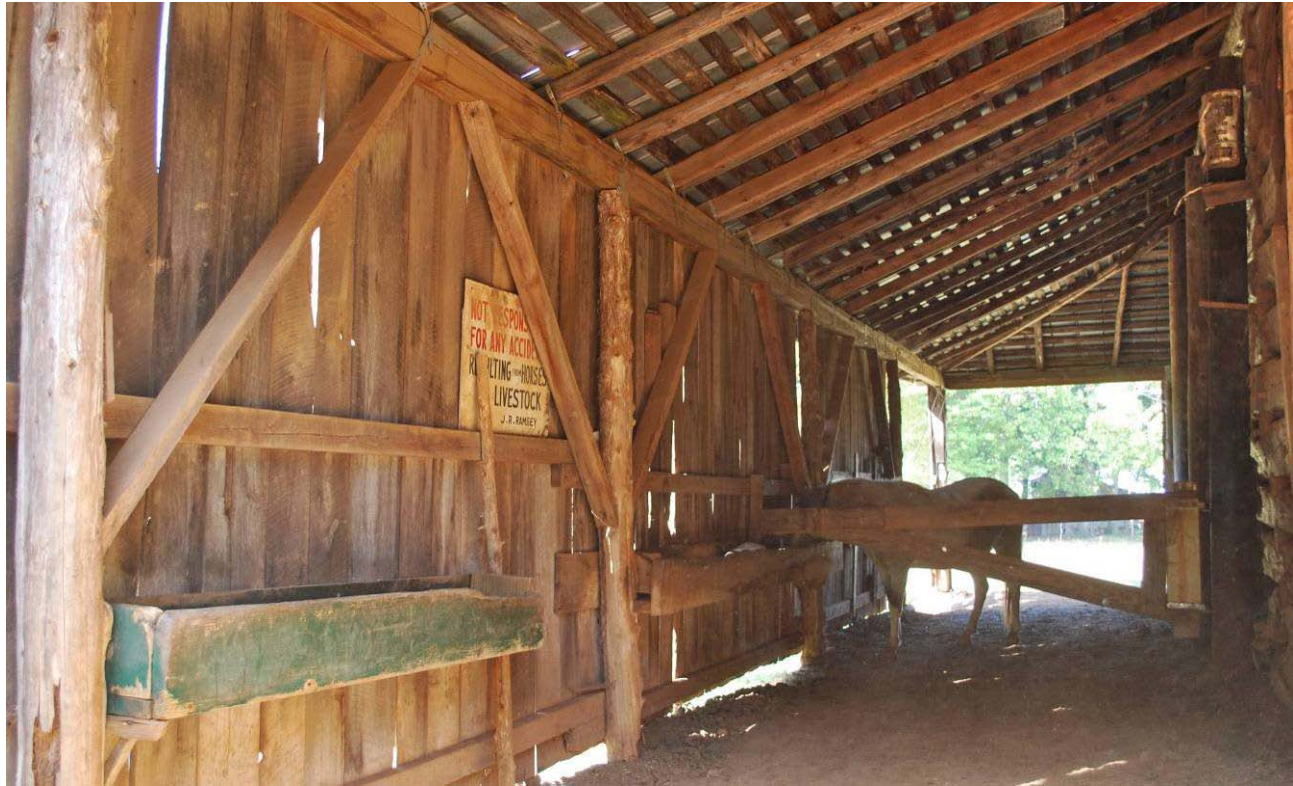
South shed, south wall, looking southwest
