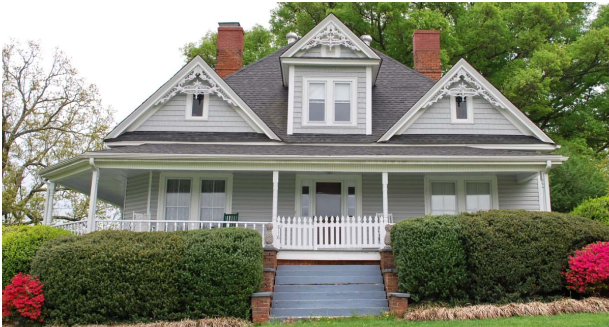
Pickney Alexander Shinn House (ID0840), early twentieth century, 816 Shinnville Road, Shinnville
