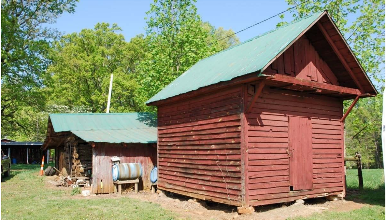
Log smokehouse with equipment shed additions (left) and frame smokehouse Hellard-Hartness Farm (ID1079), Central vicinity
