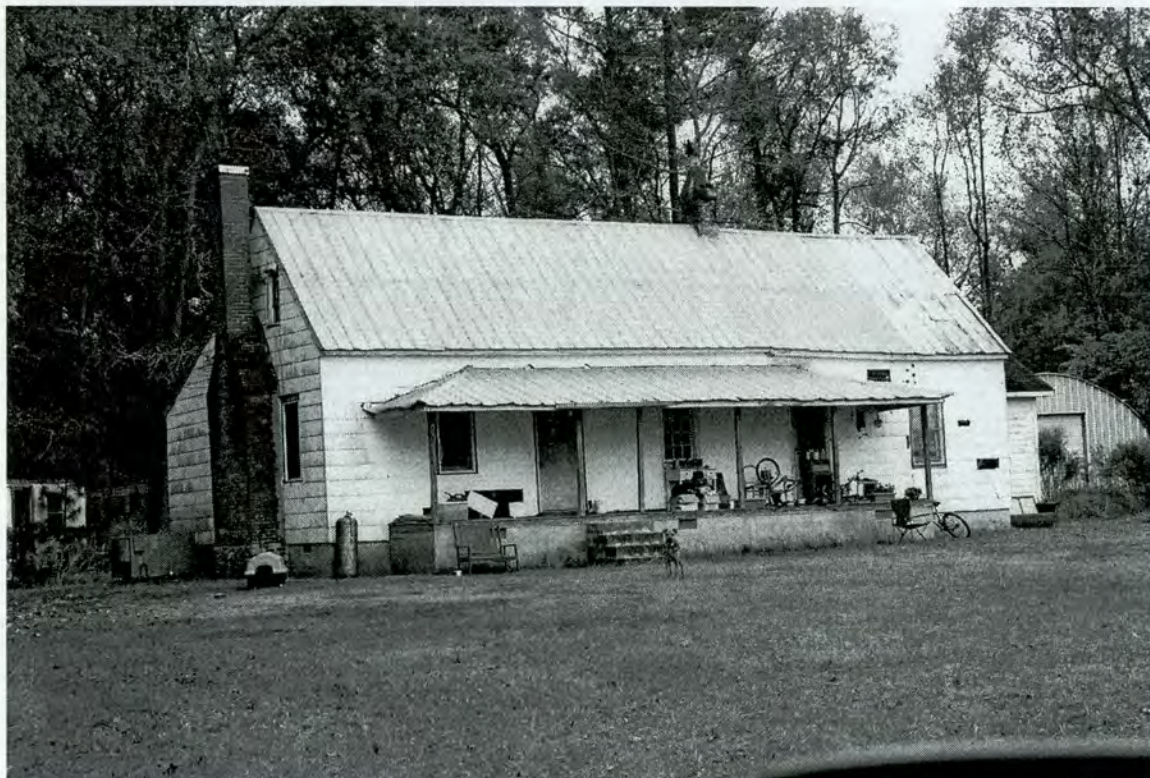
John Reddin Brown House, North and West Elevations
