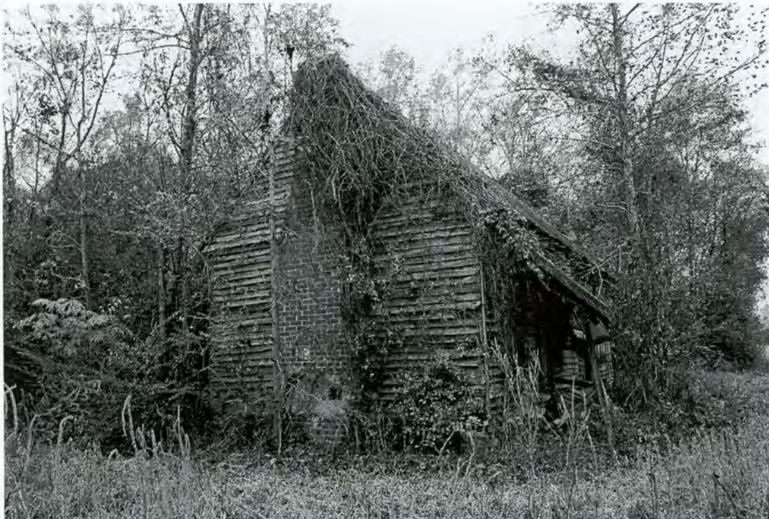
Brown House, West and South Elevations
