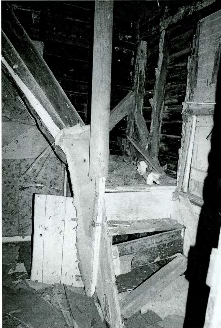
Brown House Interior, Corner Stair
