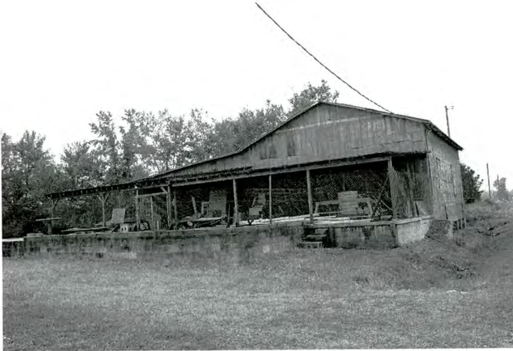
Property 24. Dupree Brothers Supply Company Building, circa 1940, west side of NC 33 just south of intersection with SR 1403, Belvoir, Pitt County
