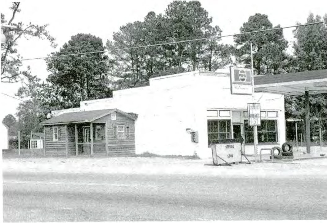
Property 26. Commercial Building, circa 1920, east side of NC 33 just north of junction with SR 1400, Belvoir, Pitt County
