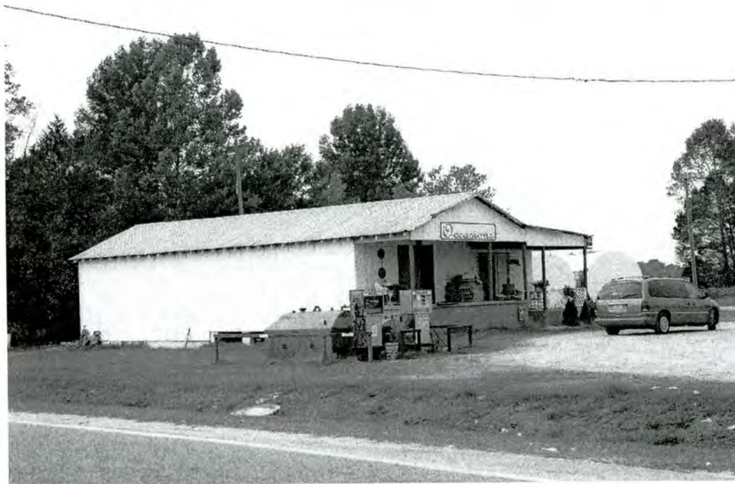
Property 25. Commercial Building, circa 1950, on triangular parcel of land in between SR 1400 and SR 1403, Belvoir, Pitt County
