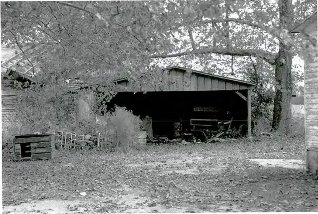
Property 11. Garage, circa 1920, 2756 NC 33, Pitt County
