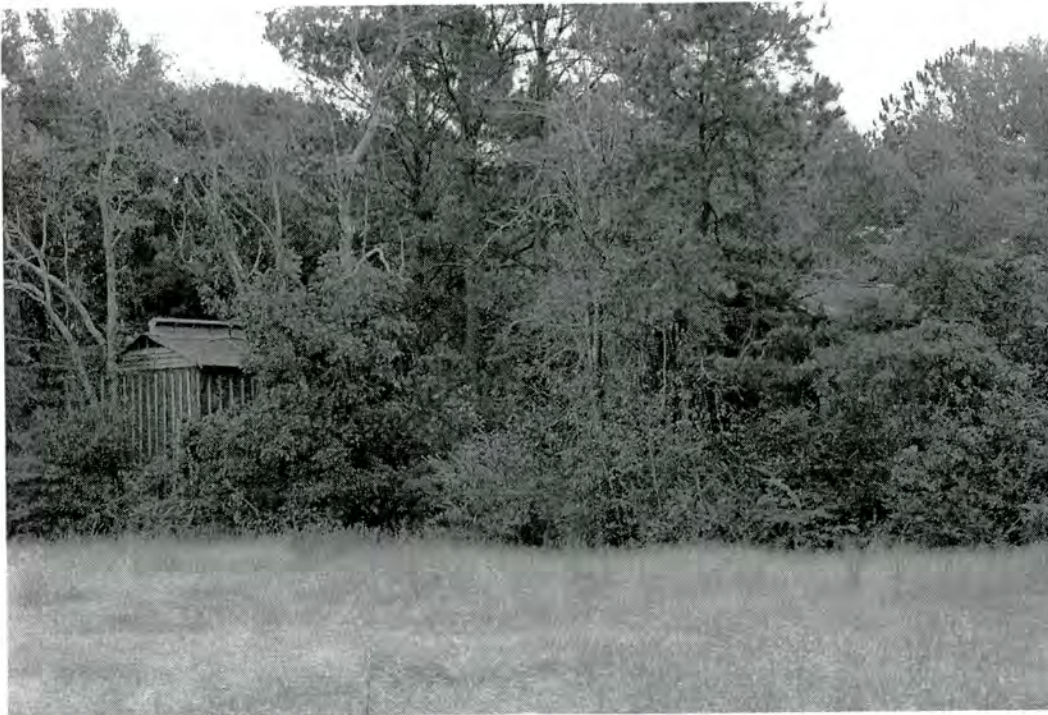
Property 9. Tobacco Barns, circa 1940, located in the woods on the east side of NC 33 just north of its intersection with US 264, Pitt County
