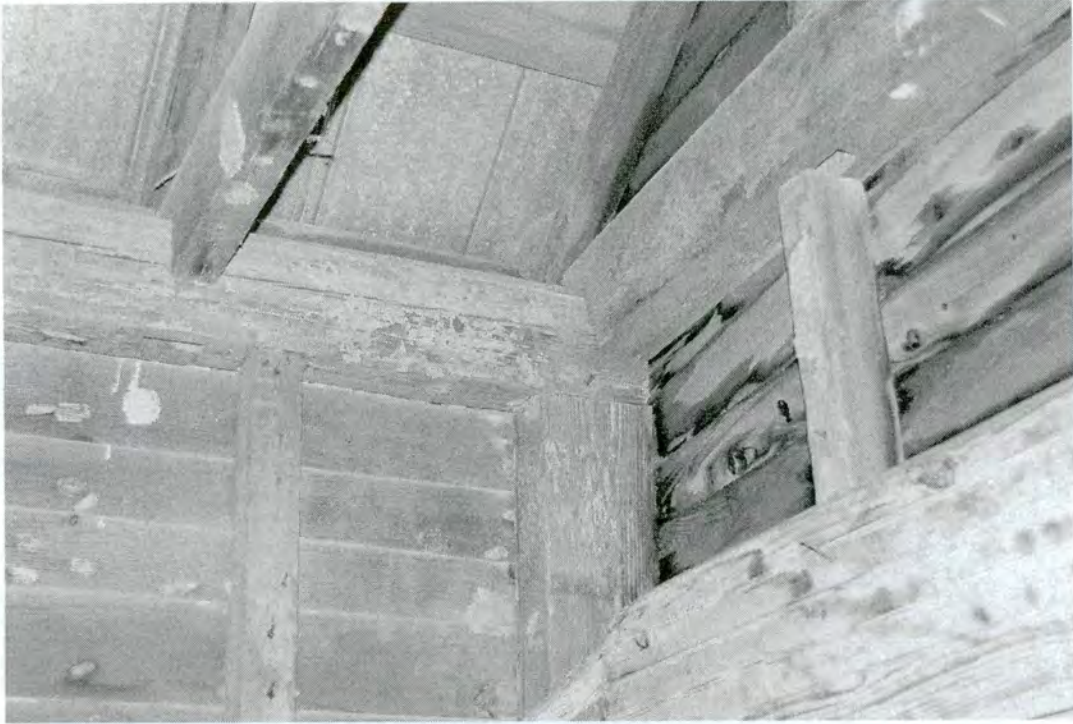
Little House Interior, Corner Framing Detail
