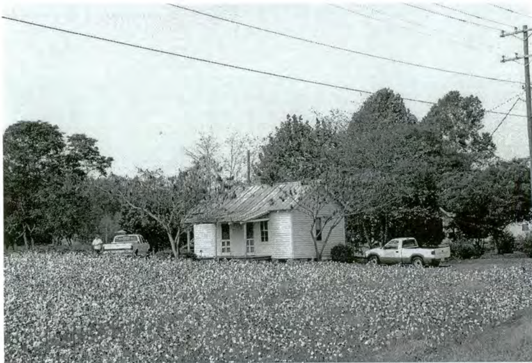
Tyson Tenant House, South and East Elevations
