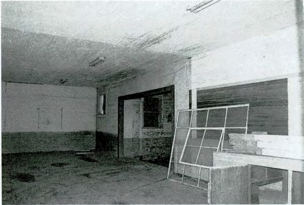
Belvoir School, 1948 Classroom Addition to Agriculture Shop Interior
