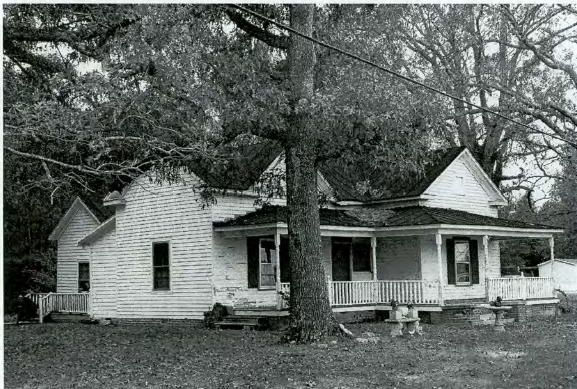
Shade and Addie Elizabeth Harris House South and East Elevations
