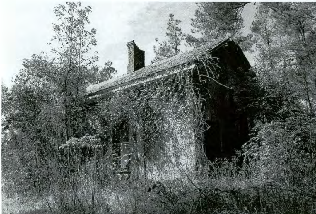
Penny Hill Doctor's Office, South and East Elevations
