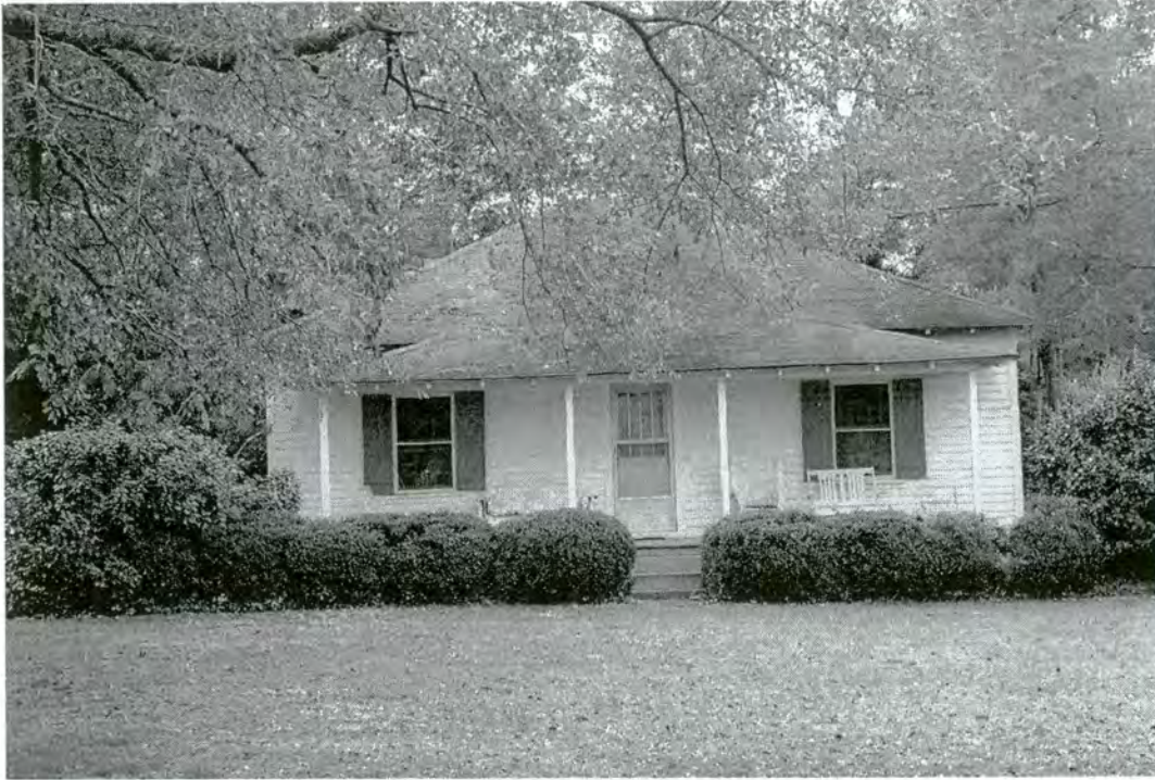
Tyson House, East Elevation
