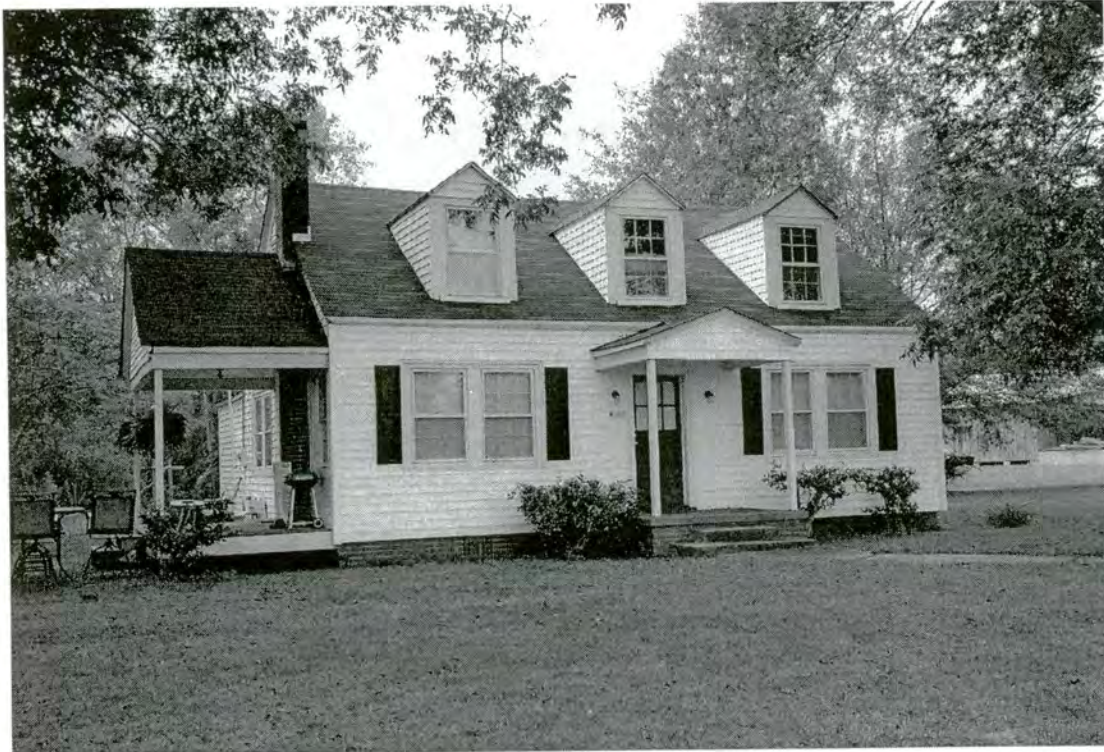
Property 22. House, circa 1940, 4110 NC 33, Belvoir, Pitt County
