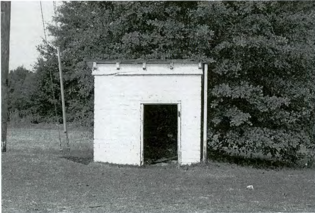
Belvoir School, Brick Shed, South Elevation
