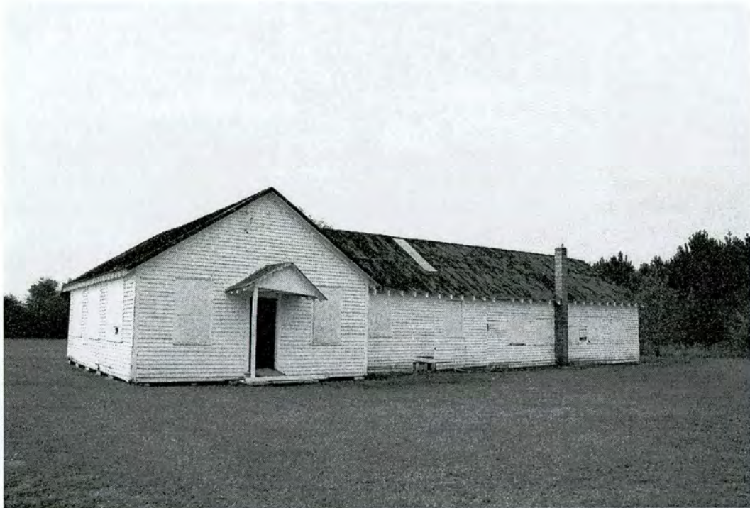
Belvoir School, 1935 Agriculture Shop with 1948 Classroom Addition, South and East Elevations
