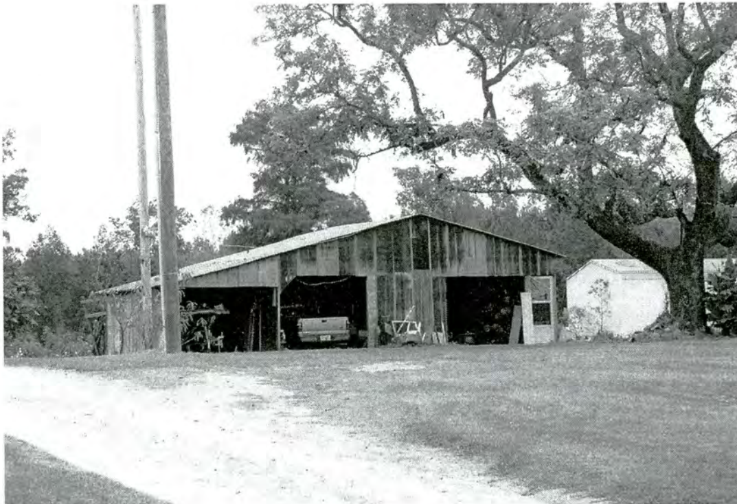
Property 18. Garage, circa 1940, 3934 NC 33, Pitt County
