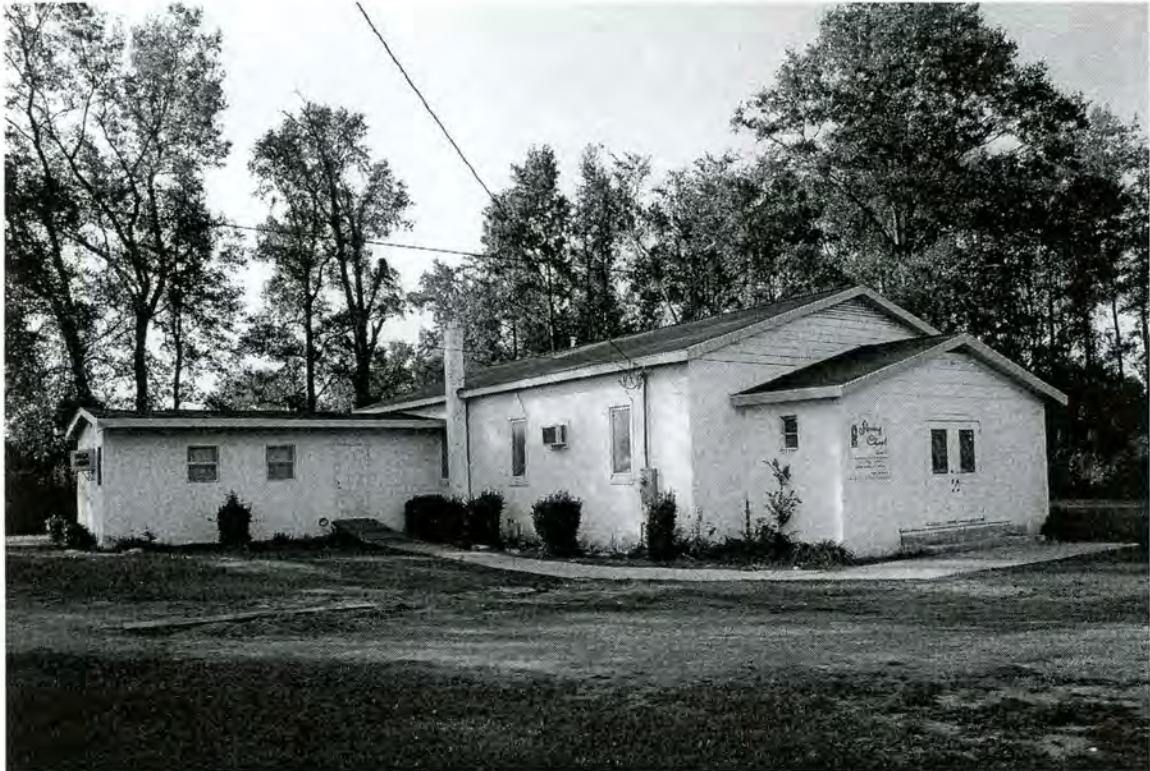
Fleming Chapel African Methodist Episcopal Zion Church East and South Elevations
