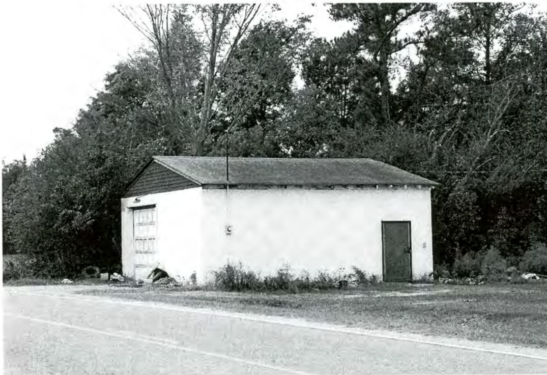
Property 25. Garage, circa 1950, on triangular parcel of land in between SR 1400 and SR 1403, Belvoir, Pitt County
