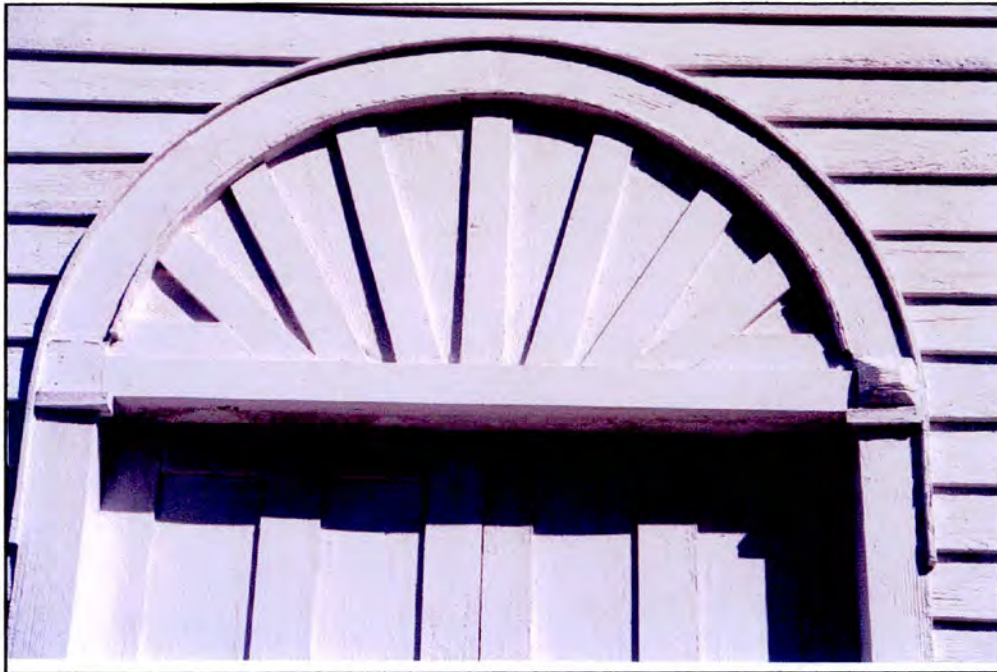
Property 5: Blind fanlight over center entrance ( Figure 12 )
