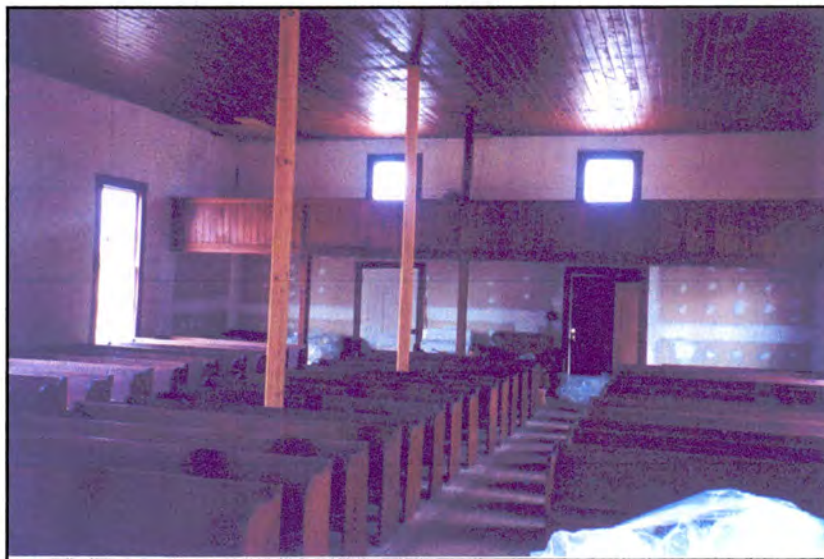
Figure 23: Spring Green Primitive Baptist Church, Hamilton vic., Martin County, N. C. This rural church was built approximately thirteen years before Singleton and its gallery, though more in keeping with antebellum fashion, is similar in finish (Photograph by Fred Harrison, Martin County Historical Society, March 2003).
