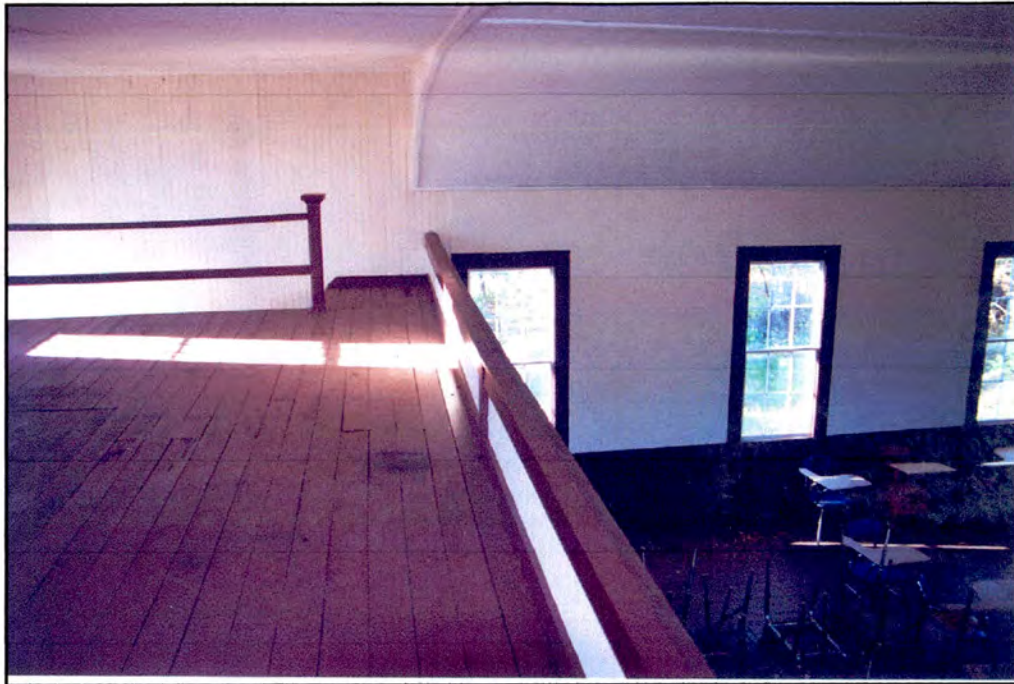
Property 5: Upper Gallery, view to west wall and stair rail/newel ( Figure 16 )
