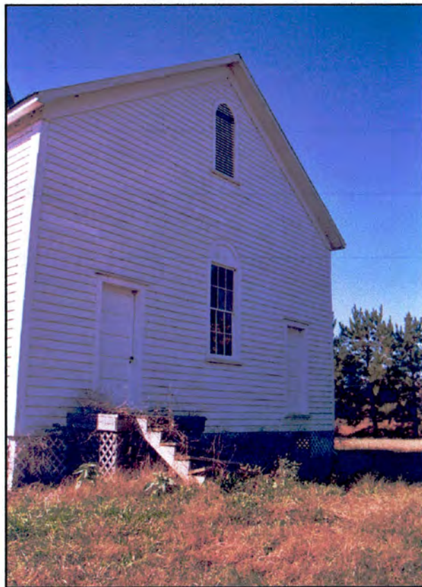
Property 5: North (rear) elevation ( Figure 9 )
