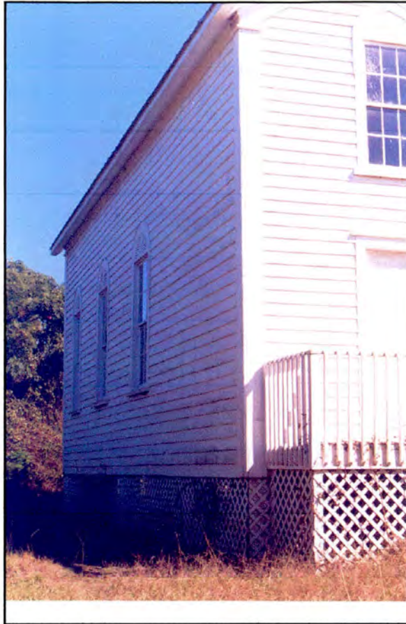
Property 5: West elevation (no ghost marks seen of an earlier window at south end) (Figure 10)
