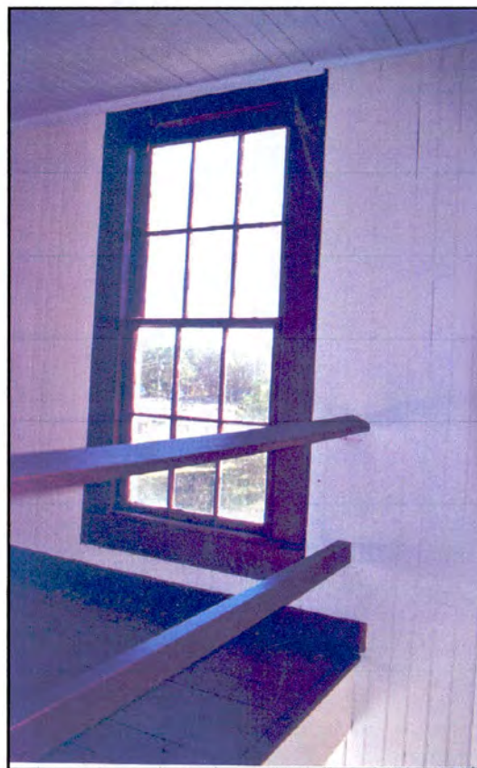
Property 5: Example of Interior Finish (sheathing, windows, flooring) ( Figure 21 )
