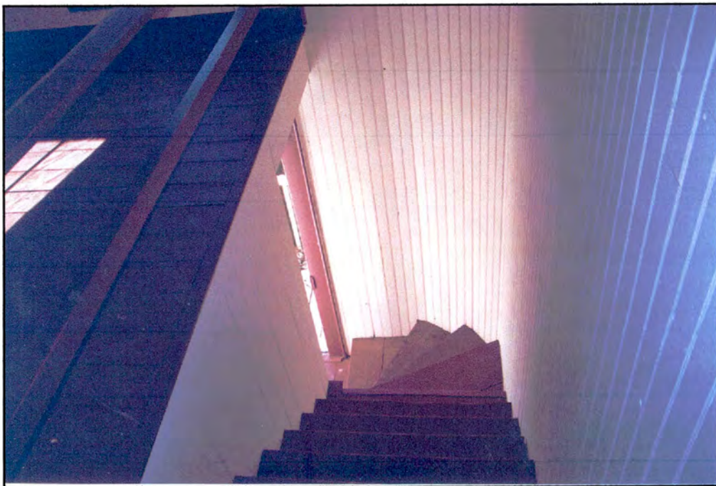
Property 5: Interior stair to gallery ( Figure 15 )
