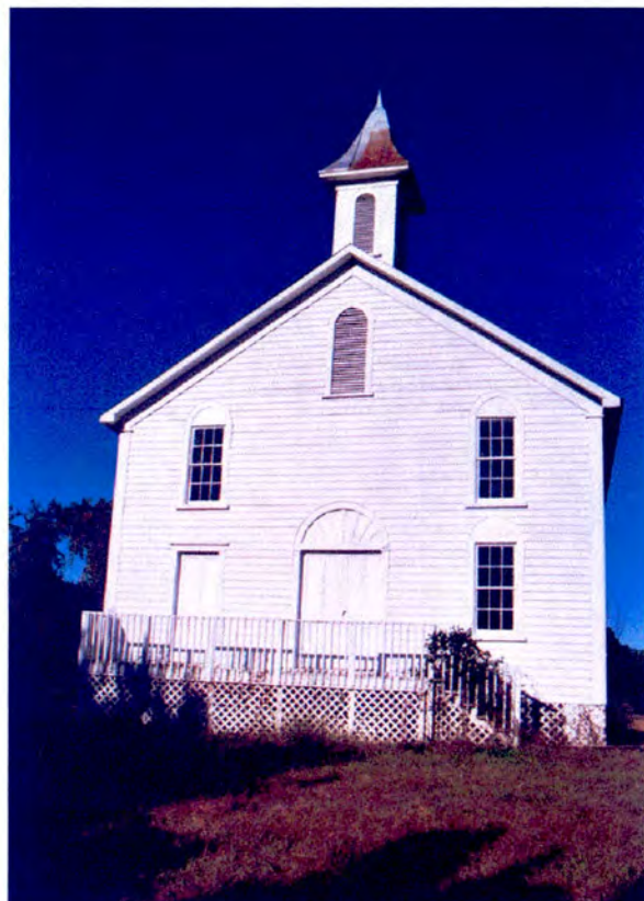
Property 5: North (entrance) elevation ( Figure 7 )
