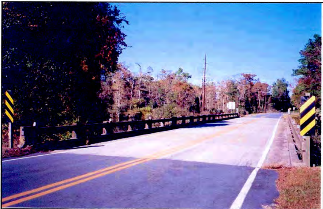
Figure 20. Bridge No. 104 looking north.
