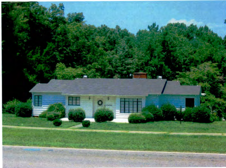
House (No. 33), Looking North.
