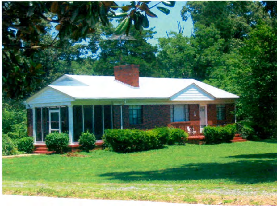
House (No. 31), Looking Northeast.
