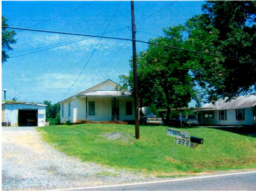
House (No. 23), Looking North.
