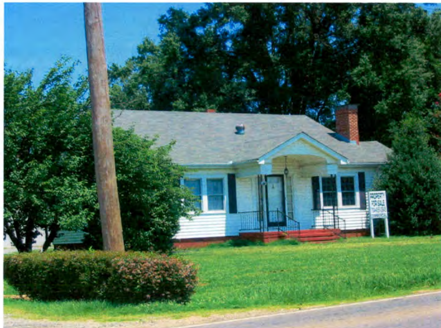
House (No. 8), Looking North.
