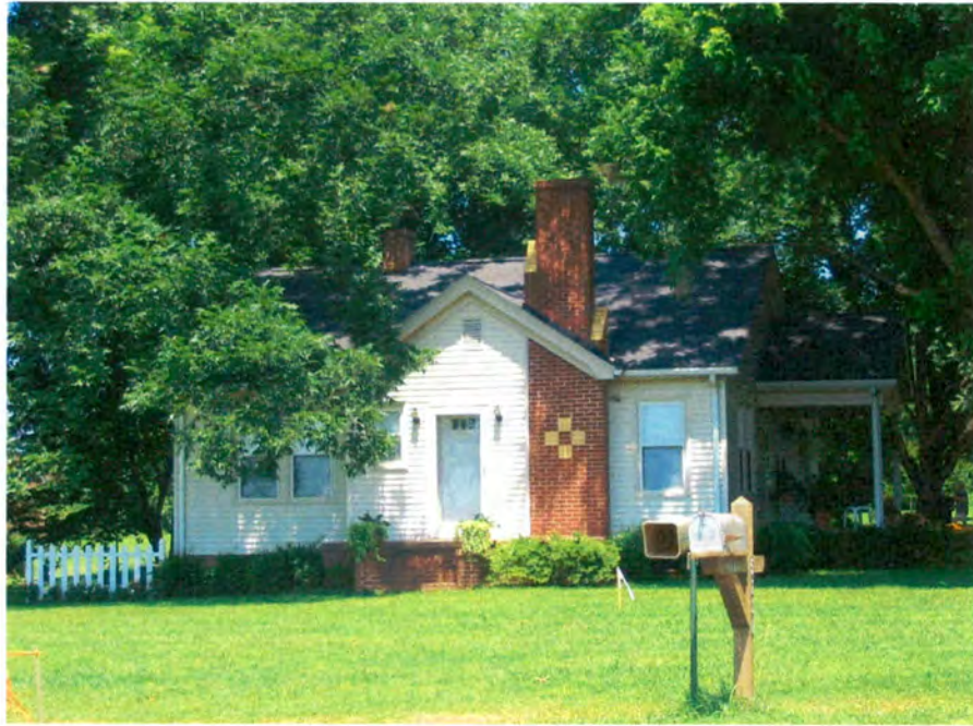
House (No. 7), Looking North.
