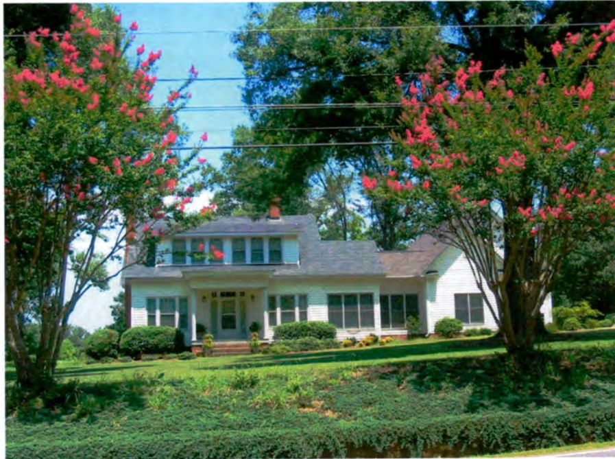
House (No. 14), Looking North.
