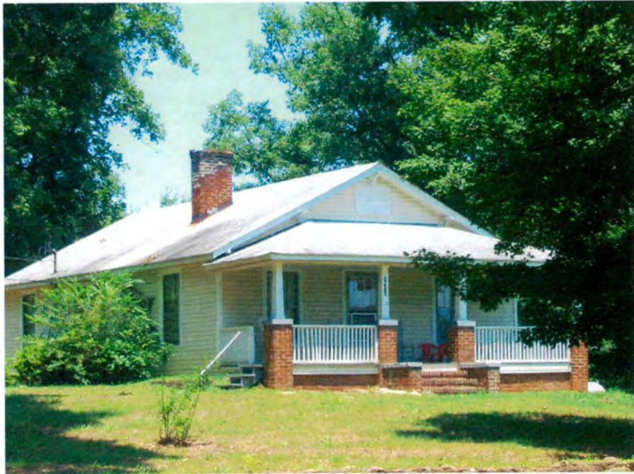
House (No. 21), Looking Northeast.
