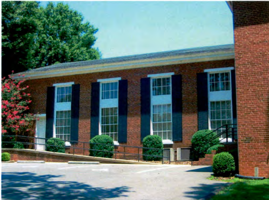
Plate 2. Poplar Tent Presbyterian Church (No. 2), Side (South) Elevation, Looking North.
