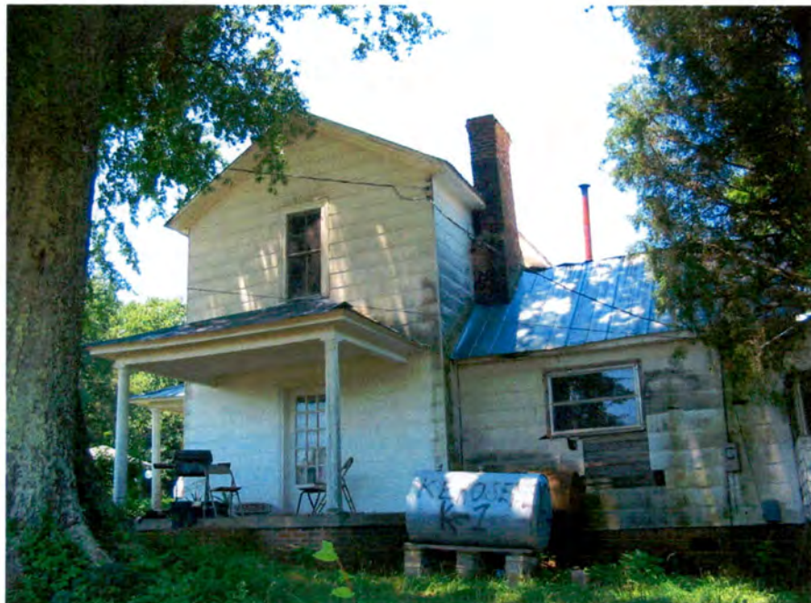
Cannon House (No. 9), Side (East) Elevation, Looking West.
