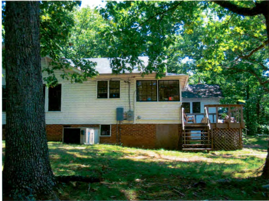
House (No. 15), Side (West) Elevation, Looking East.
