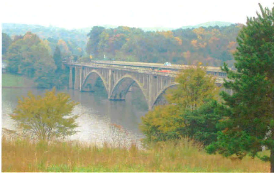
Plate 17. James B. Garrison Bridge (No. 27), View of North Profile, Looking Southeast.
