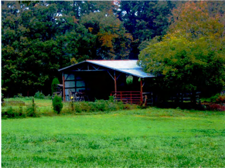
Plate 11. Dennis Barringer Farm (No. 12), Modern Equipment Shed, Looking Northwest.
