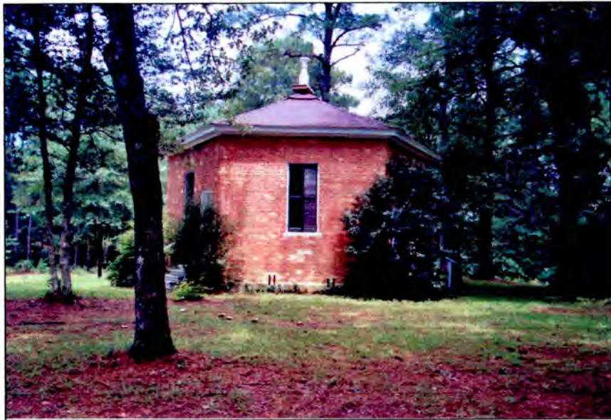
Figure 43: West elevation of Richmond Temperance and Literary Society Hall. Photograph by Penne Sandbeck/NCDOT, August 2004.
