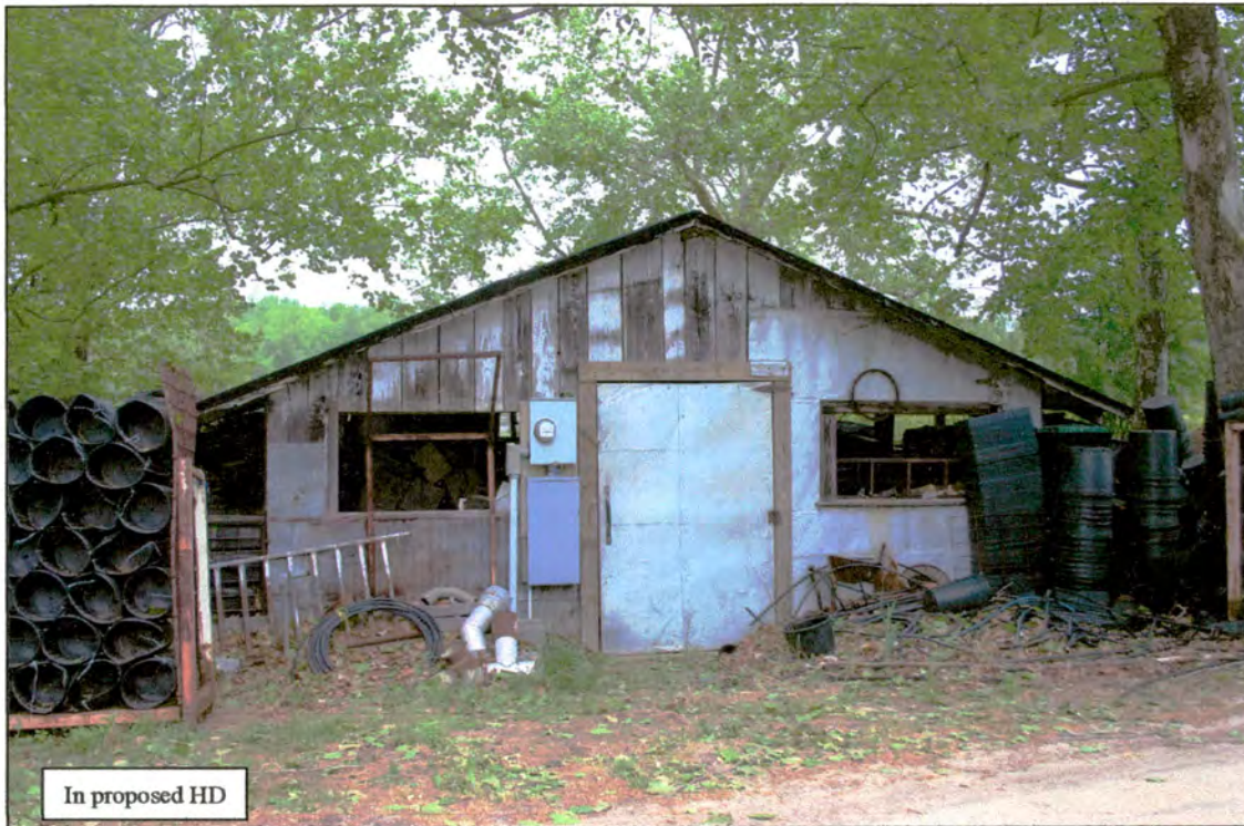
Figure 35: Property 5f: Cooley Farm, former hog house. Present owner, John C. Cooley, says his father, Jim Cooley, built this in the 1940s as a nursery for their pigs, and planted the sycamores at either side for shade.
