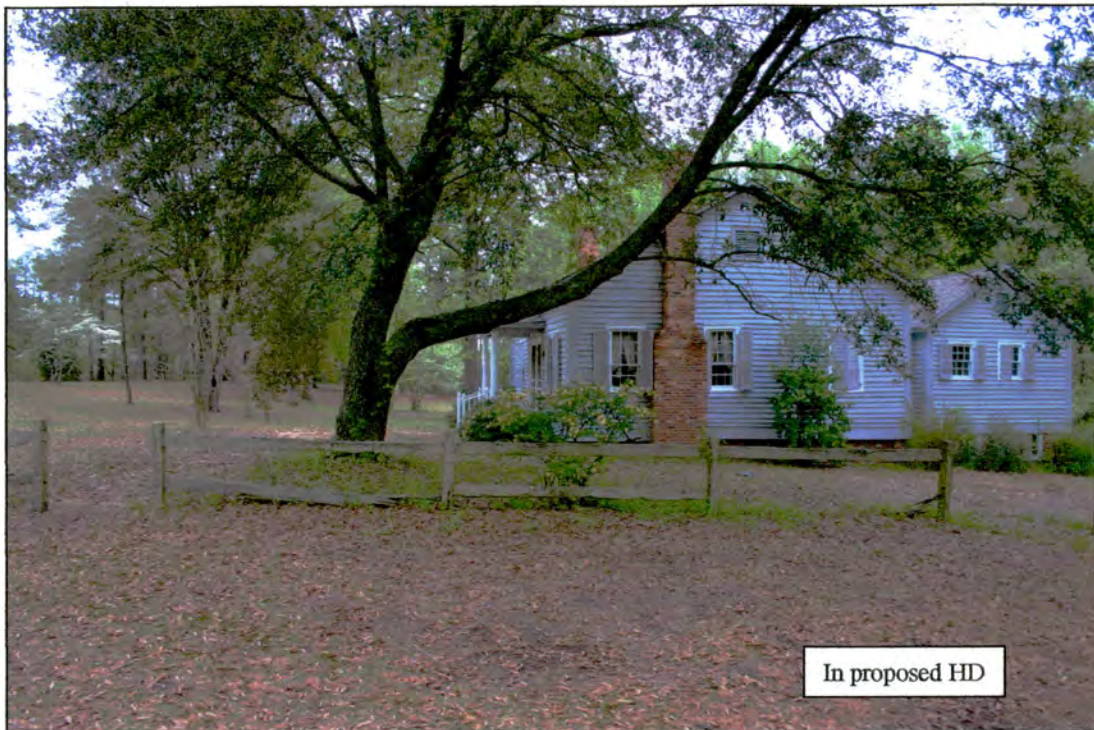
Figure 13/ Property 2: West elevation of Ellerslie
