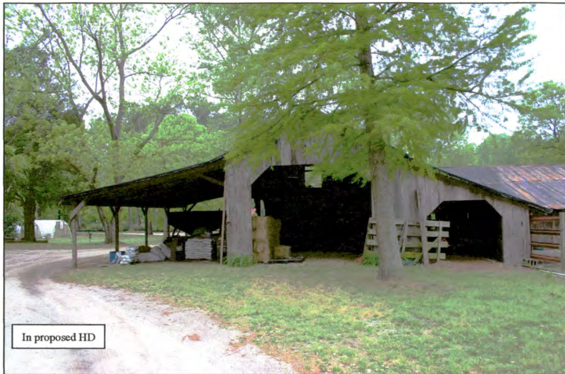
Figure 31 / Property 5c: Cooley Farm, livery stable, east elevation
