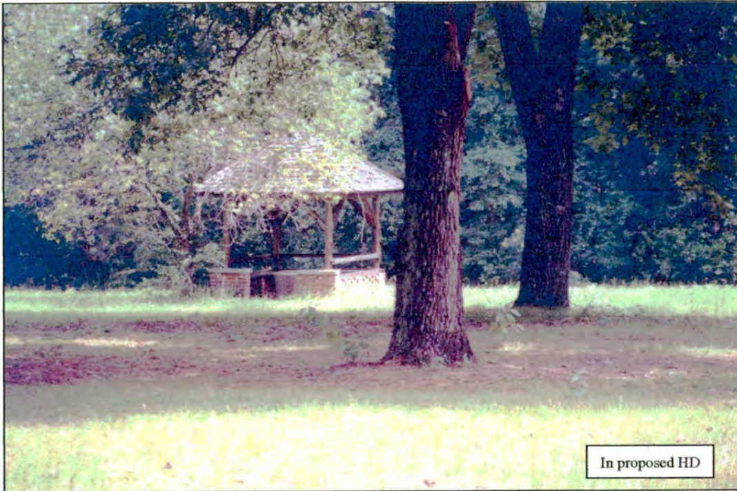
Figure 17 / Structure 4a: Spring Hill Gazebo (source of spring, constructed ca. 1966 by Wagram Garden Club), north and west elevations
