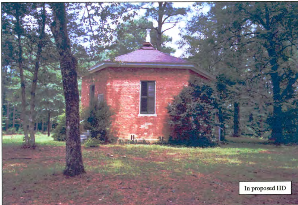
Figure 16 / Property 3: Richmond Temperance and Literary Society Hall, west, northwest, and southwest elevations
