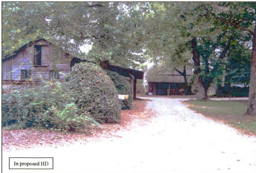
Figure 32 / Property 5c: Cooley Farm, livery stable, west elevation (smokehouse in background)
