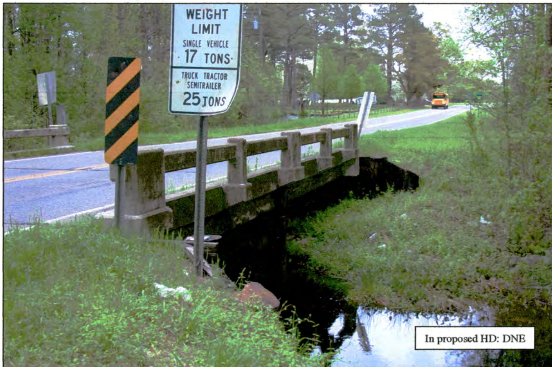
Figure 58, Property No. 4: South side of Bridge No. 14
