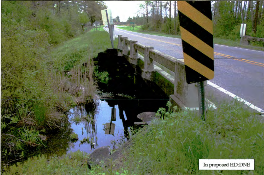
Figure 57, Property No. 4: North side of Bridge No. 14
