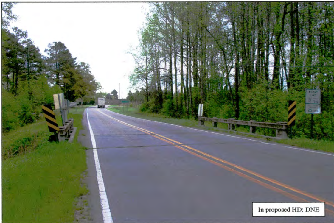
Figure 56, Property No. 4: Bridge No. 14, view from west to east
