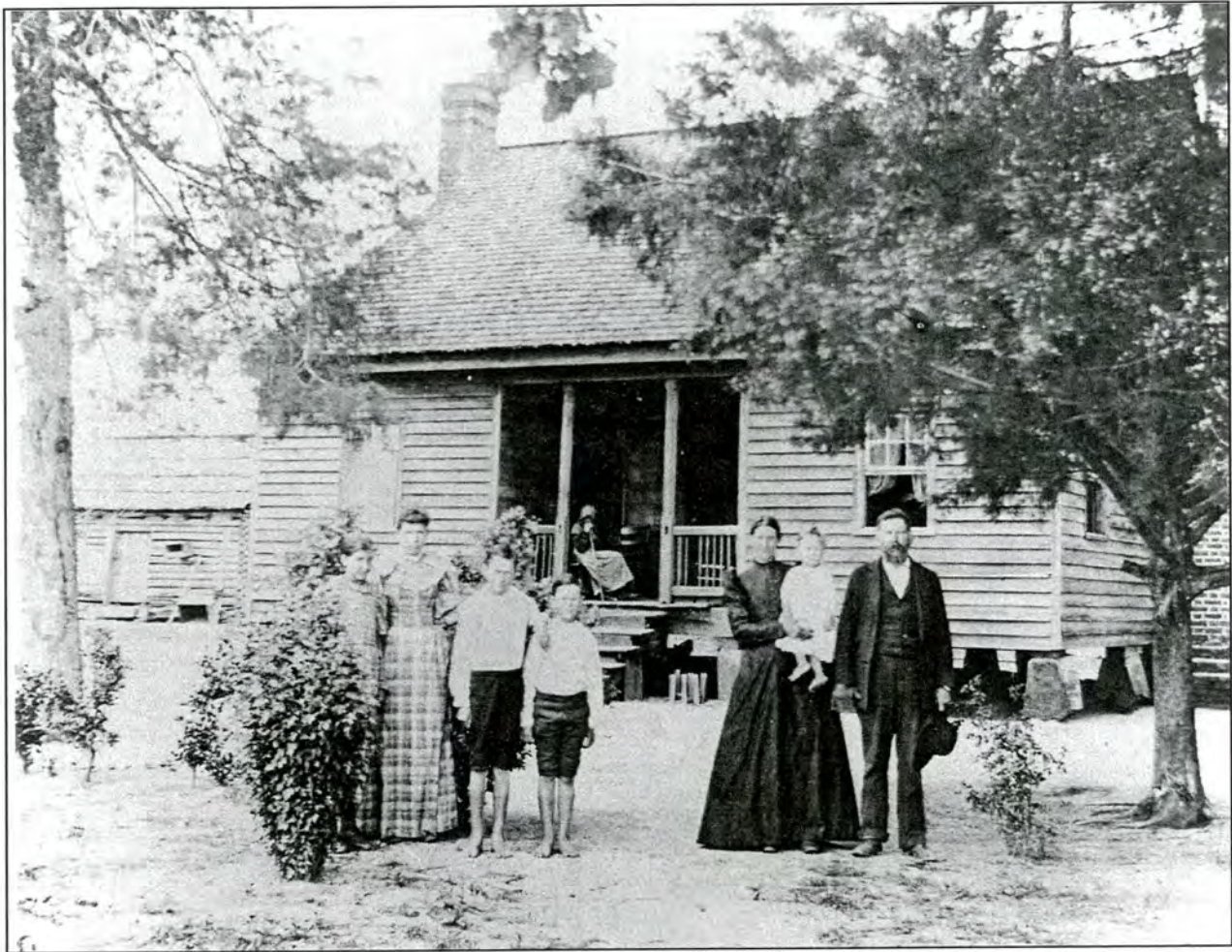
Figure 48: Archibald Leach House, Wagram vicinity, ca. 1894. The Leach House, a hall-parlor plan antebellum house with an engaged shed porch, stands in deteriorated condition north of Spring Hill. Survey and Planning Files, NC-HPO
