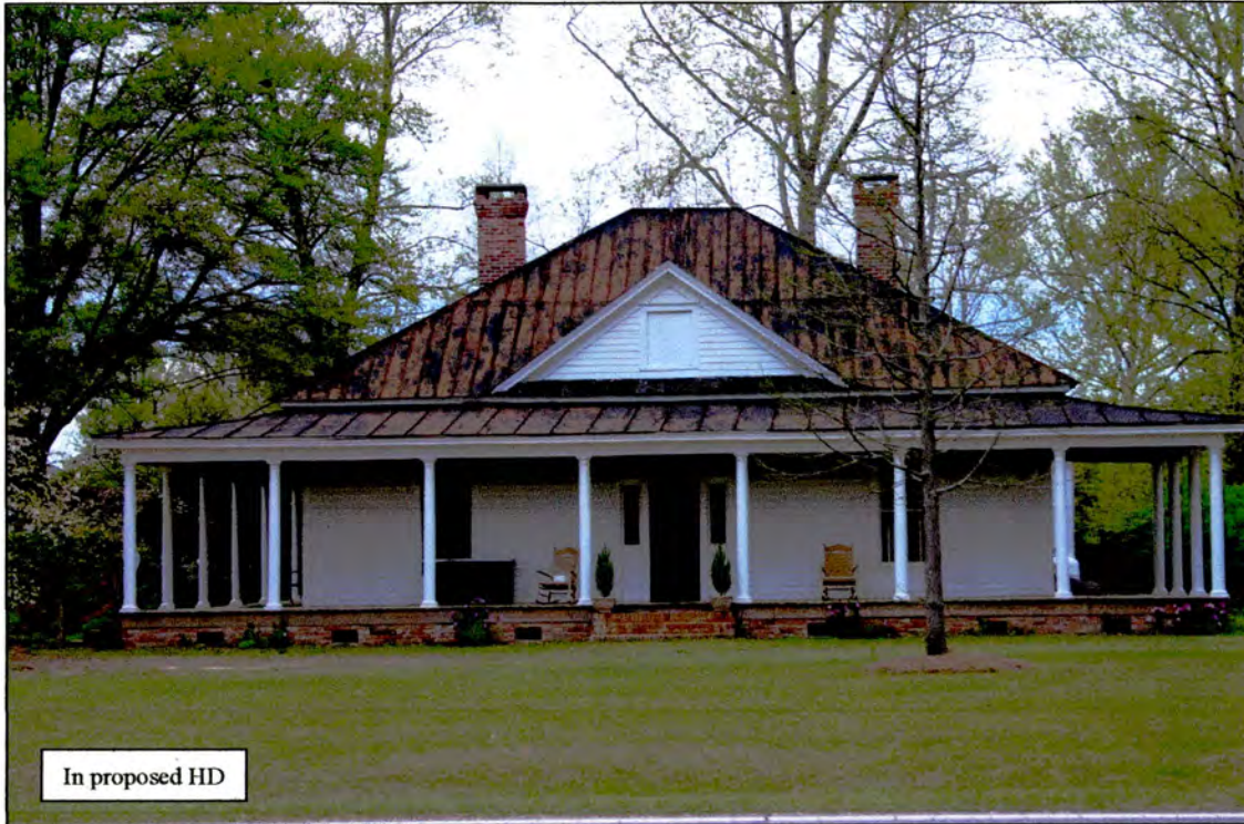
Figure 19 / Property 5: Cooley House, ca. 1880, altered 1928, front (south) elevation. House retains original weatherboard siding, ca. 1880-1928 Tuscan porch supports partly replaced with composite Tuscan posts in 2004.
