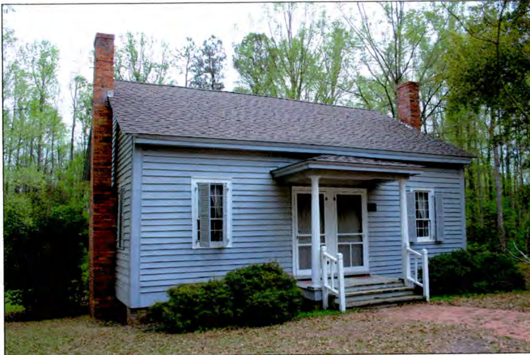
Figure 45: North (front) elevation of Ellerslie, in McNeill Memorial Park. Photograph by Penne Sandbeck, April 2005.
