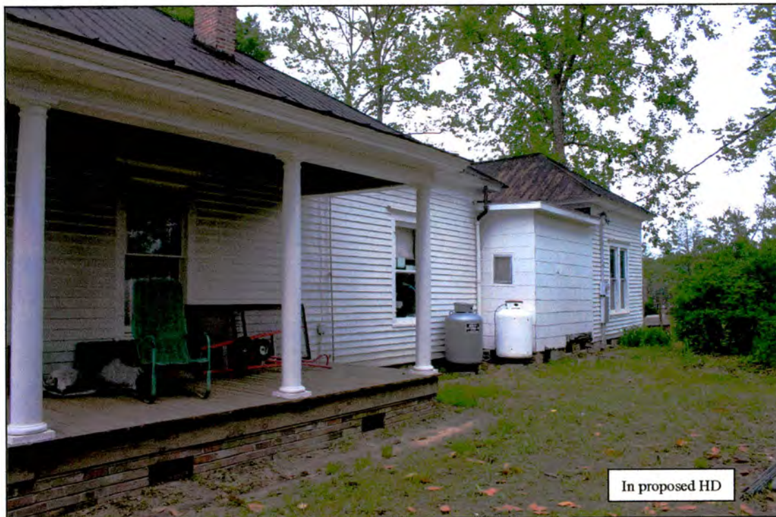
Figure 22 / Property 5: Cooley House. Detail of house's east elevation (asbestos-sided infill is the 1960s bathroom), kitchen/dining room at rear
