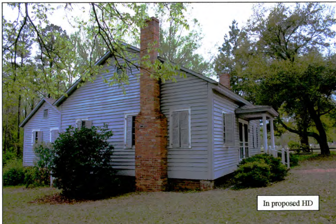
Figure 14/ Property 2: East elevation of Ellerslie
