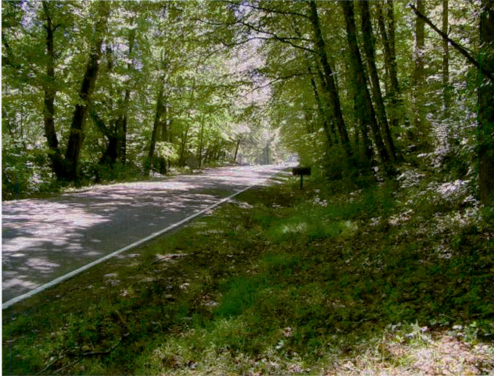
Figure 23. Newfound Gap Road, looking south from intersection with Park Circle Drive
