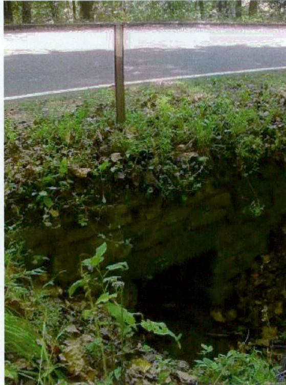
Figure 25. Pipe culvert (Sta 18+57) – west headwall, south of Park Circle Drive
