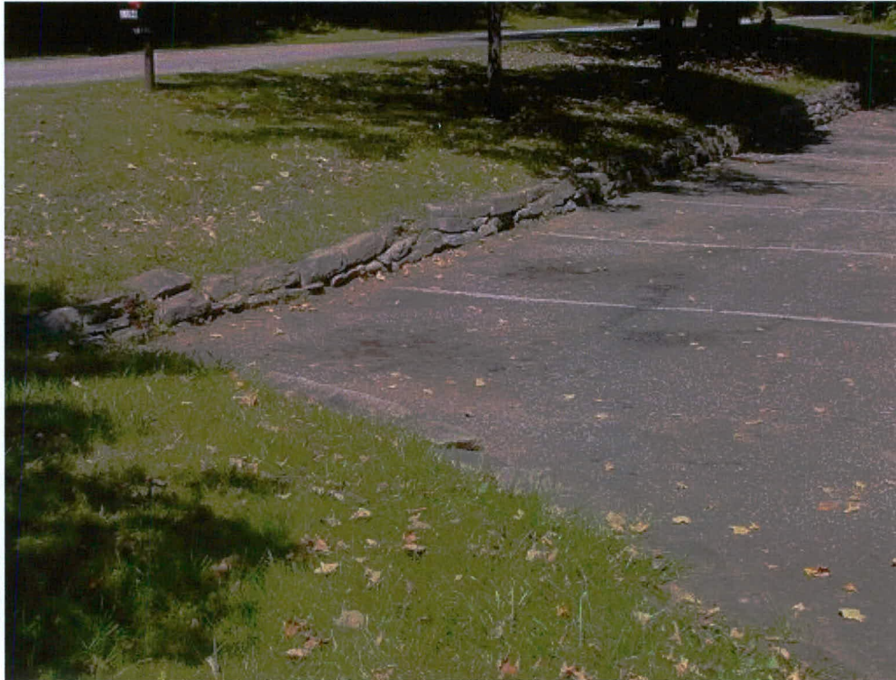
Figure 31. Detail, retaining wall, Oconaluftee Visitor Center parking area
