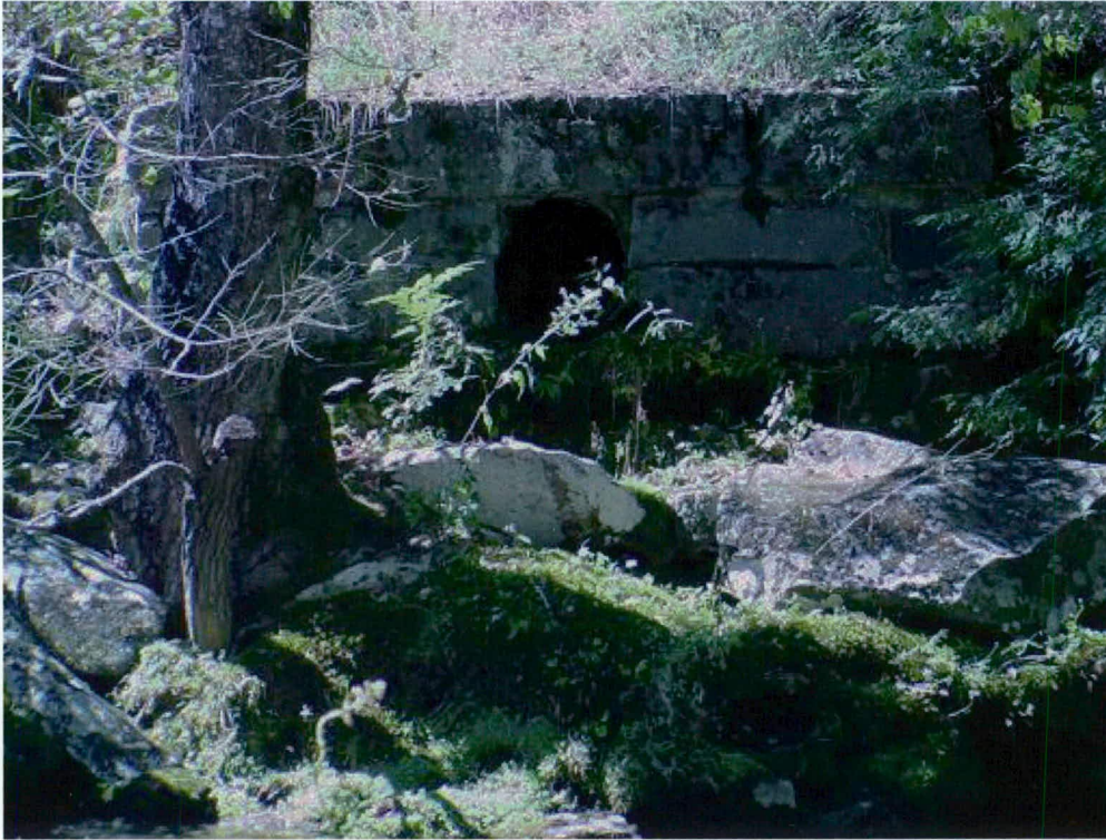
Figure 14. Pipe culvert (Sta 21+05) – east headwall, north of entrance to Smokemont Campground
