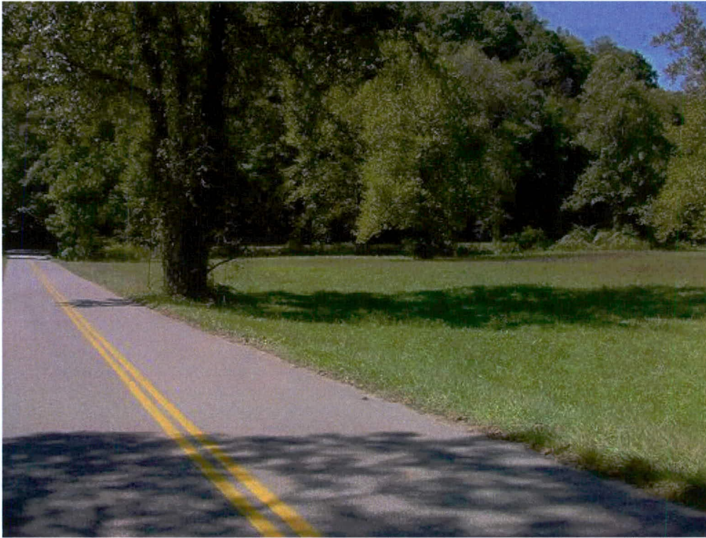
Figure 17. Tow String Road, looking west to Newfound Gap Road along the existing section and area of realignment
