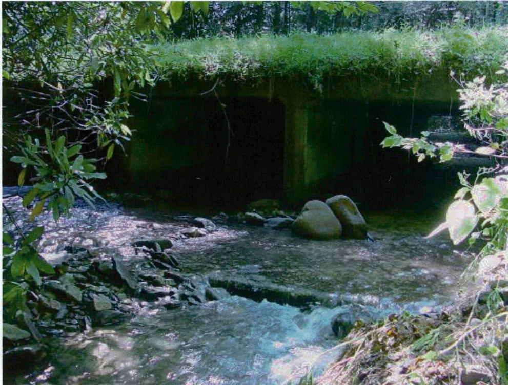
Figure 6. Collins Creek culvert, east side
