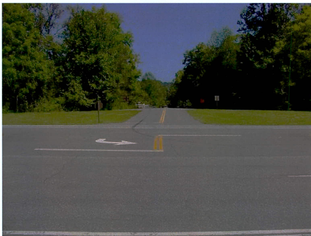
Figure 37. Blue Ridge Parkway at Newfound Gap Road, looking east across median turn lanes to the Parkway.
