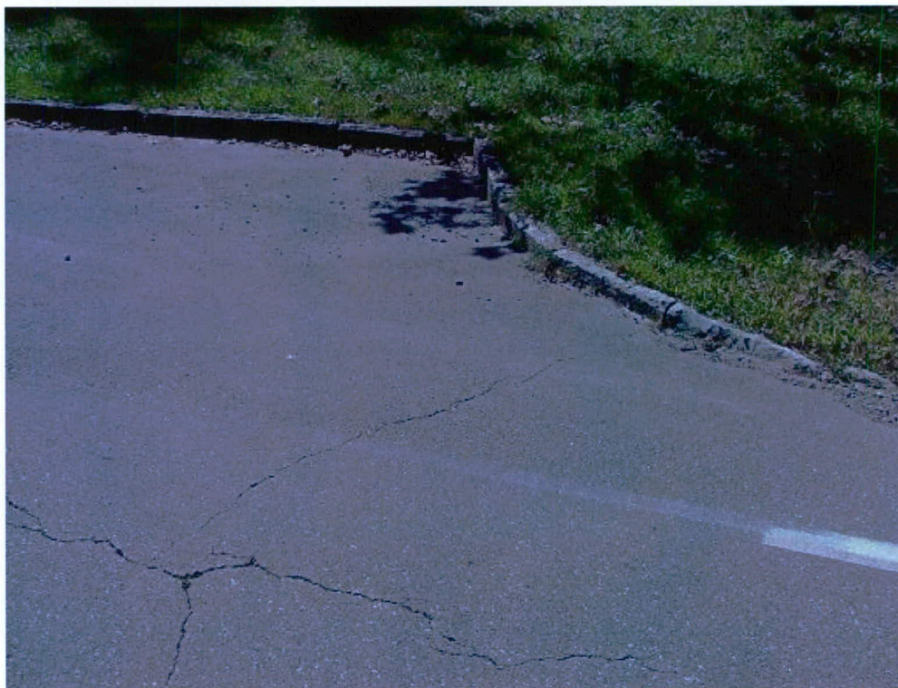
Figure 12. Detail, stone curbing in automobile pull-out, west side of Newfound Gap Road at entrance to Smokemont Campground
