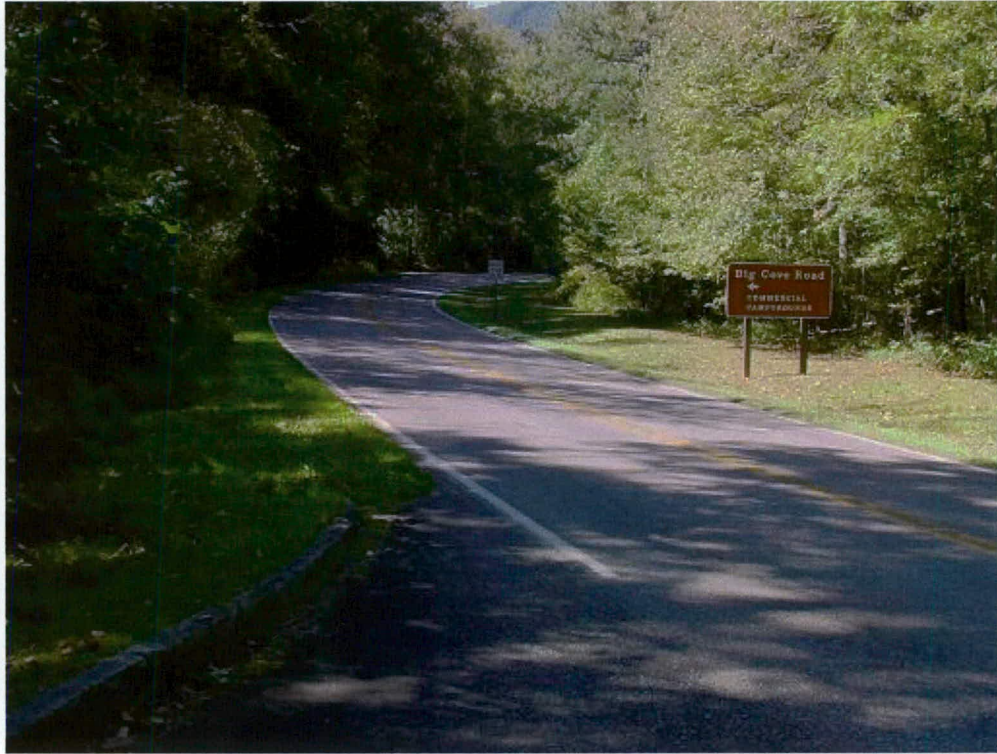
Figure 39. Newfound Gap Road, looking west to Big Cove Connector Road intersection from automobile pull-out
