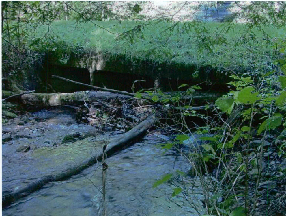
Figure 7. Collins Creek culvert, west side
