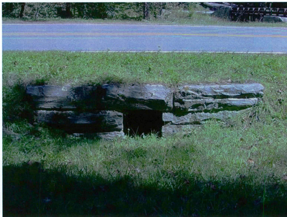
Figure 13. Pipe culvert (Sta 21+05) – west headwall, north of entrance to Smokemont Campground
