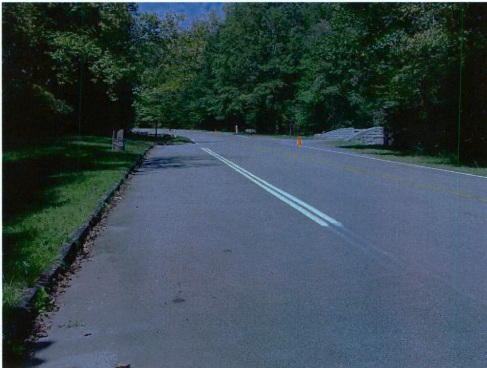
Figure 11. Automobile pull-out, west side Newfound Gap Road, looking north to entrance to Smokemont Campground
