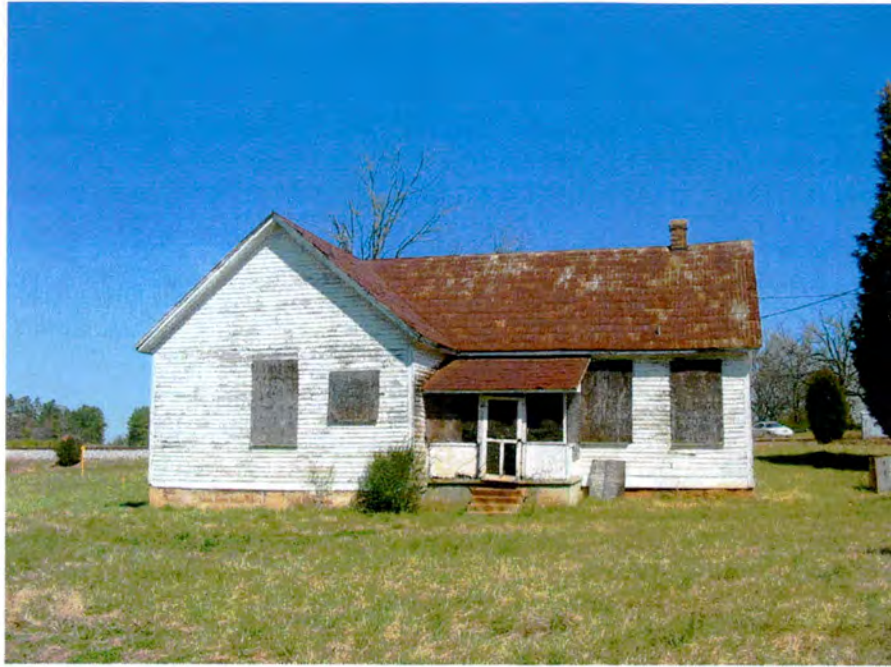
Plate 1. Bethesda School, Main (West) Elevation, Looking East.
