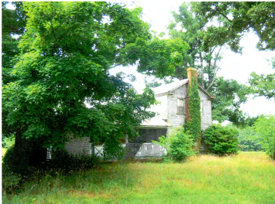
Plate 4. Cashion-Moore House, Side (North) Elevation, Looking Southwest.
