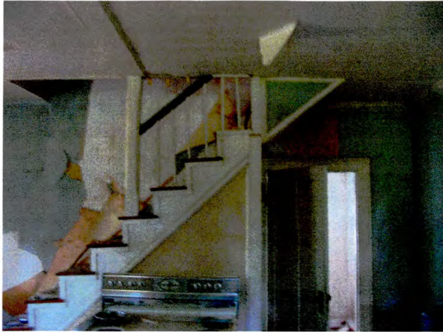
Plate 9. Cashion-Moore House, Interior, Staircase and Door Detail.
