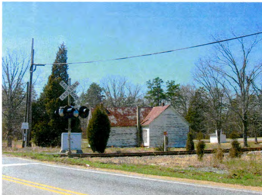
Plate 2. Bethesda School, Rear (East) Elevation, Looking Northwest Across Eastfield Road.
