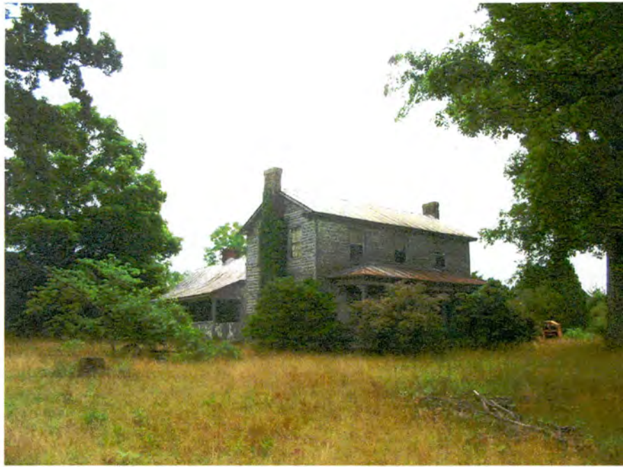
Plate 3. Cashion-Moore House, Facade and Side (North) Elevation, Looking Southeast.
