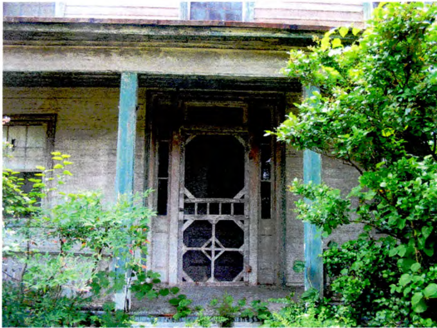
Plate 7. Cashion-Moore House, Entrance Detail.
