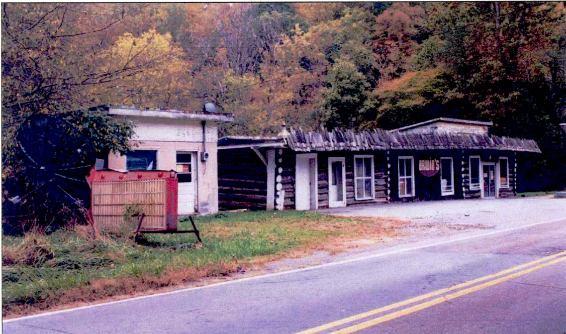
Figure 3. Northwest perspective of Erwin's building looking southeast, showing shed-roofed concrete block building at north end of original log building.
