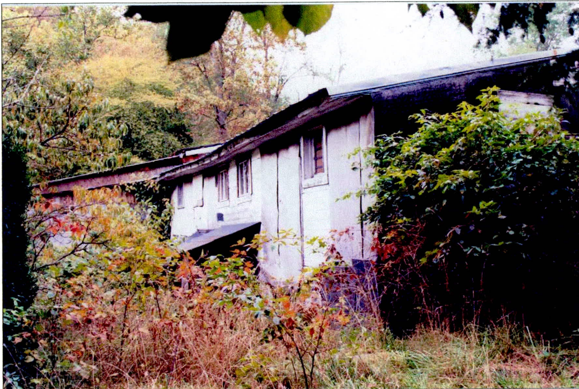
Figure 7. Northeast perspective of Erwin's building showing rear concrete block addition.
