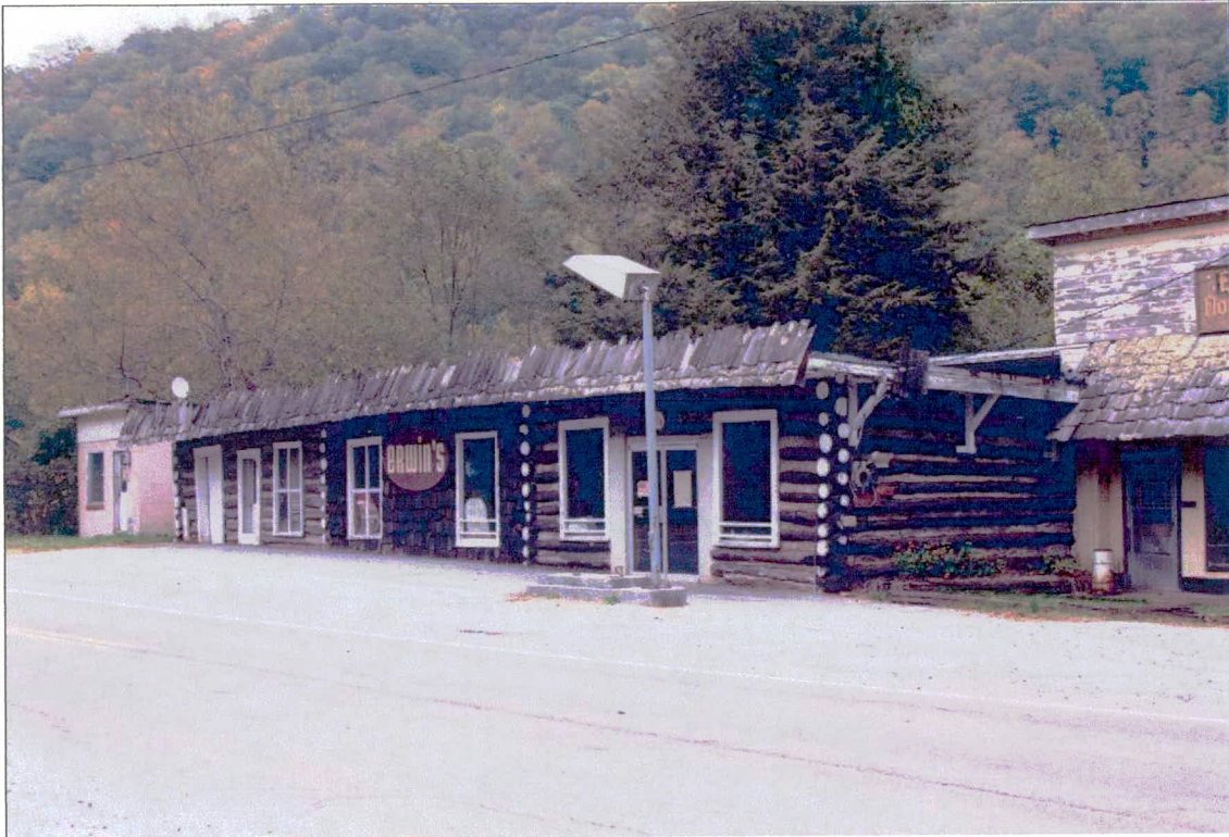
Figure 5. Southwest perspective of Erwin's building showing log section, concrete pad, and light pole.
