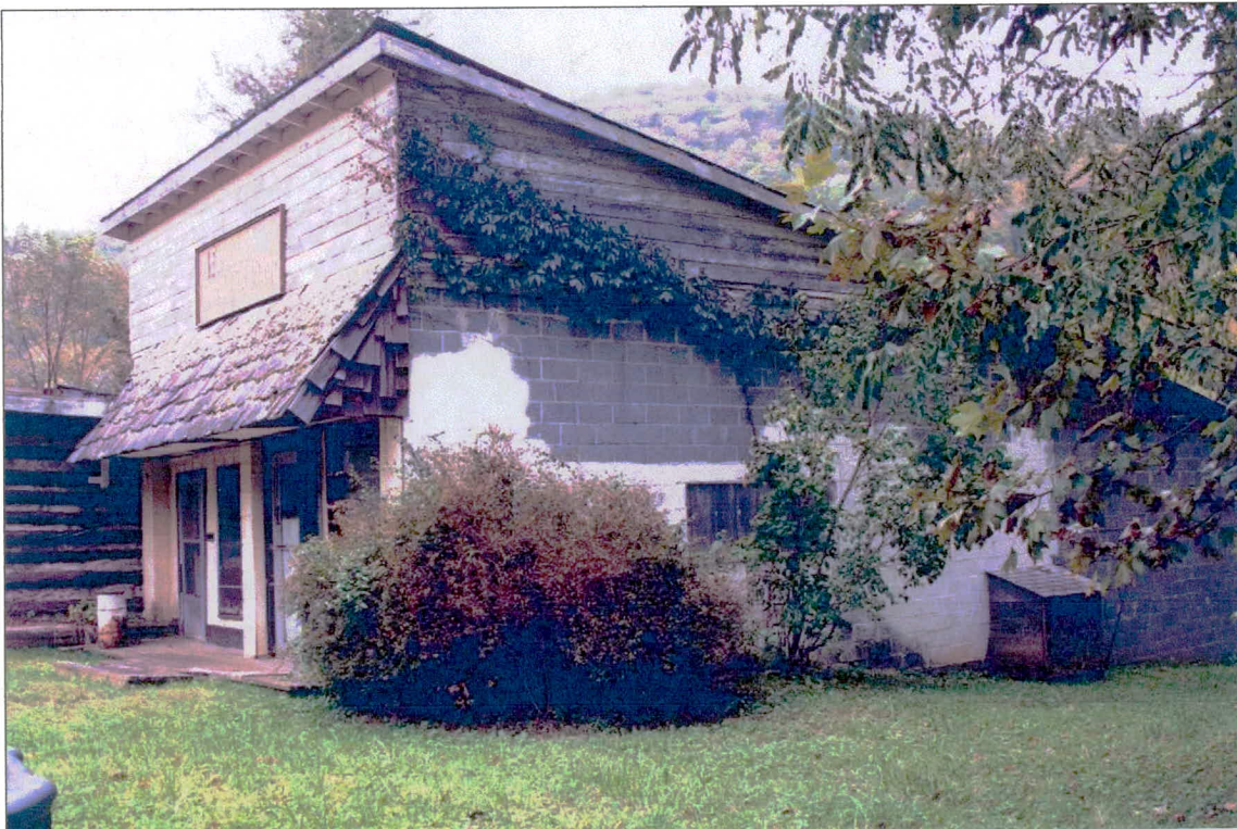
Figure 6. Southwest perspective of Erwin's building showing concrete-block section at south end of log section.
