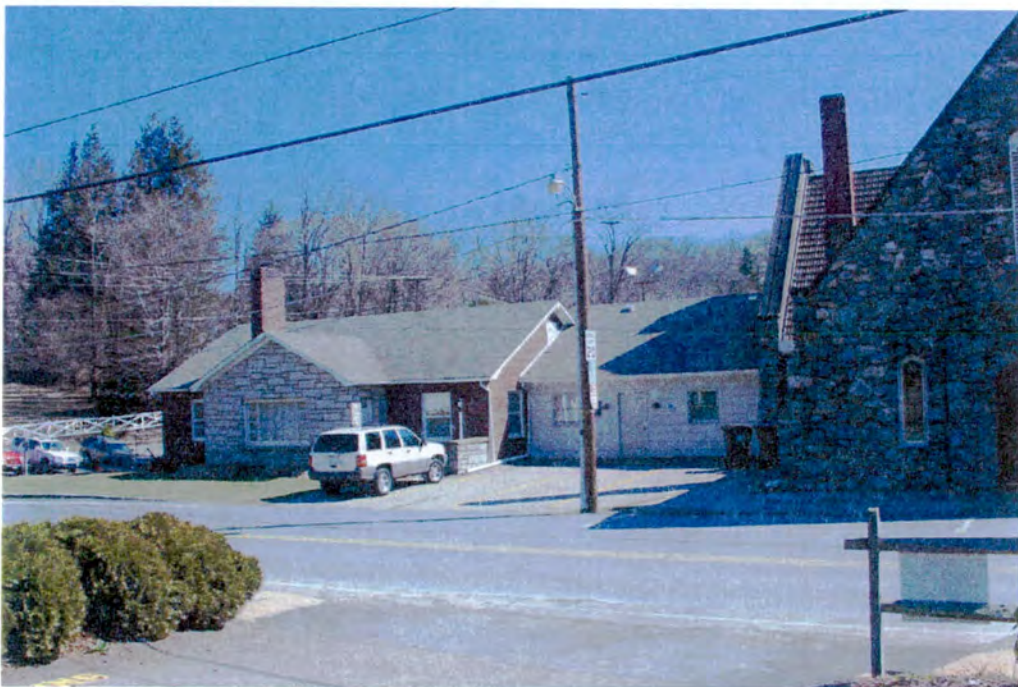
8. West elevation of Advent Christian Church showing 1980s frame hyphen connecting the church and the parsonage
