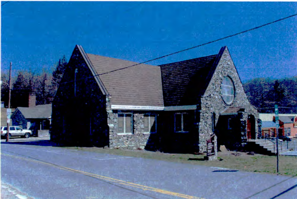
4. South front and west side elevations.
