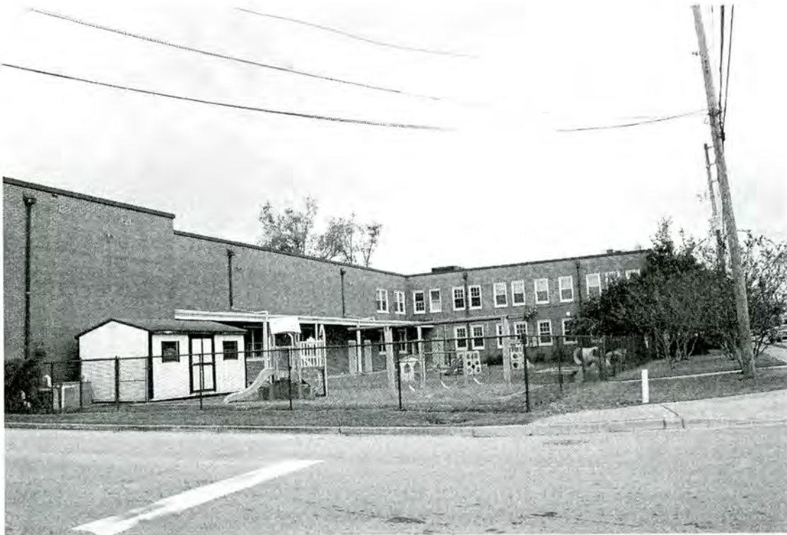
Winter Park Presbyterian Church, West and North Elevations of Additions
