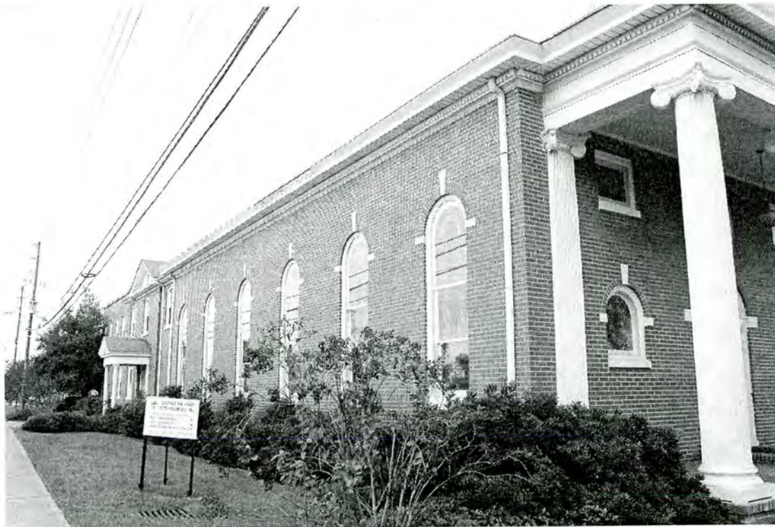
Winter Park Presbyterian Church, West Elevation
