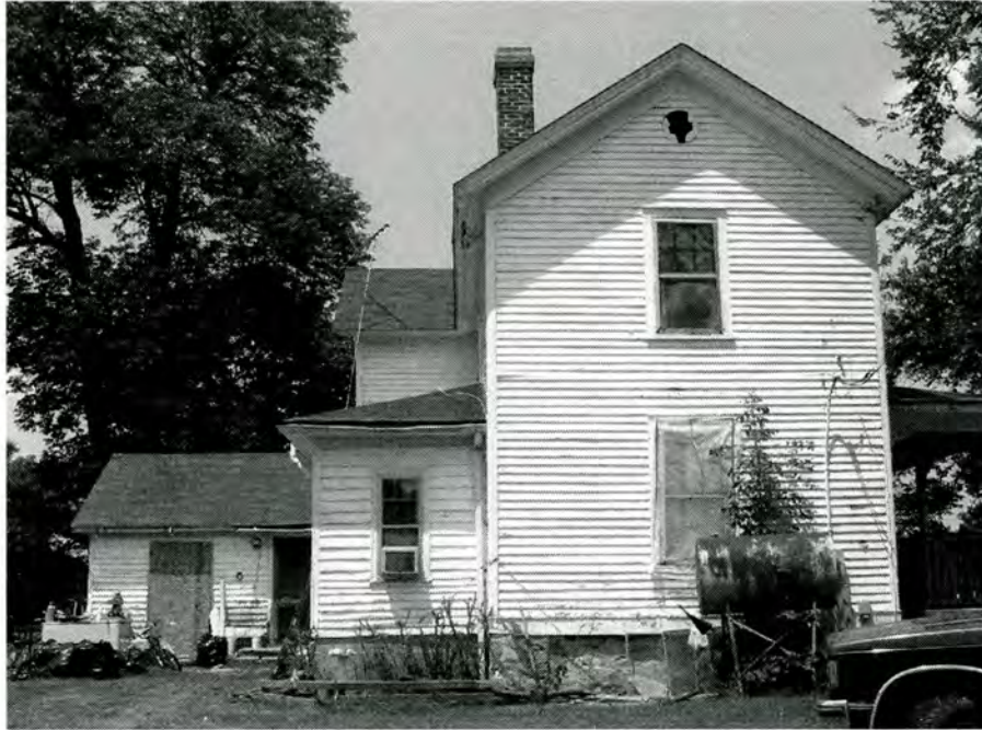
House (No. 4), Side (South) Elevation of House, Looking North.
