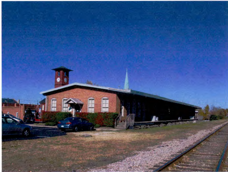
Plate 11. Seaboard Air Line Railway, Freight Station, Henderson, Vance County Looking North.
