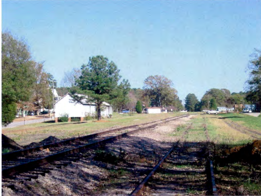
Plate 3. Railroad Bed, Norlina, Warren County, Looking North.
