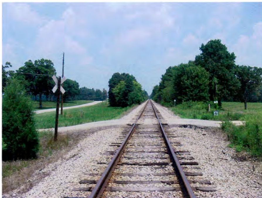
Plate 2. Railroad Bed, Crossing S.R. 1501, Middleburg, Vance County, Looking North.
