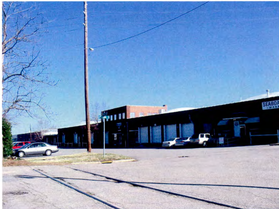
Plate 6. Seaboard Air Line Railway Station and Warehouses, Warehouses, Raleigh, Wake County, Looking North.
