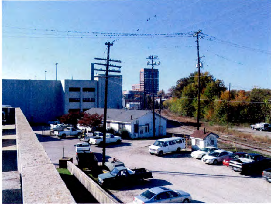
Plate 15. Seaboard Air Line Shops Building, Raleigh, Wake County, Looking Southwest.
