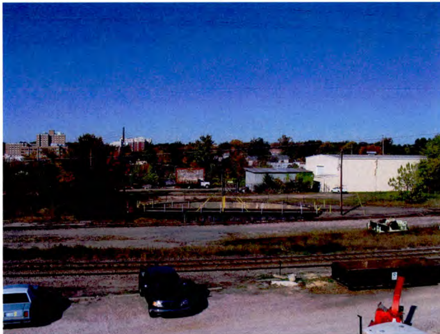
Plate 14. Raleigh and Gaston Railroad Turntable, Raleigh, Wake County, Looking West.
