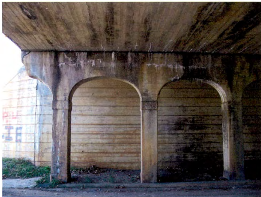
Plate 26. Seaboard Air Line Railway Bridge over U.S. 158, Substructure, Norlina, Warren County.
