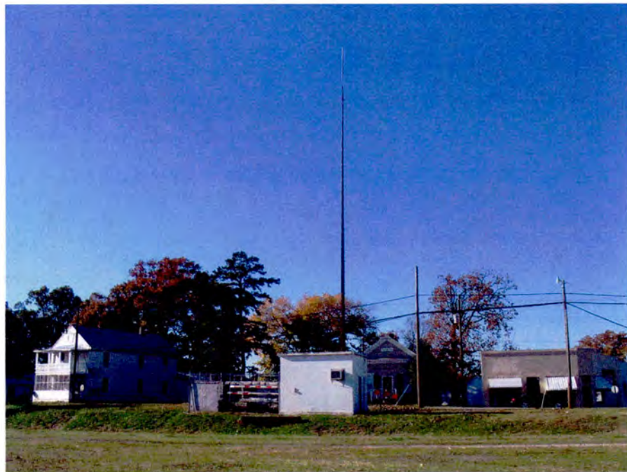
Plate 28. Seaboard Air Line Railway, Repeater Tower, Norlina, Warren County, Looking West.
