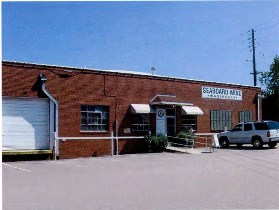
Plate 7. Seaboard Air Line Railway Station and Warehouses, Warehouse, Raleigh, Wake County, Looking East.
