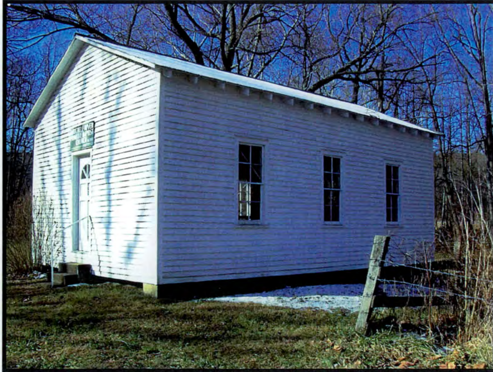
Figure 6: Mitchell River Primitive Baptist Church. Side/northeast elevation.
