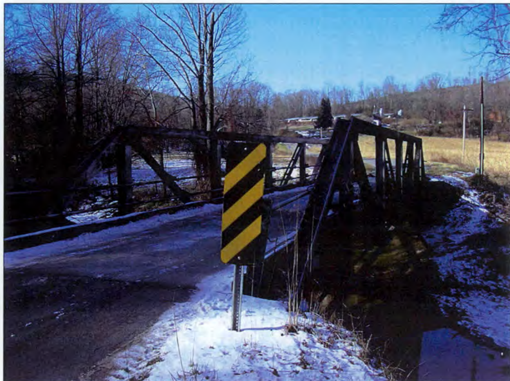
Figure 1: Bridge No. 37. View looking west on SR 1330 (Haystack Road).
