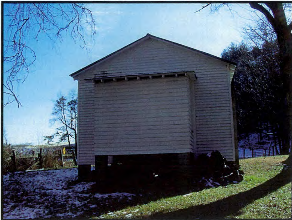
Figure 7: Mitchell River Primitive Baptist Church. Rear/northwest elevation.
