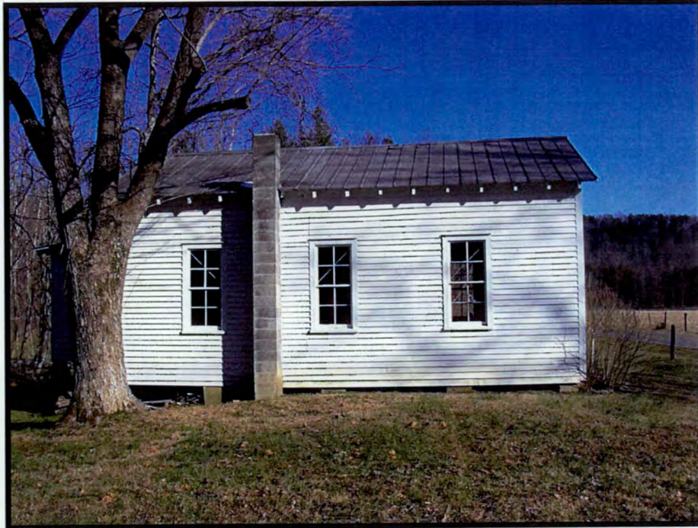
Figure 8: Mitchell River Primitive Baptist Church. Side/southwest elevation.
