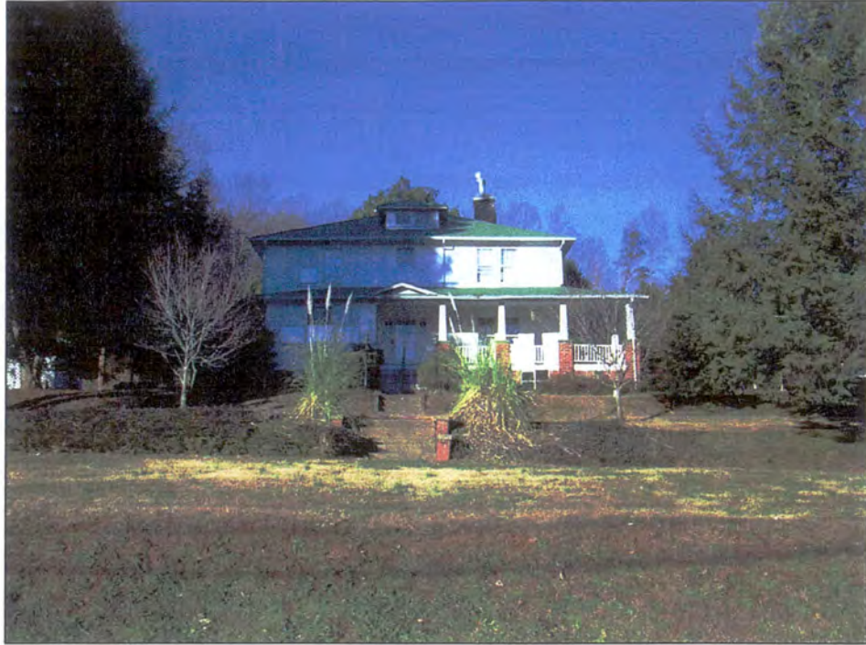
Figure 10: Stacy House, front (south) elevation.
