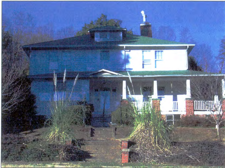
Figure 11: Stacy House, front (south) elevation.
