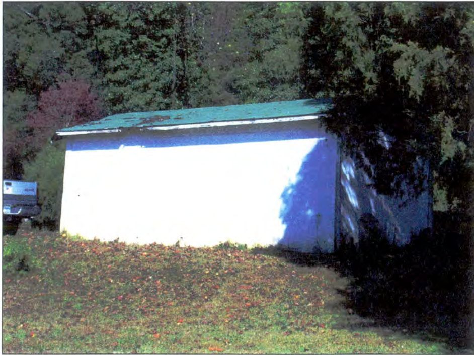
Figure 14: Stacy House, concrete block garage east of house.
