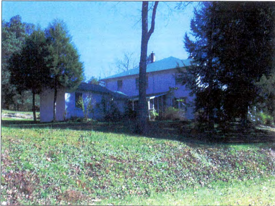
Figure 13: Stacy House, side (west) elevation with shed at left of frame.
