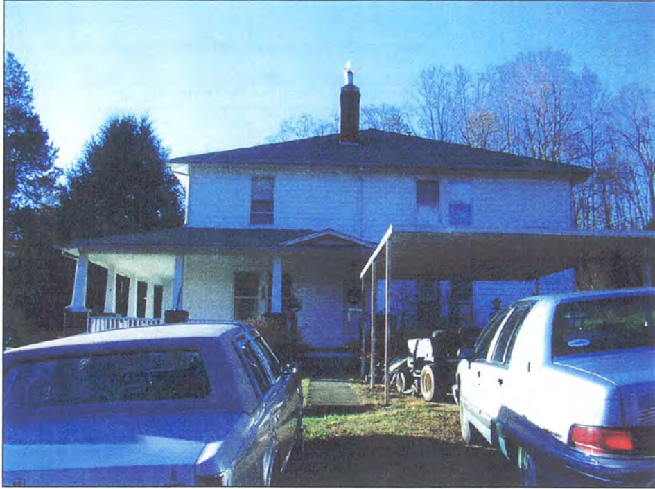
Figure 12: Stacy House, side (east) elevation.
