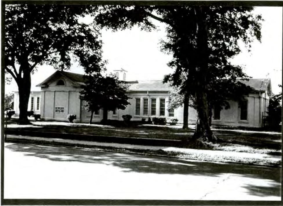
Plate VII.1 Former Salisbury Graded School, 314 North Ellis Street (1881 Block) (#1)
