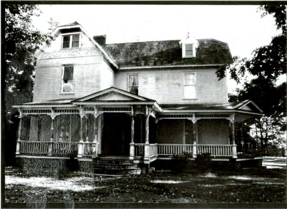
Plate VII.23 David A. Atwell House II, 404 West Kerr Street (#16)
