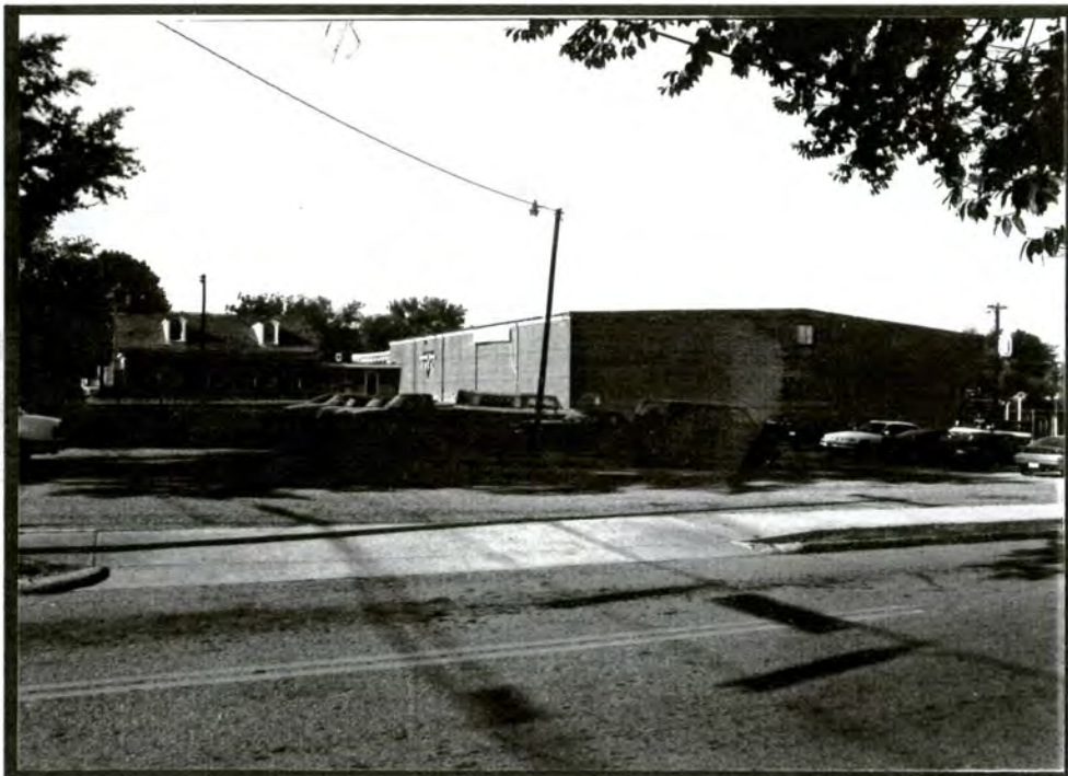
Plate IV.4 400 Block of West Liberty Street, SW Side
