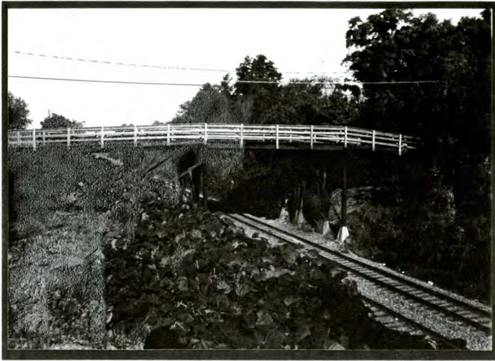
Plate VII.5 Ellis Street Bridge (#2)
