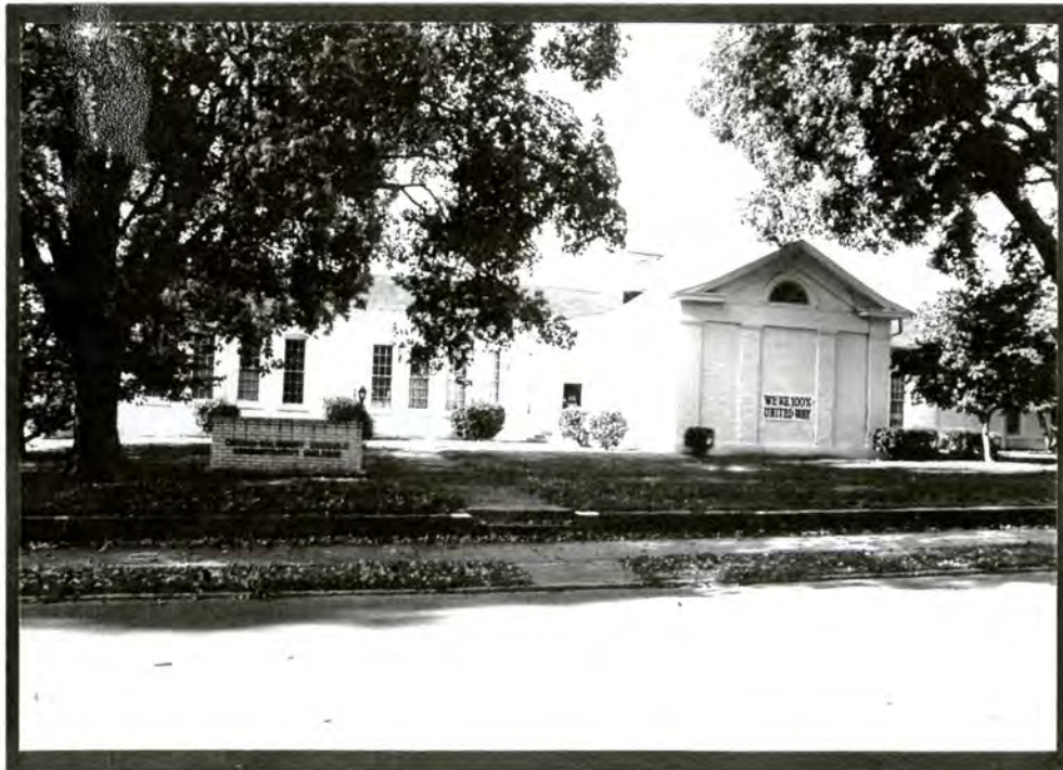
Plate IV.10 Former Salisbury Graded School, 314 North Ellis Street (1881 Block) (#1)
