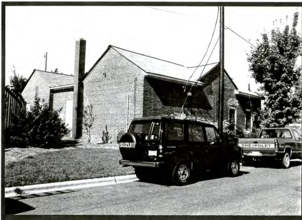
Plate V.10 Former Salisbury Waterworks Emergency Power Plant, 404 North Jackson Street
