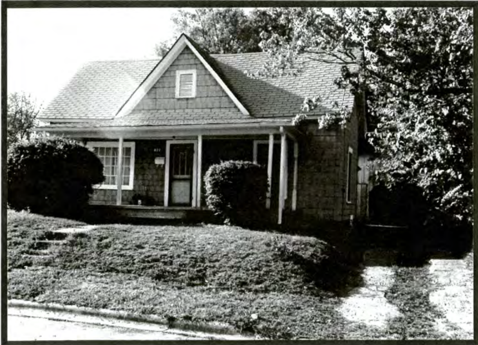
Plate V.6 422 North Caldwell Street
