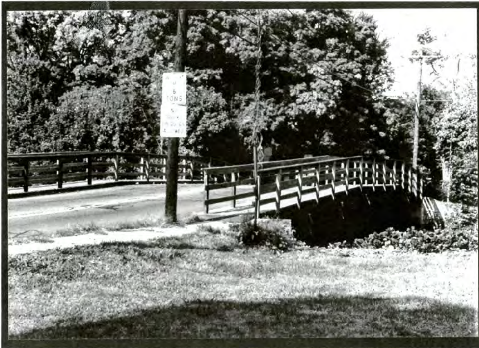
Plate VII.6 Ellis Street Bridge (#2)
