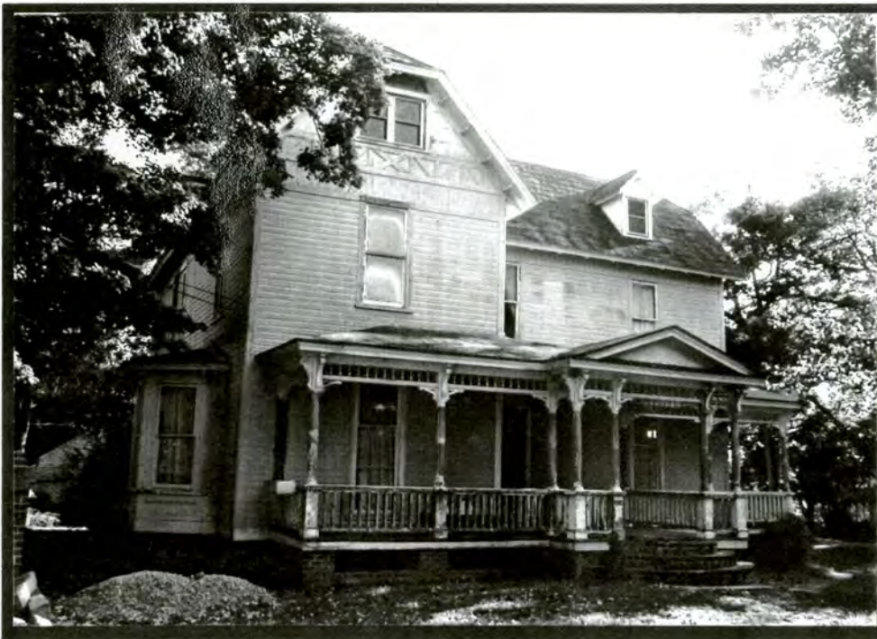
Plate VII.24 David A. Atwell House II, 404 West Kerr Street (#16)
