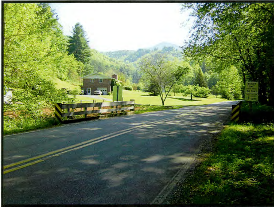
Figure 1: Bridge No. 36. Looking east on SR 1388.
