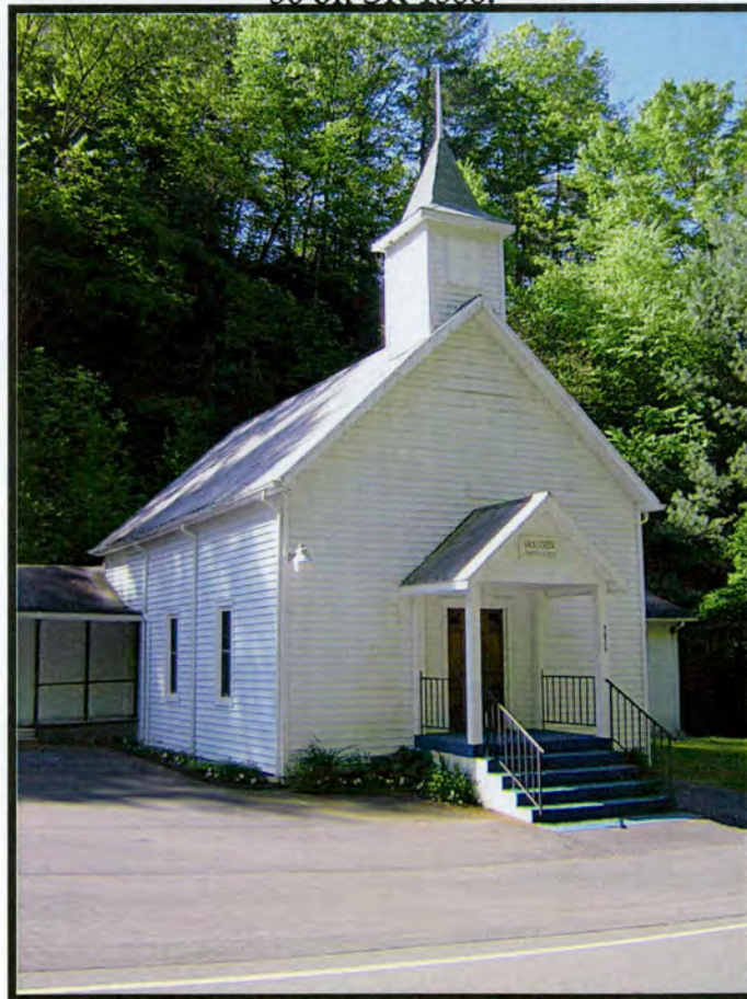
Figure 8: Front (northwest elevation)
