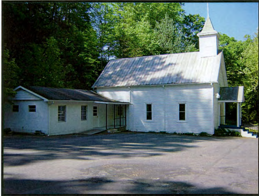
Figure 11: Side (northeast) elevation.
