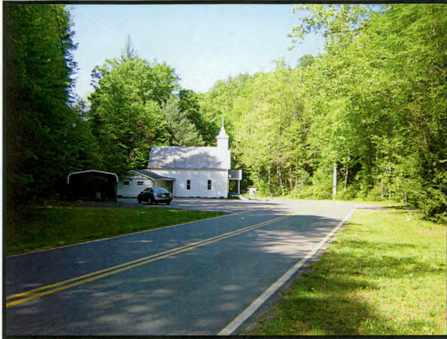
Figure 7: Dick's Creek Baptist Church setting. Looking west from Bridge No. 36 on SR 1388.
