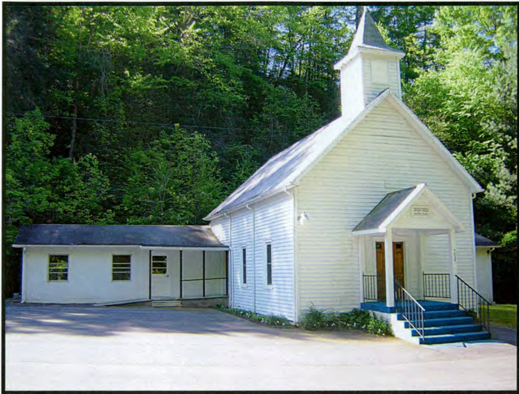
Figure 9: Front (northwest) elevation showing 1960s concrete block addition.
