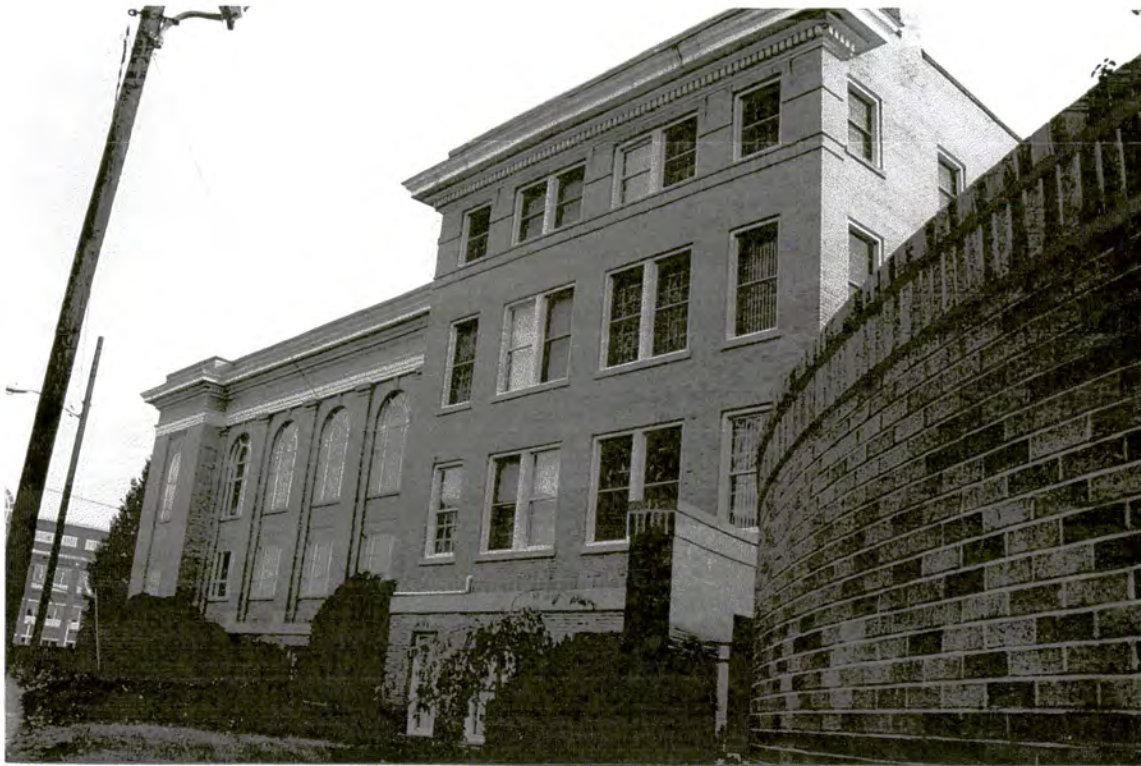
Plate 31: First United Methodist Church - original 1925 block, north side and west rear elevations
