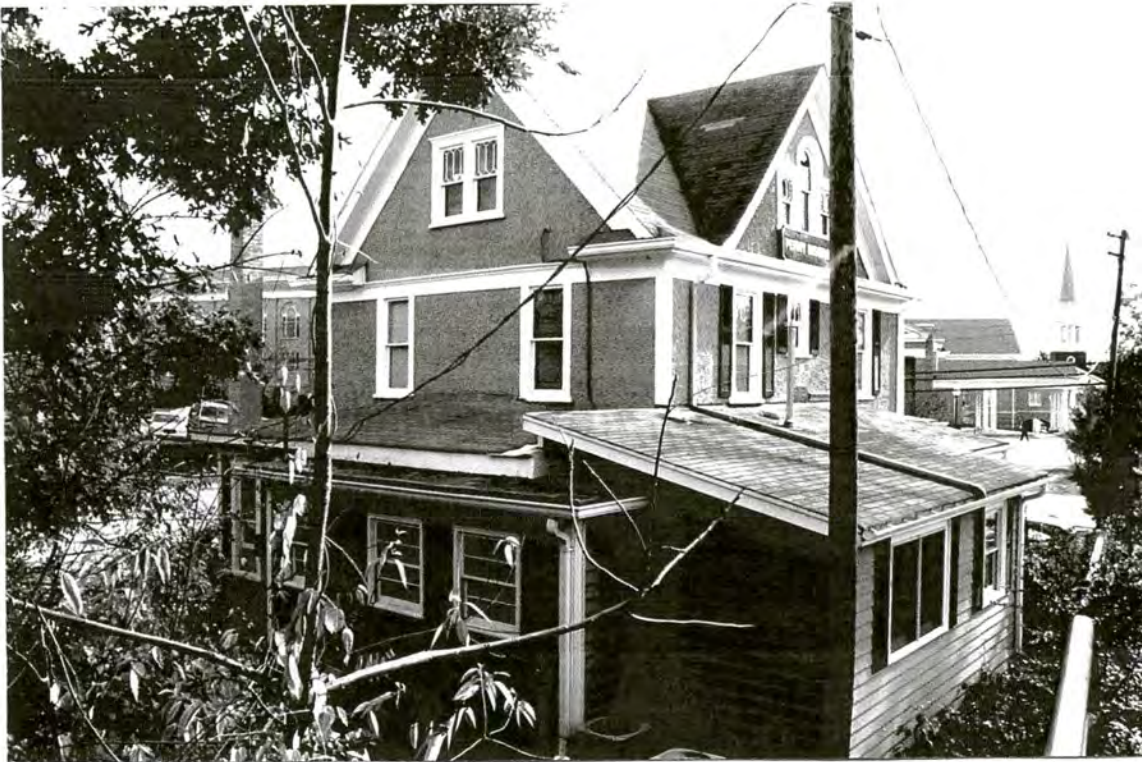
Plate 48: Hill-Hunter House – north rear and west side elevations
