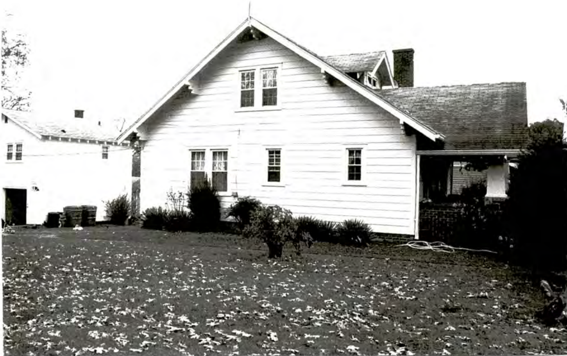
Plate 52: Bungalow at 825 Sixth Avenue West, Hendersonville (URS #2) – west side elevation
