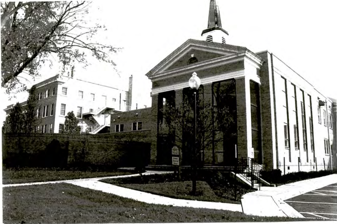
Plate 35: First United Methodist Church – Brunson Memorial Chapel at right, original 1925 block at left, looking southeast
