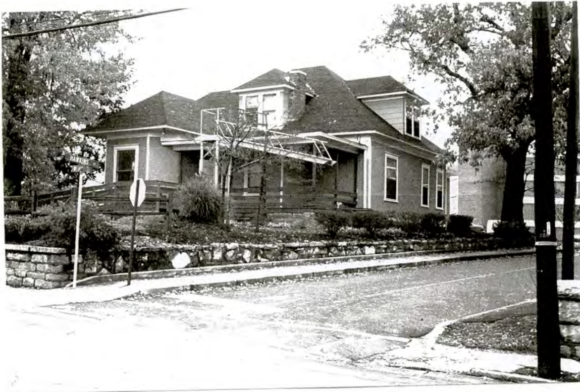
Plate 58: Former House at northwest corner of Hawkins Street and Sixth Avenue West (URS #8) – south front and east side elevations
