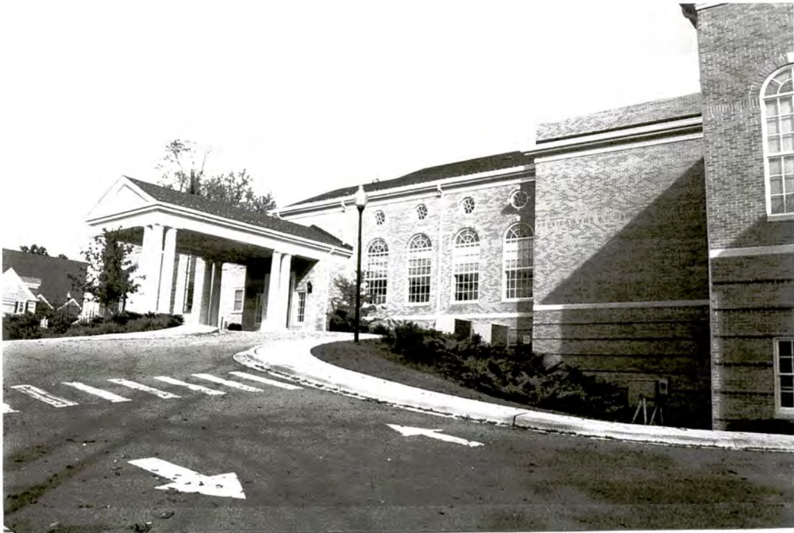
Plate 36: First United Methodist Church – 1990s/2000s addition, looking northeast
