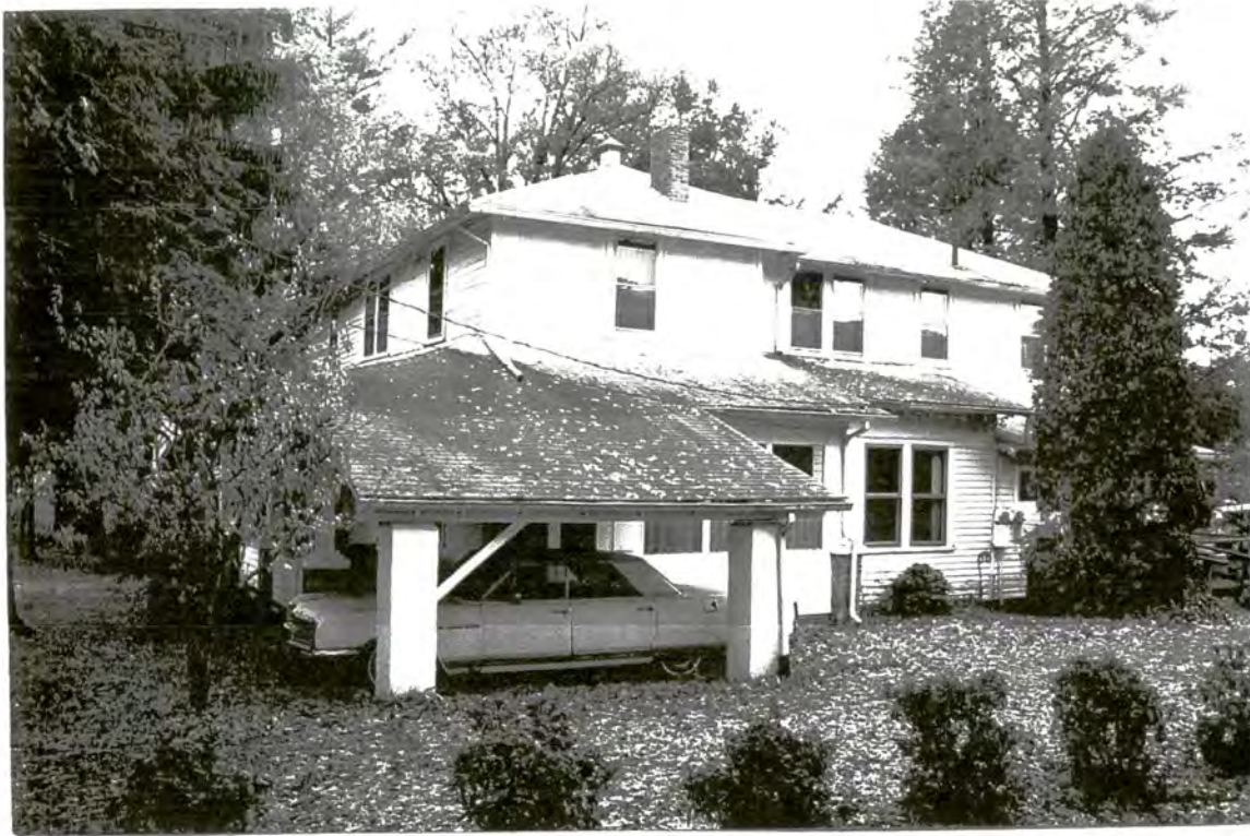
Plate 54: Foursquare at 747 Sixth Avenue West, Hendersonville (URS #4) – east side and south front elevations
