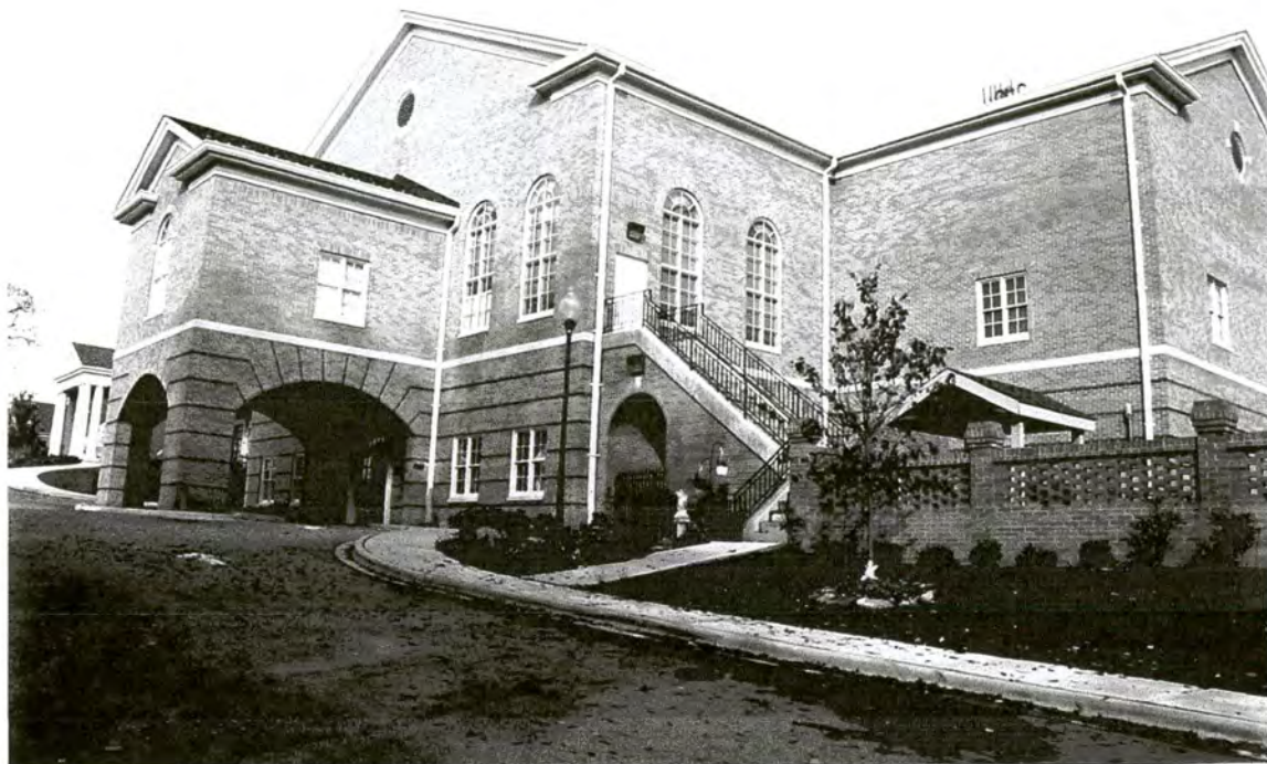
Plate 37: First United Methodist Church – 1990s/2000s addition, looking northeast
