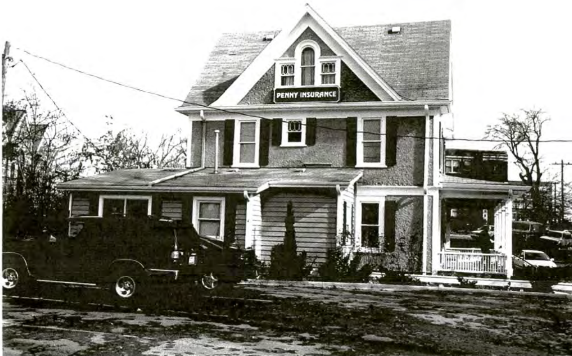
Plate 49: Hill-Hunter House – west side elevation
