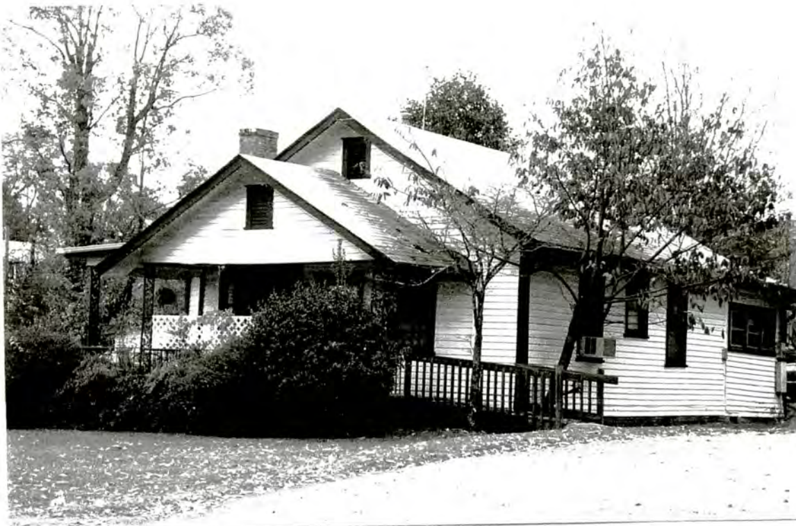
Plate 56: Gable-front House at 728 Sixth Avenue West, Hendersonville (URS #6) (Pampered Palate Café) – north front and west side elevations
