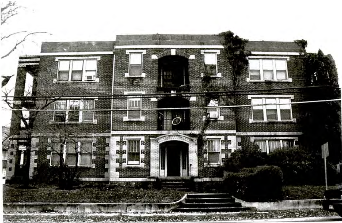
Plate 39: Former Bellevue Apartments – south front elevation
