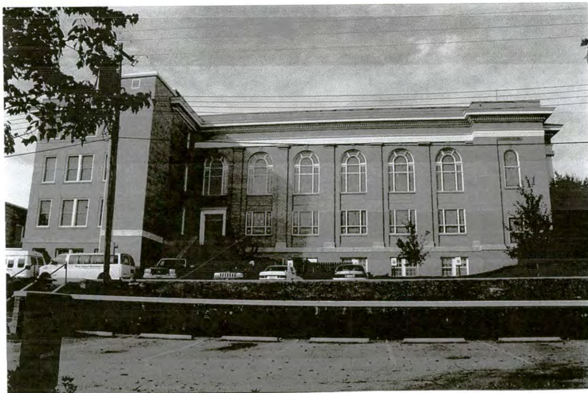
Plate 28: First United Methodist Church – original 1925 block, south side elevation
