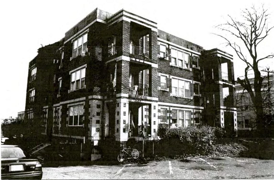
Plate 43: Former Bellevue Apartments – north rear and west side elevations
