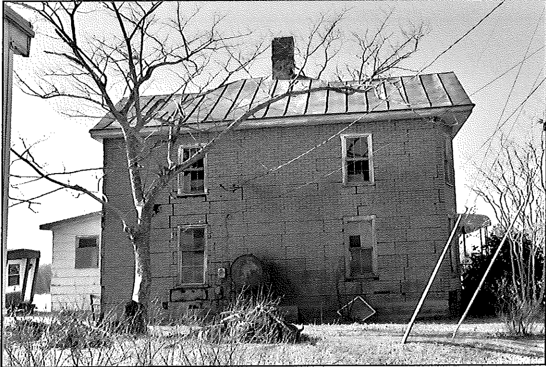
Photo 5 Johnny and Ninnie Bryant House (Property 1), North Elevation
