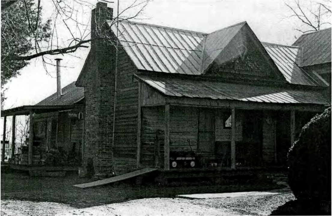
Figure 7. Dwelling House. Period II - west (main) and north elevations. Photographed February 11, 2003.
