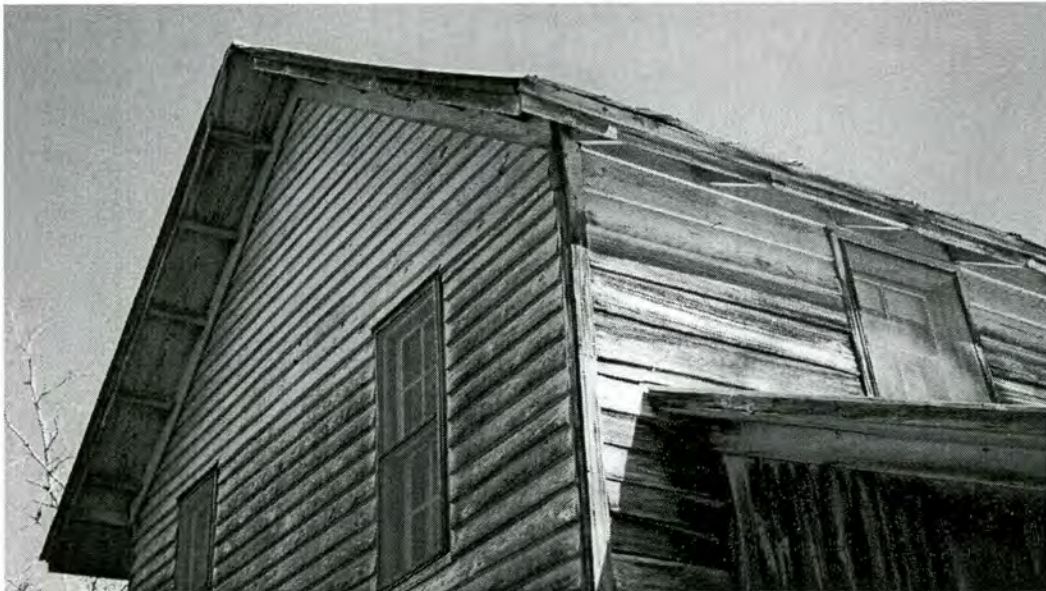
Figure 6. Dwelling House. Period I - detail of eaves, southwest corner. Photographed February 11, 2003.
