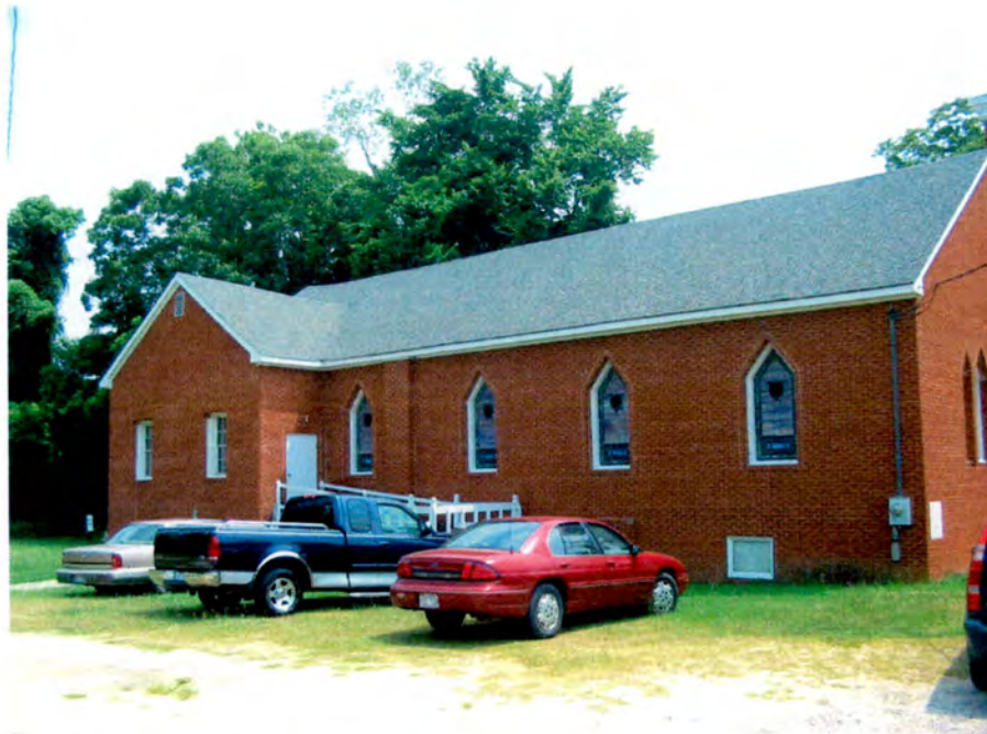
Plate 2 St. John's A.M.E. Zion Church, Side (West) Elevation, Looking Northeast from Church Parking Lot.
