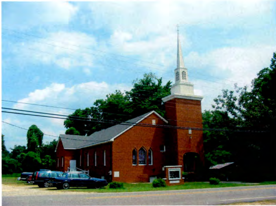
Plate 1 St. John's A.M.E. Zion Church, Looking North
