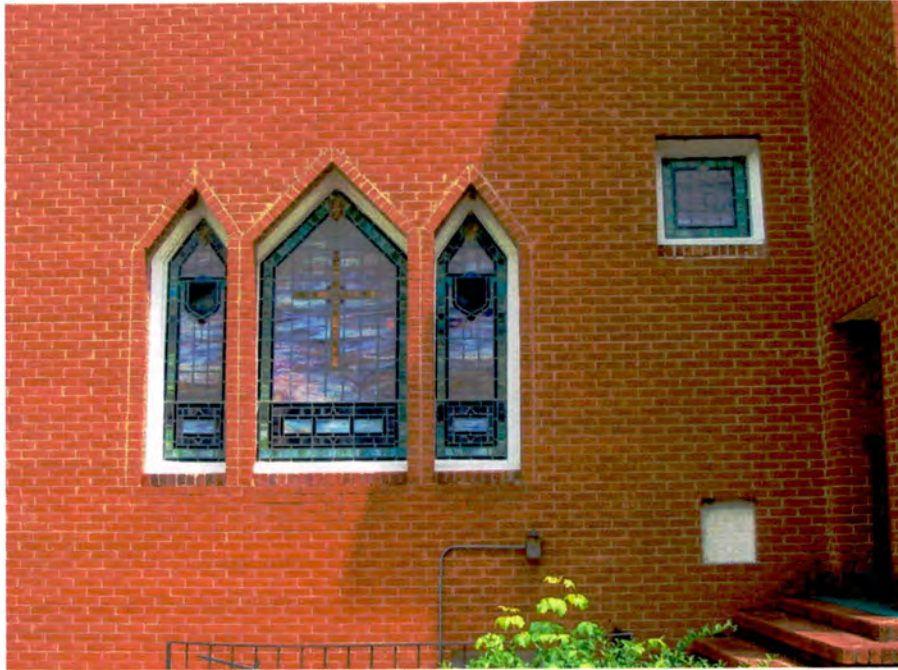
Plate 3. St. John's A.M.E. Zion Church, Detail of Façade Showing Modern Brick Veneer (1976) and Pointed Arch Windows.
