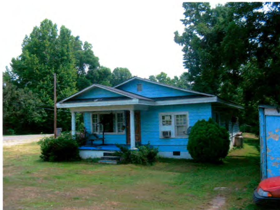
Plate 6. House (130 Liberia Street) on Corner of S.R. 2237 and Liberia Street, Looking East.
