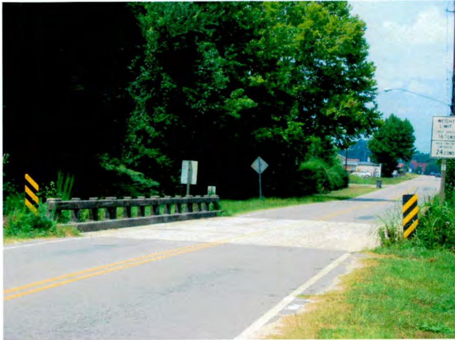
Plate 7. Bridge No. 94, Looking West From Factory Site on East Side of Bridge.
