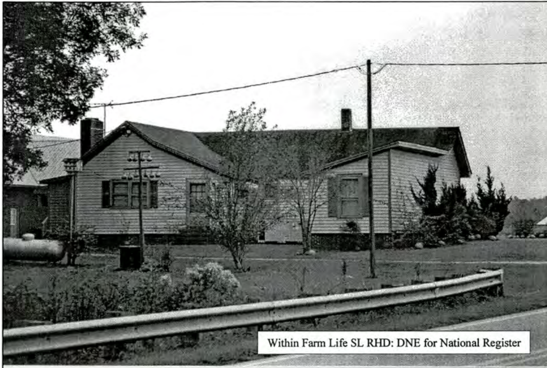
Property 10: Bridgman Perry House, 8817 NC 171 (North and West elevations) Figure 42
