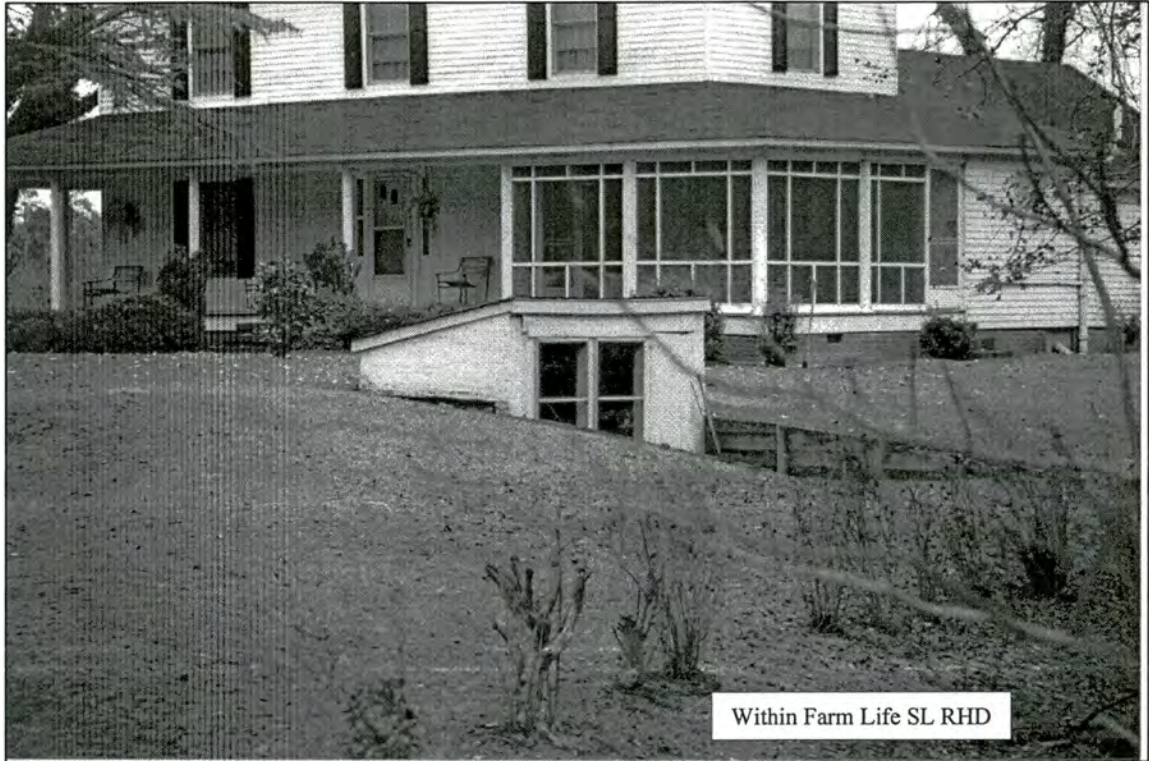
Property 3: Roberson-Gurkin House, garden house, south and west elevations Figure 18
