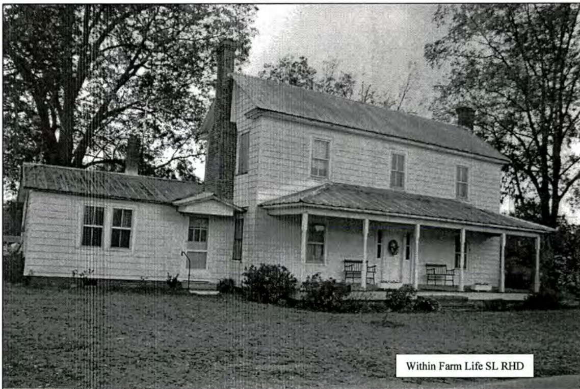
Property 15: W. B. Harrington Farm, N. elevation of house Figure 34
