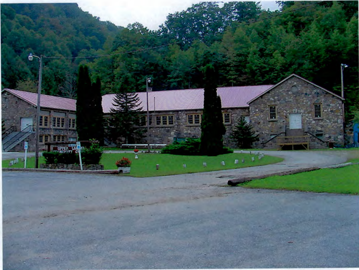
Ebbs Chapel School, front façade, overall view to northwest (September 2004)
