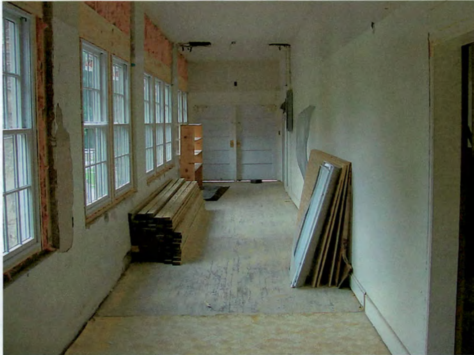
Ebbs Chapel School, interior, 1950s wing (September 2004)
