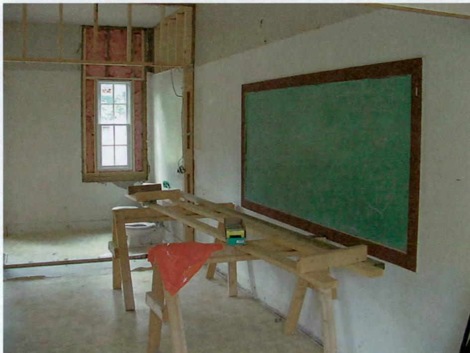
Ebbs Chapel School, interior, 1950s wing (September 2004)
