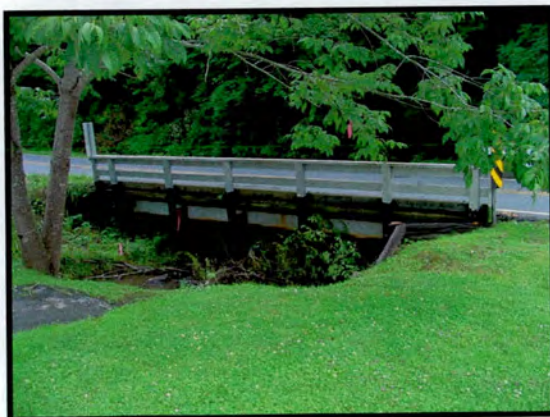
Figure 6. Bridge No. 246 on SR 1503
