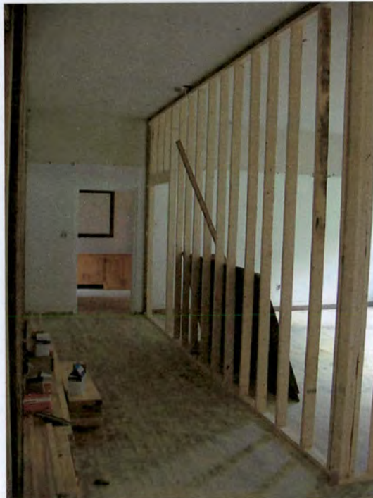
Ebbs Chapel School, interior, 1950s wing (September 2004)
