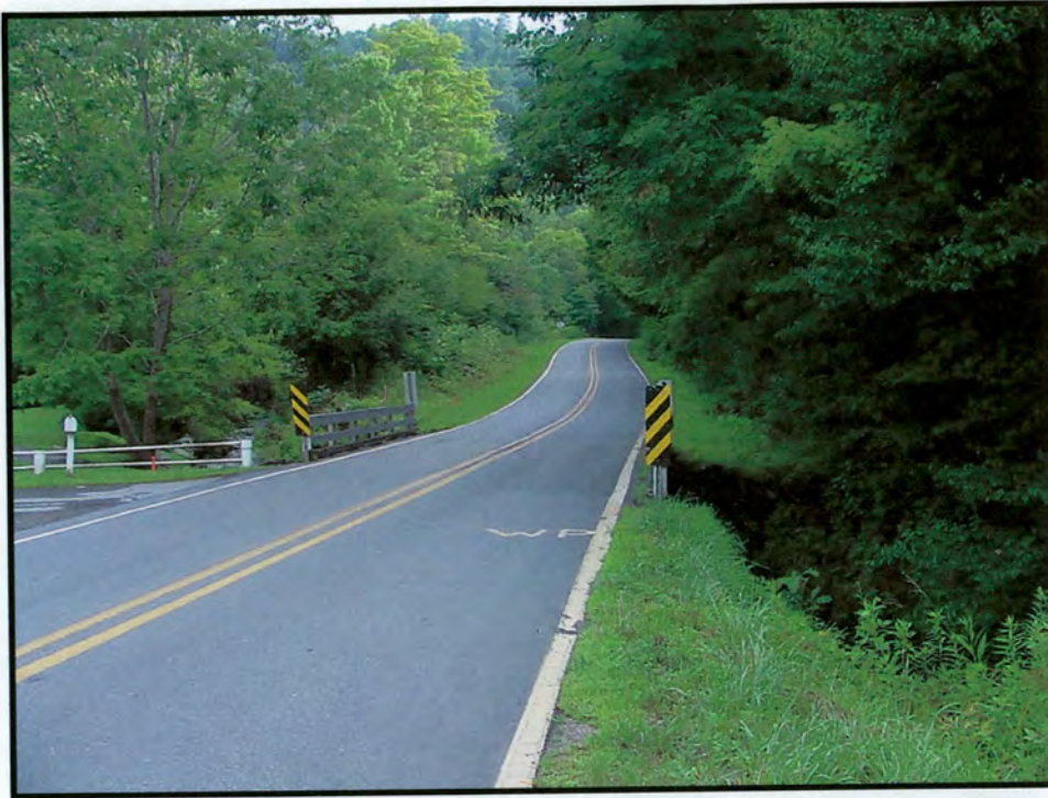
Figure 2. Bridge No. 246, view to northeast along Laurel Valley Road (SR 1503)
