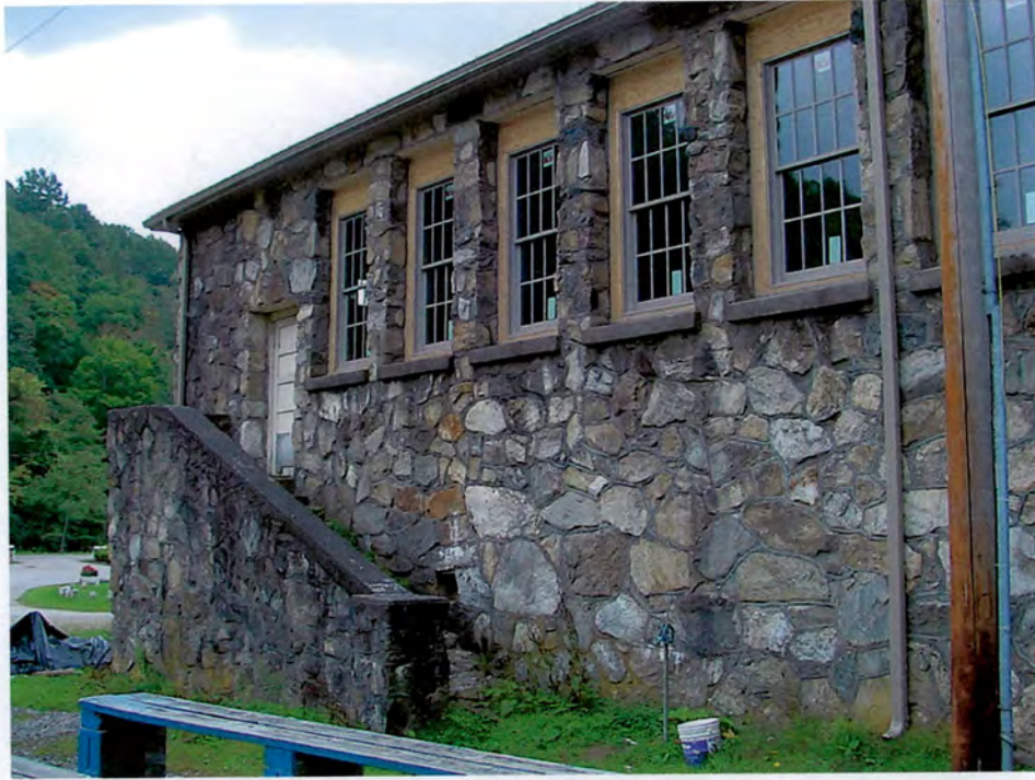
Ebbs Chapel School, auditorium (NE side elevation) (September 2004)
