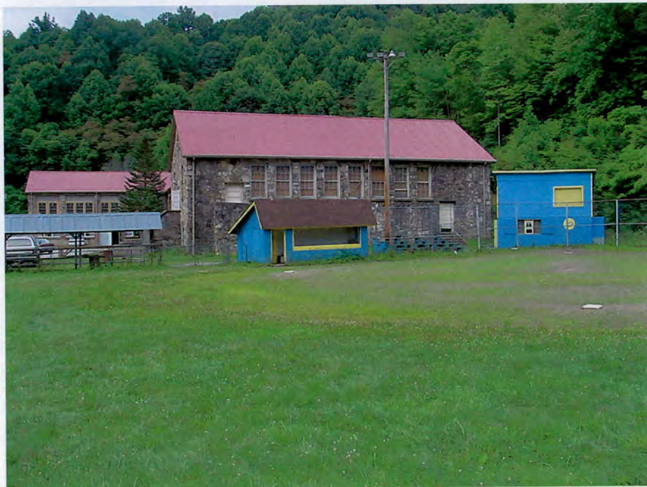
Ebbs Chapel School, baseball field and east end of building (July 2004)
