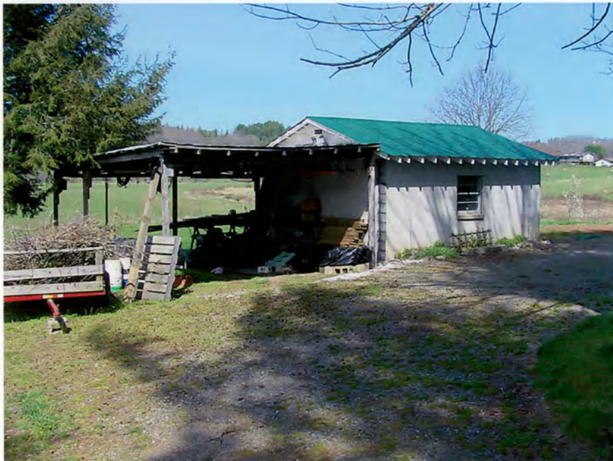
Shed #2, south and west sides, oblique view to northeast
