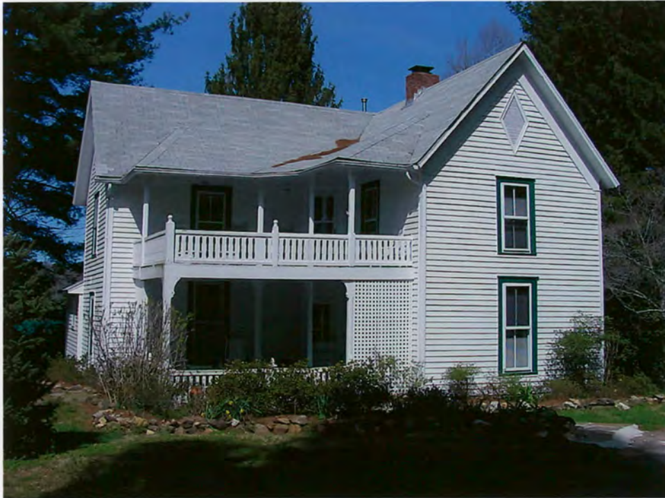
Erwin Patton House, front façade, overall view to north
