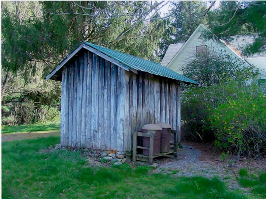
Shed #1, north and west sides, oblique view to southeast
