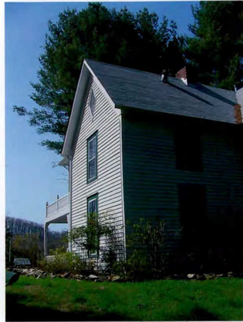
South and east elevations, oblique view
