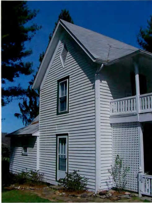
West elevation, oblique view
