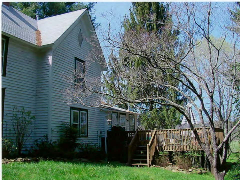
East elevation, oblique view to northwest
