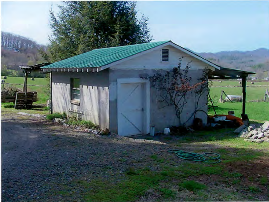
Shed #2, south and east sides, oblique view to west
