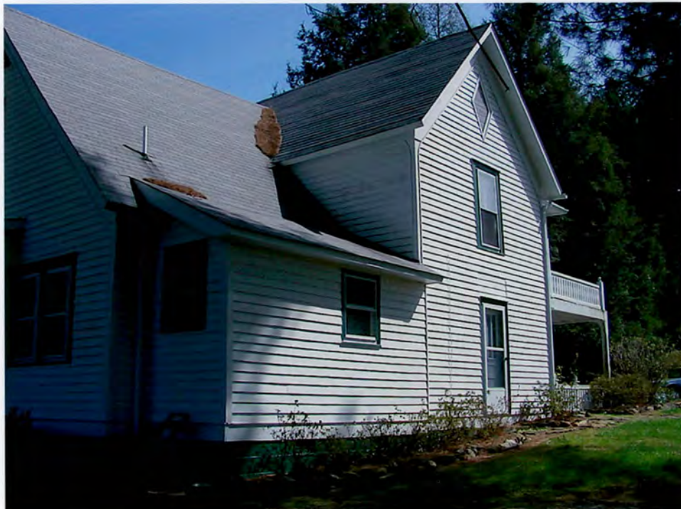
West elevation, oblique view to southeast
