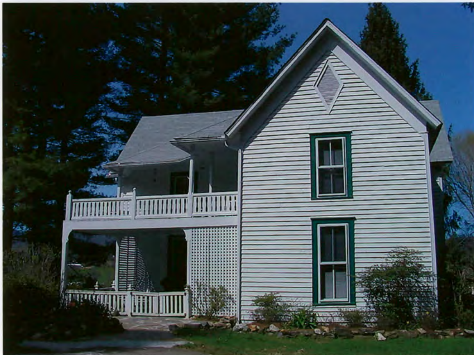
Erwin Patton House, front (south) facade
