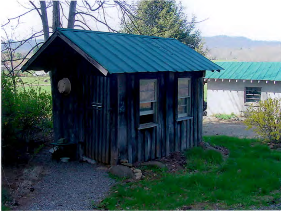
Shed #1, south and east sides, oblique view to northwest
