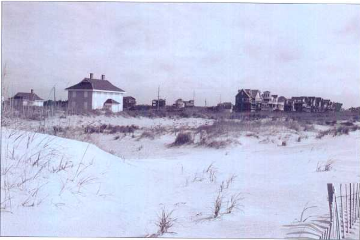
Plate 23: Looking northeast from ocean strand toward station house and messroom at left, and modern development on both sides of NC 12 at right, in April 2006
