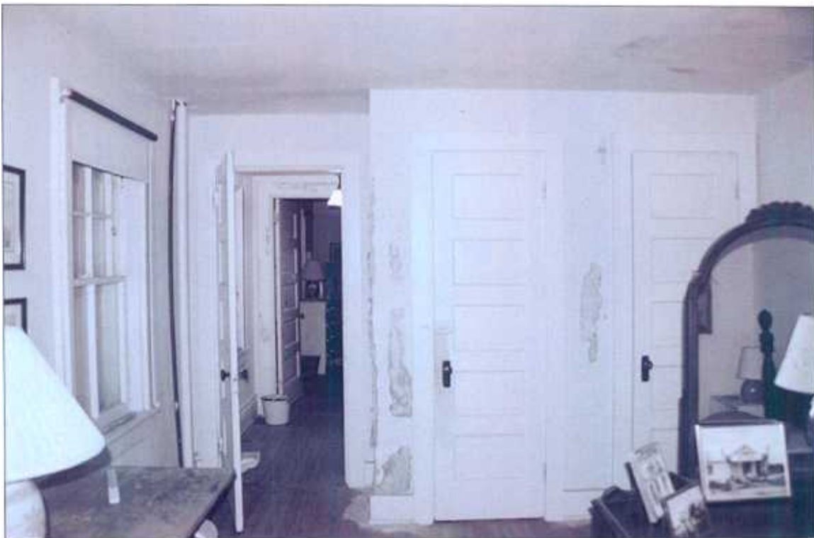
Plate 18: Surfmen's room (Room 15), including original closets, doors, and sash, in March 2006
