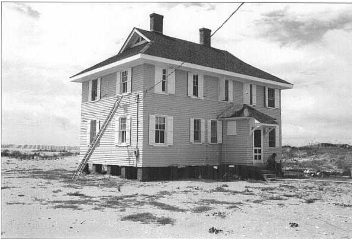
Plate 8: December 2004 image of north rear and east side elevations of station house
