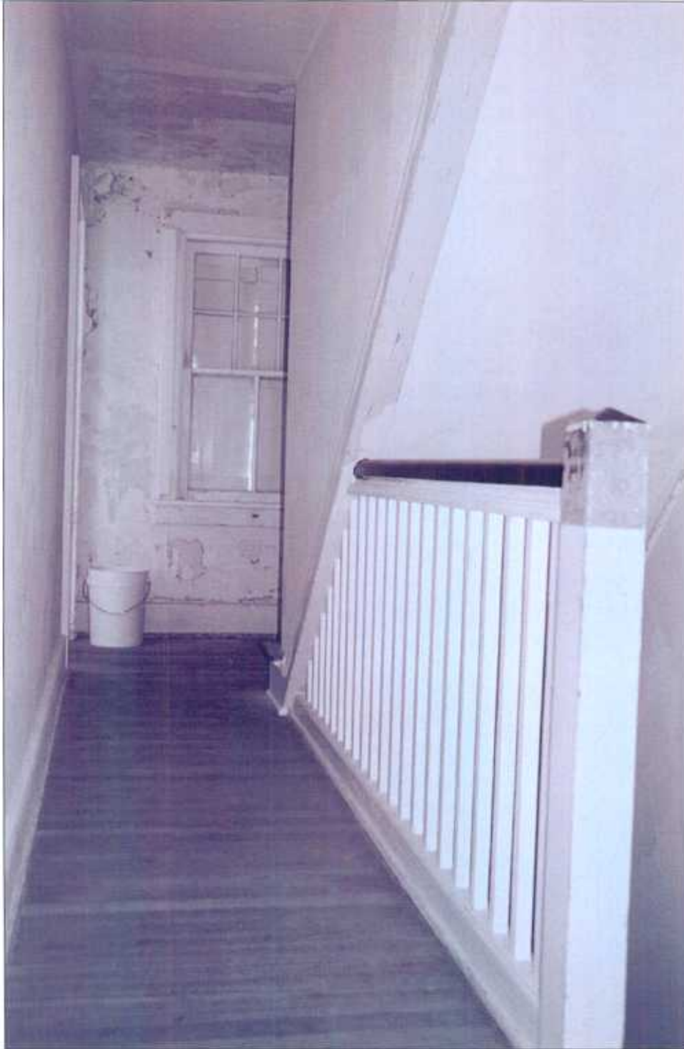
Plate 16: Second-floor hall (Room 12) in March 2006
