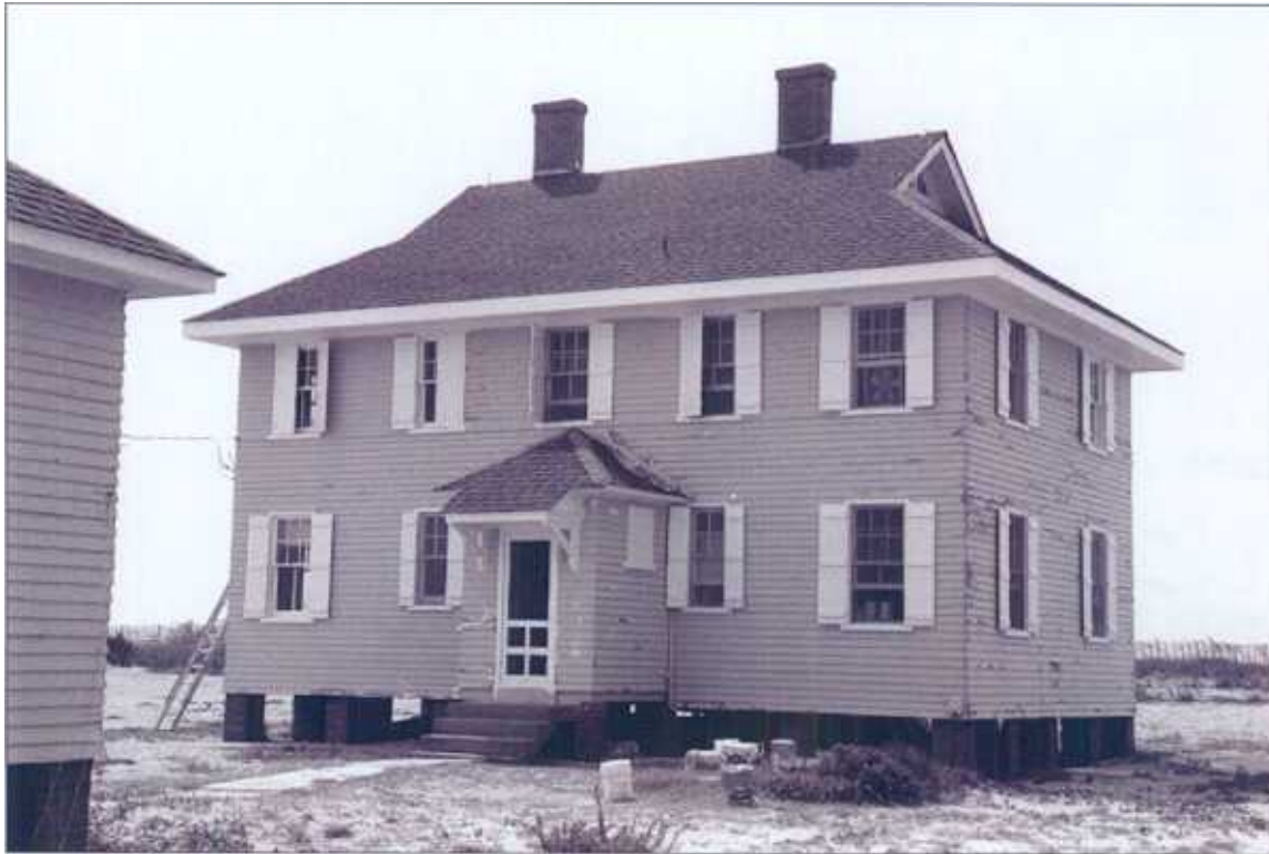
Plate 9: December 2004 image of north rear and west side elevations of station house
