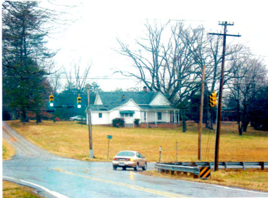
Plate 5. Waitsel Monroe Smith House, West and North Elevations, Looking Southeast.
