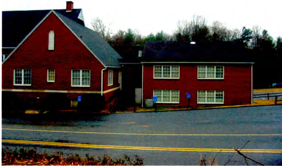
Plate 40. Colliers United Methodist Church, Side (North) Elevation of Church and Educational Building, Looking South.
