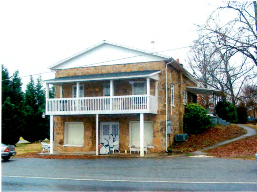
Plate 29. Store, Facade, Looking West.
