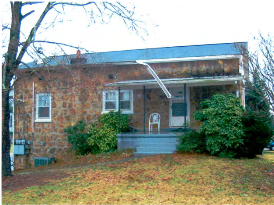
Plate 31. Store, Side (North) Elevation, Looking South.
