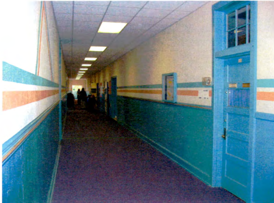
Plate 27. Baton School, Interior Corridor, Original School Building.
