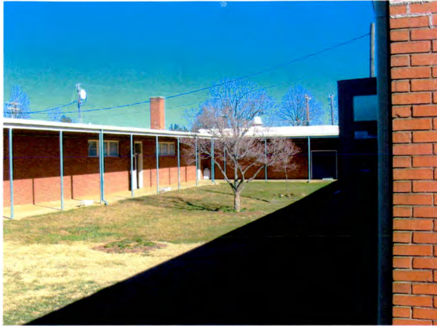
Plate 25. Baton School, 1952 Classroom Additions, Looking Northwest.
