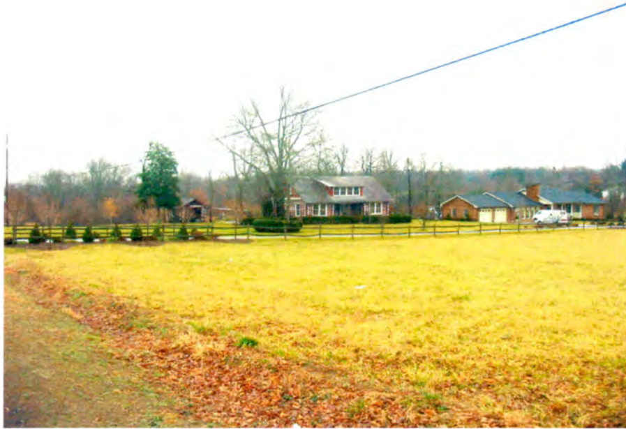
Plate 9. Elizabeth Bush House, Overall View of Bush House and Modern Ranch House, Looking Southeast.
