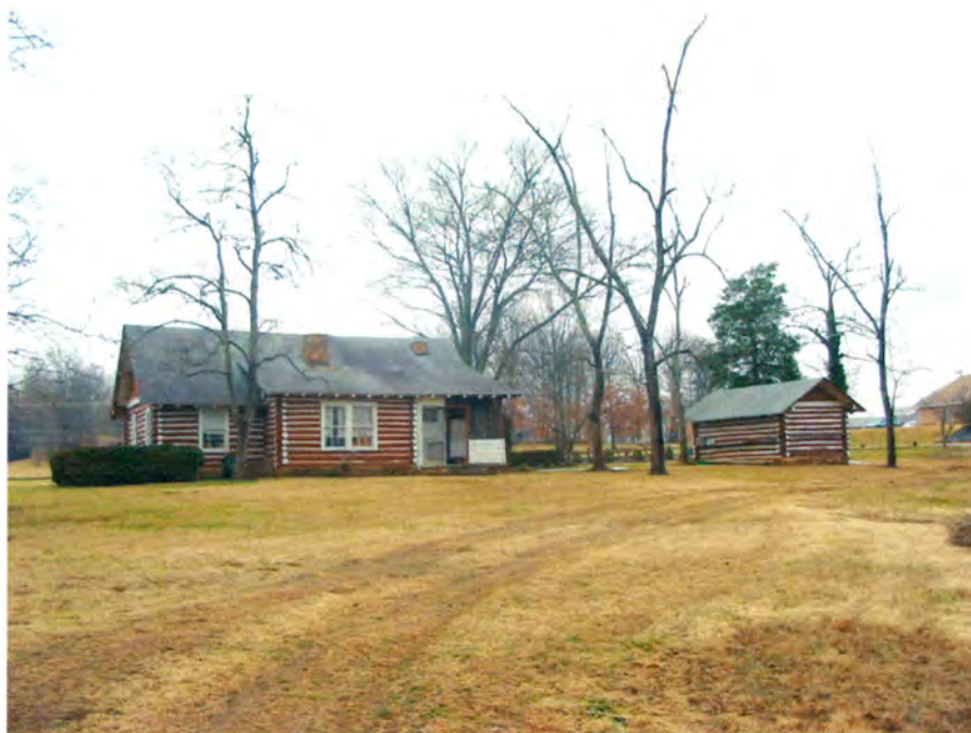
Plate 11. Elizabeth Bush House, Overall View of Bush House (Rear Elevation) and Garage, Looking Northwest.
