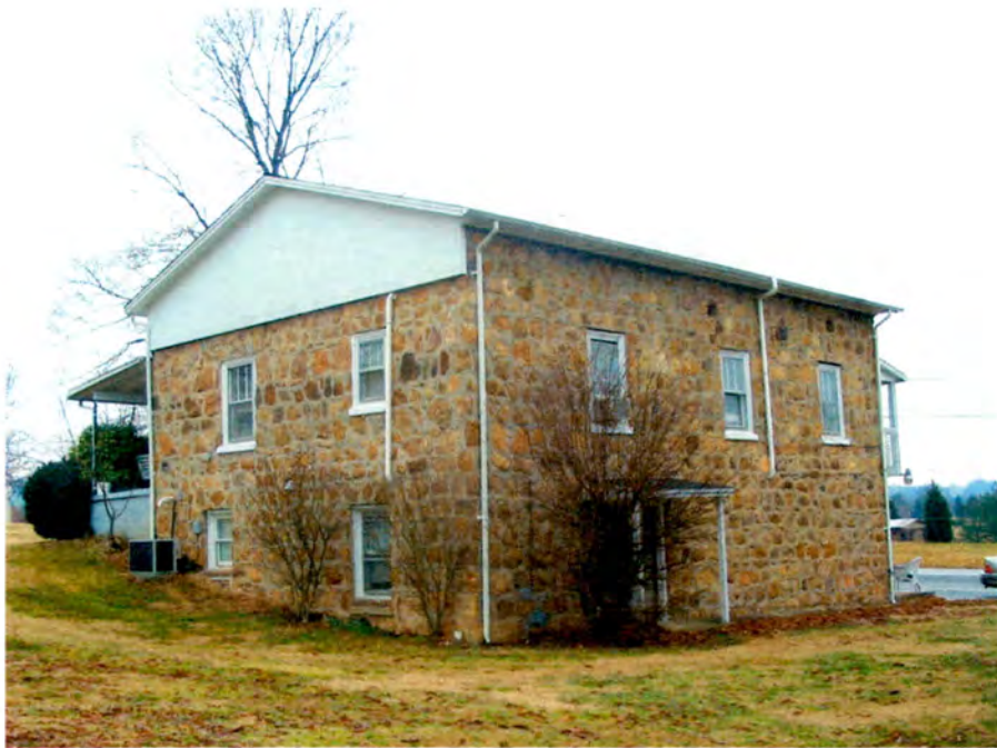
Plate 30. Store, Side (South) and Rear (West) Elevations, Looking Northeast.
