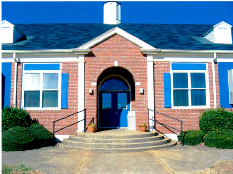
Plate 26. Baton School, Entrance Detail.
