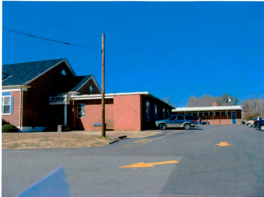
Plate 23. Baton School, Front and East Elevations and 1956 and 1960s Classroom Additions, Looking North.
