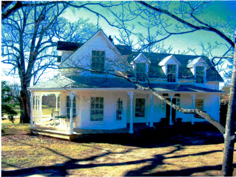
Plate 1. Waitsel Monroe Smith House, Facade, Looking West.
