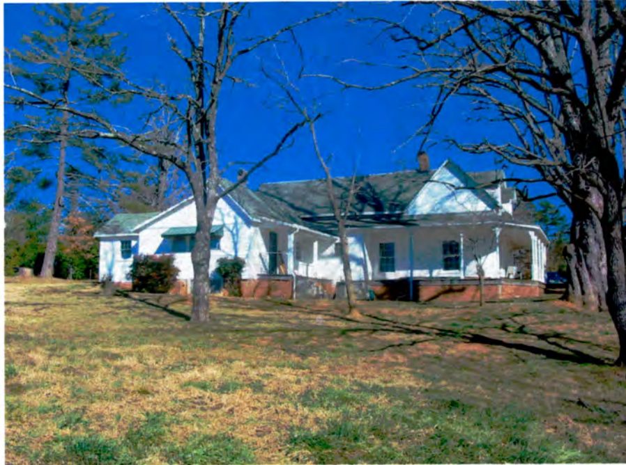
Plate 3. Waitzel Monroe Smith House, West Elevation, Looking East.
