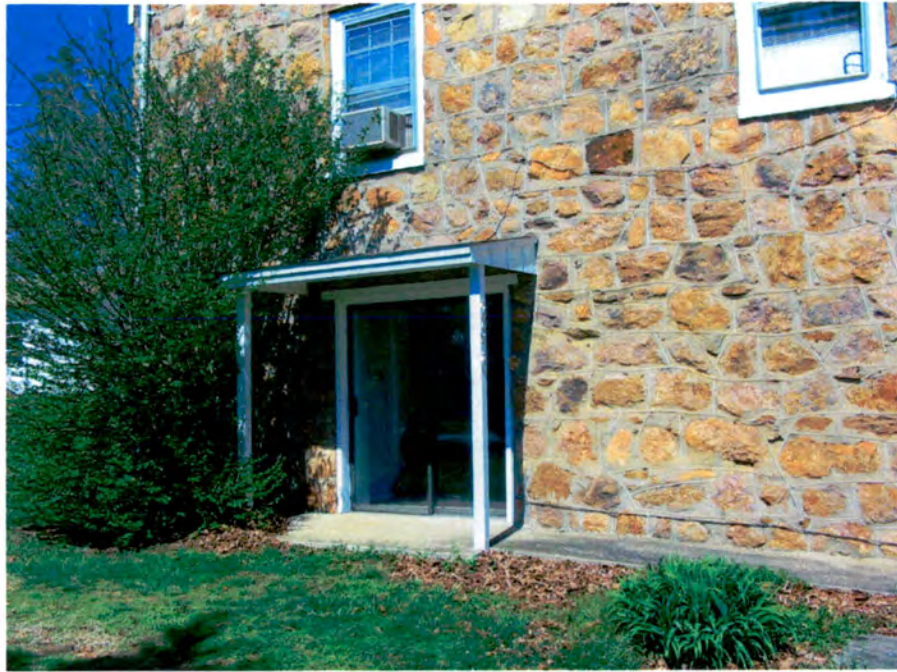
Plate 33. Store, Side (South) Elevation Showing Modern Sliding Glass Door, Looking North.
