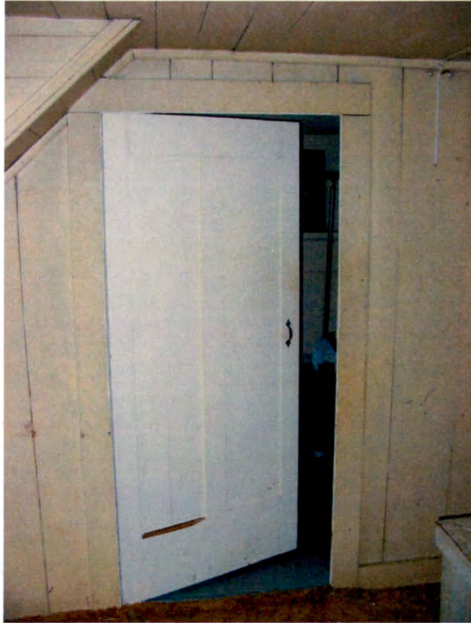
Plate 8. Waitzel Monroe Smith House, Interior, Door Detail
