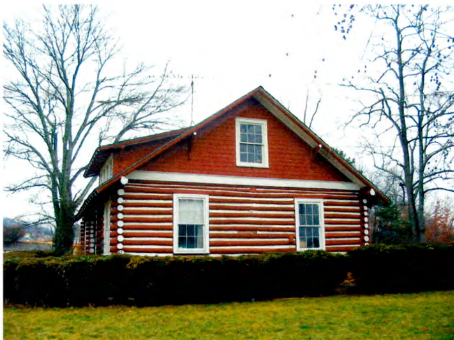
Plate 14. Elizabeth Bush House, Side (South) Elevation, Looking North.
