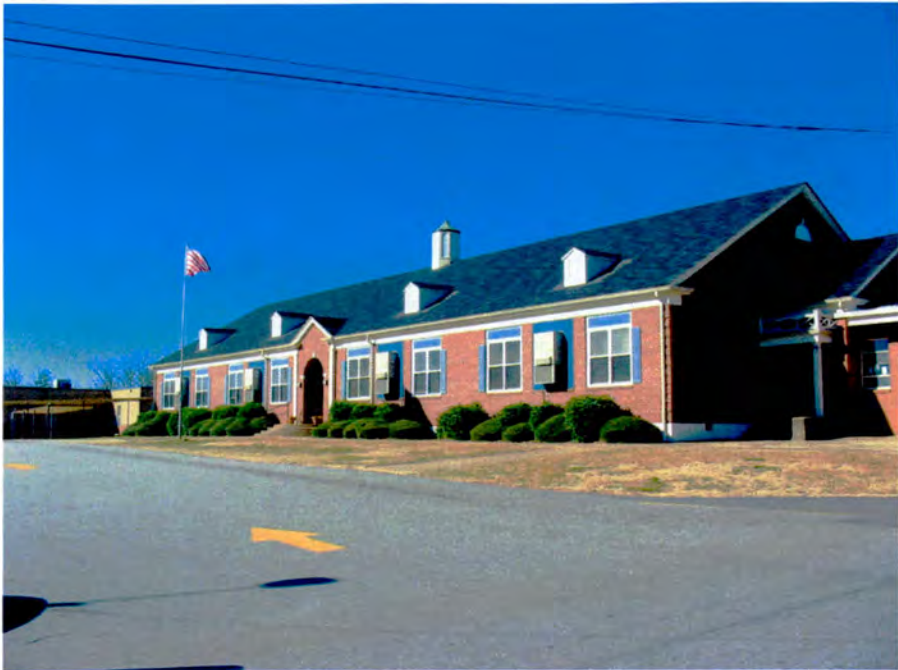
Plate 21. Baton School, Front (South) and Side (East) Elevations, Looking Northwest.
