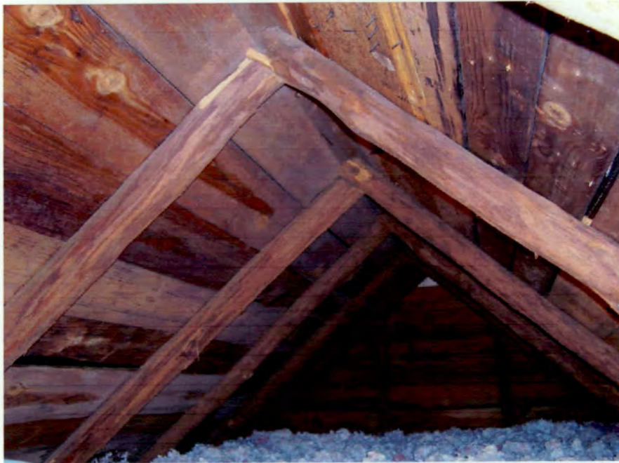
Stripped Pole Rafters in Original Log House
