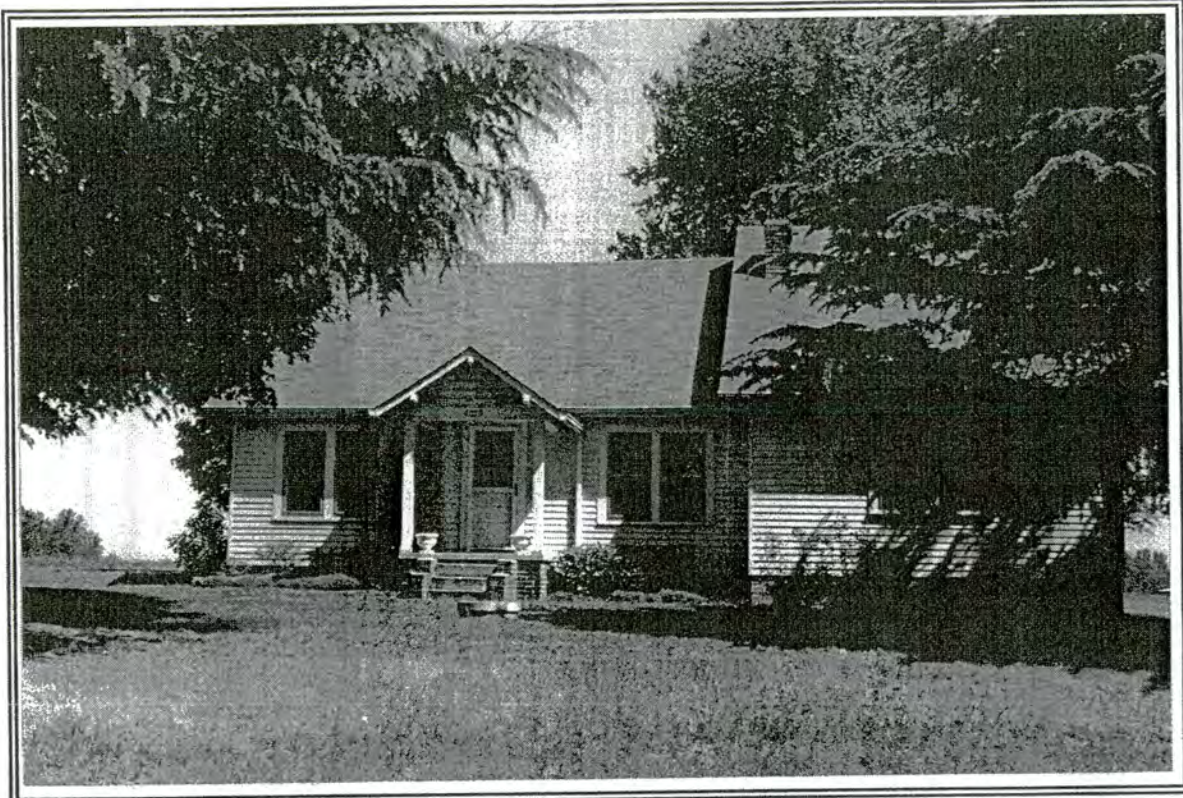
20. House and outbuildings, 4073 Glenn Hi Road
