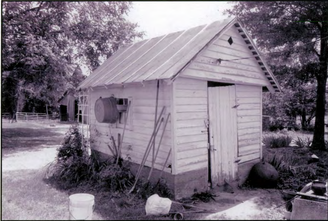
Well House (Facing SW)
