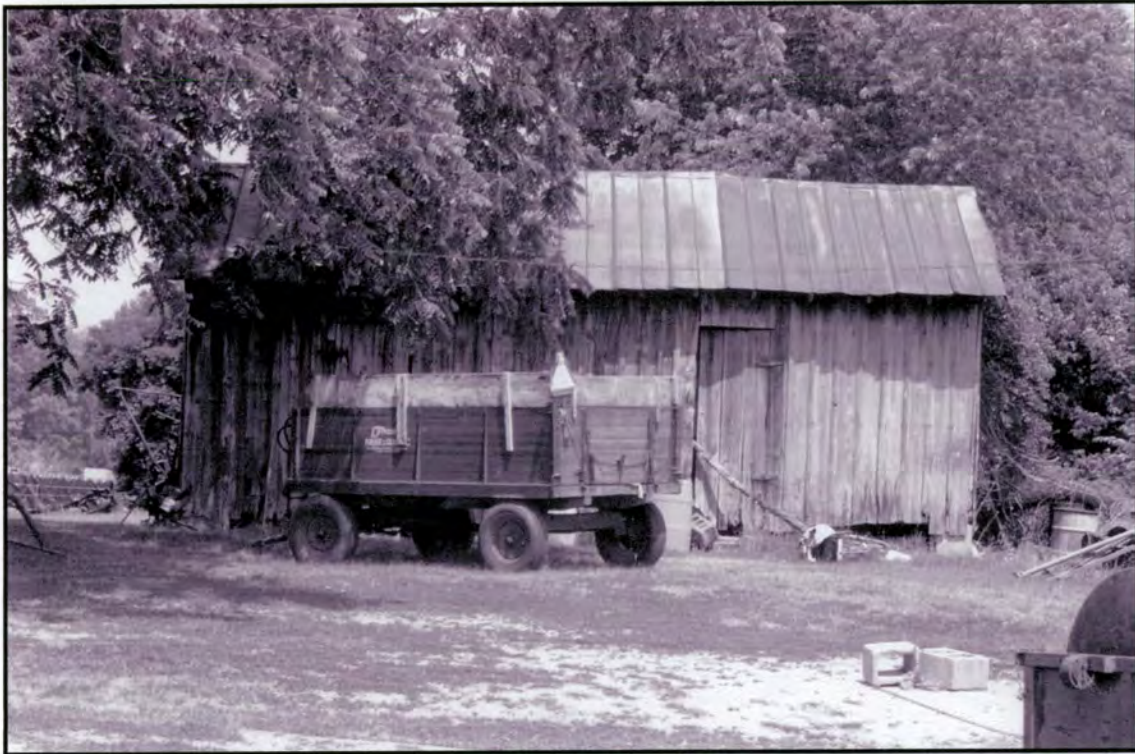
Packhouse (Facing E)
