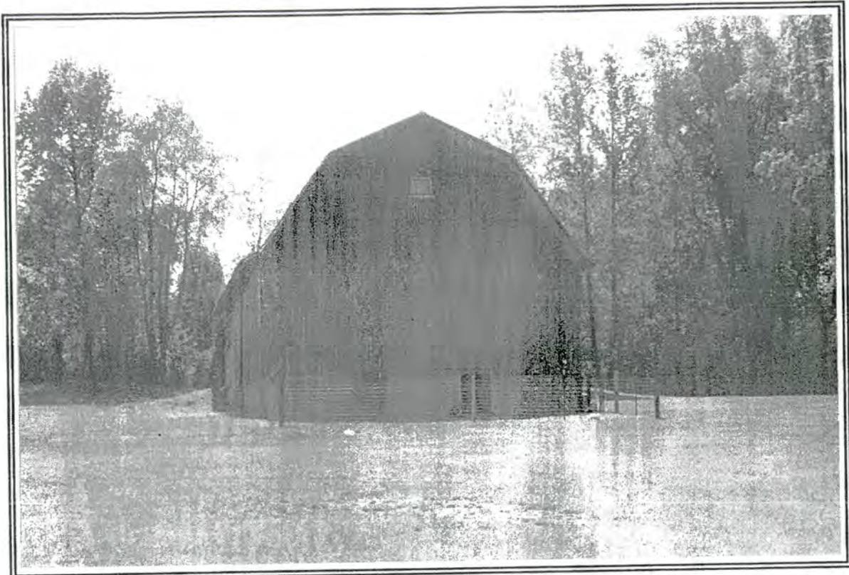
14. J. O. Tucker House and barn, 4157 High Point Road
