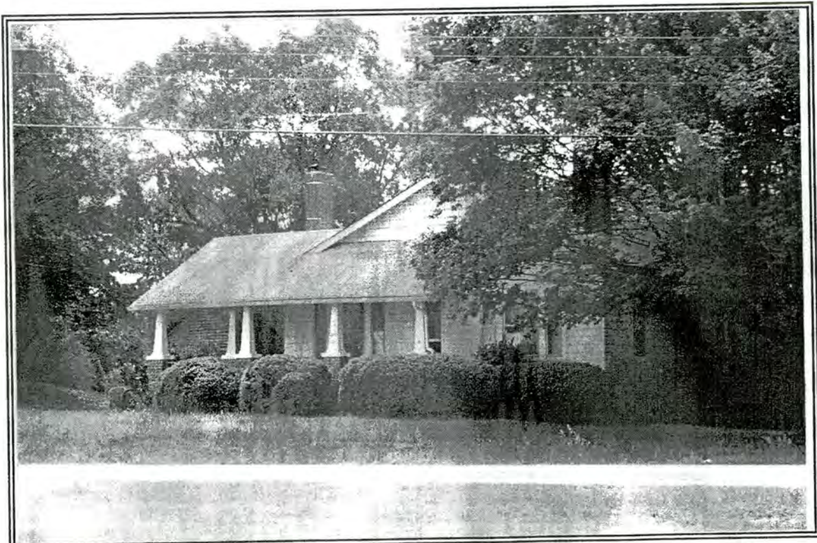
44. House, 4222 Kernersville Road
