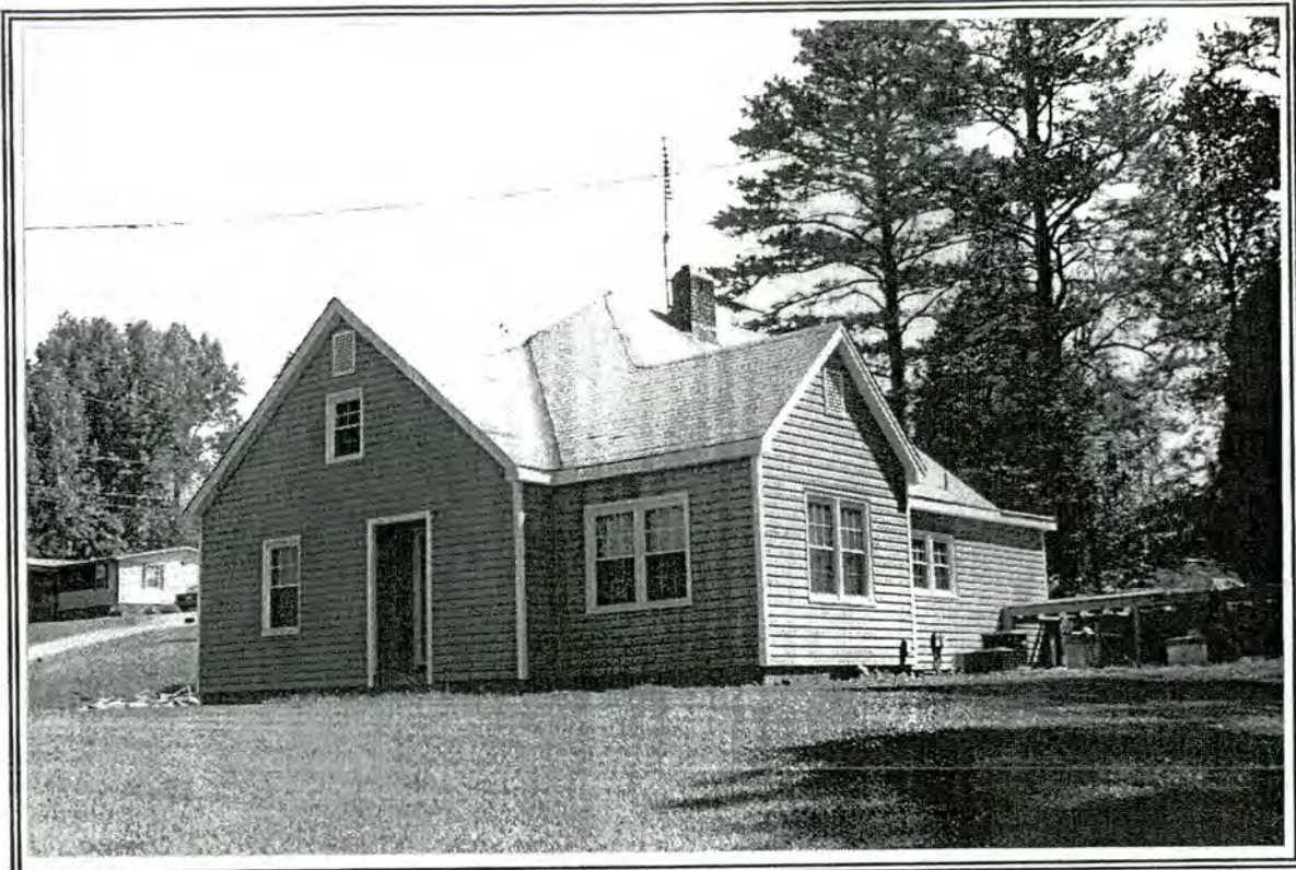
16. House, 4041 High Point Road
