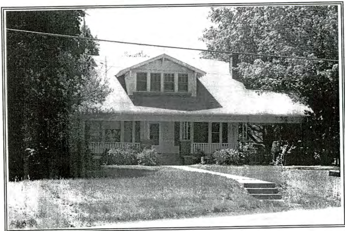
34. House, 4224 Kernersville Road
