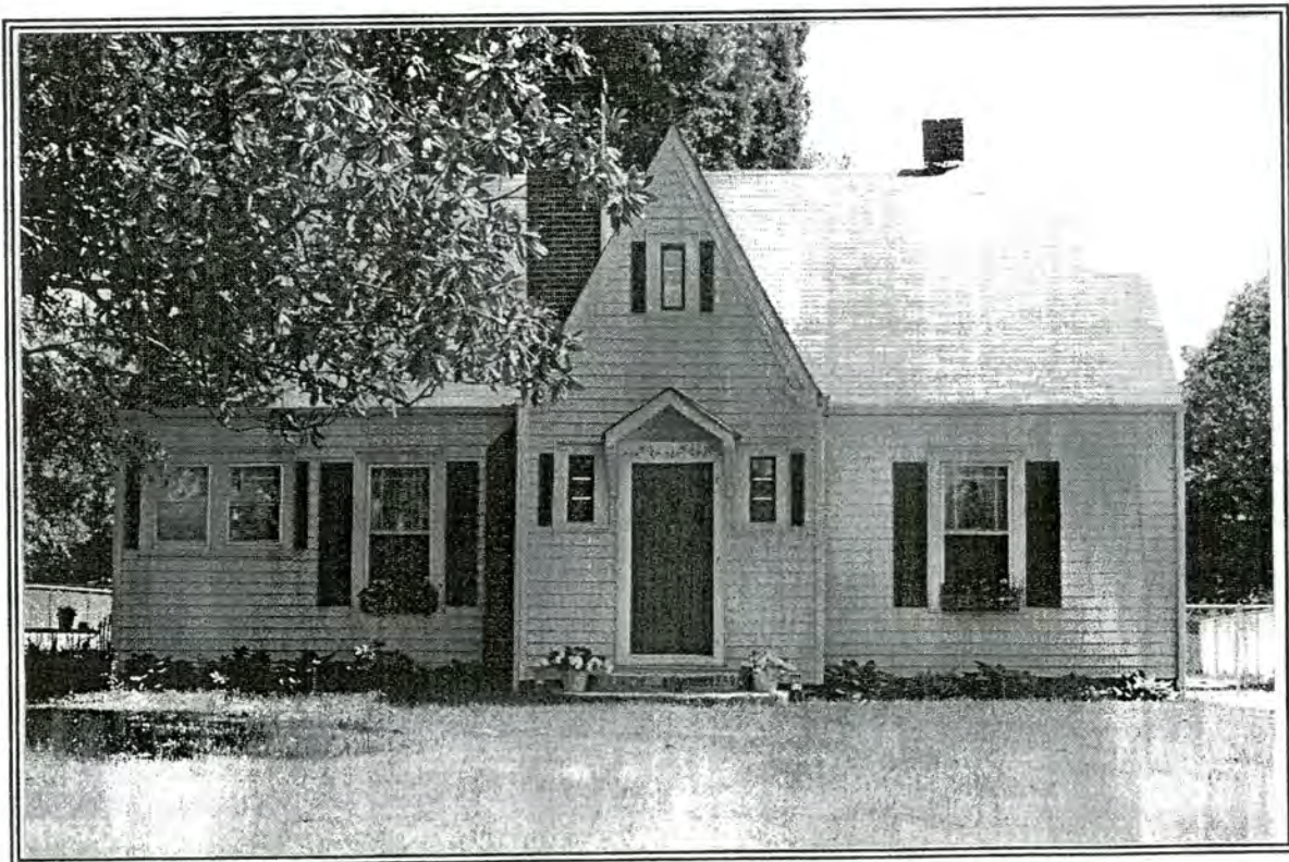
36. House, 125 Maynard Drive
