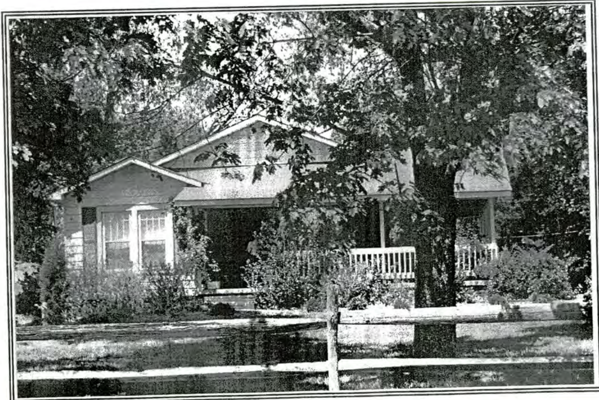
53. House, 4327 Old Winston Road
