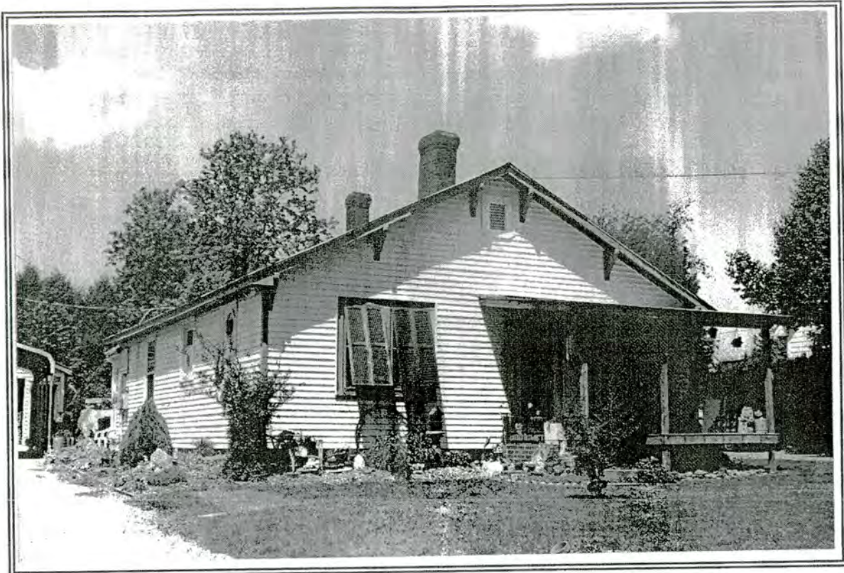
41. House, 760 Maynard Drive
