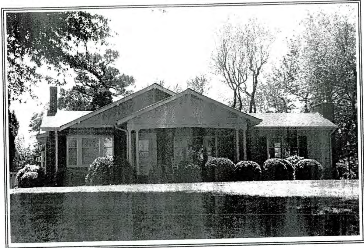
58. House, 4418 Old Winston Road
