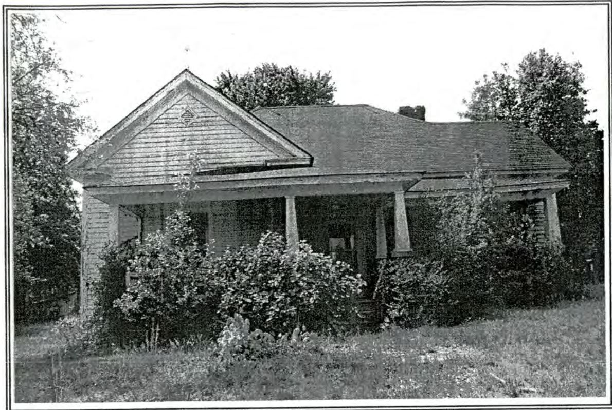
69. House, 500 Elliot Road
