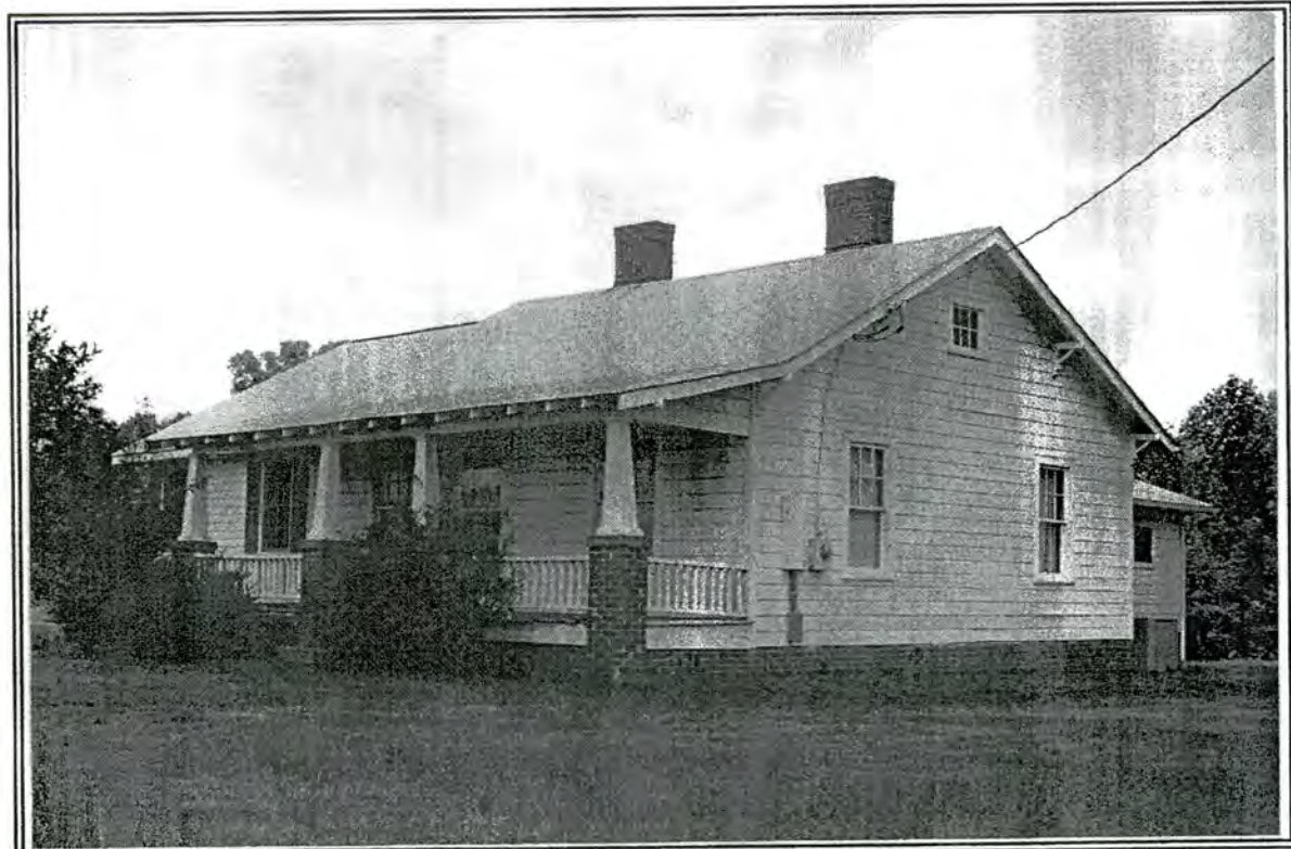
70. House, 535 Elliot Road
