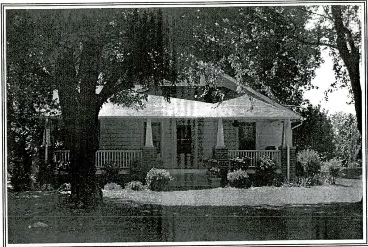
29. House, 4250 Kernersville Road
