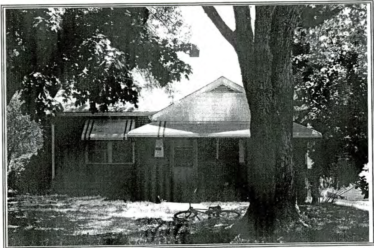
38. House, 161 Maynard Drive
