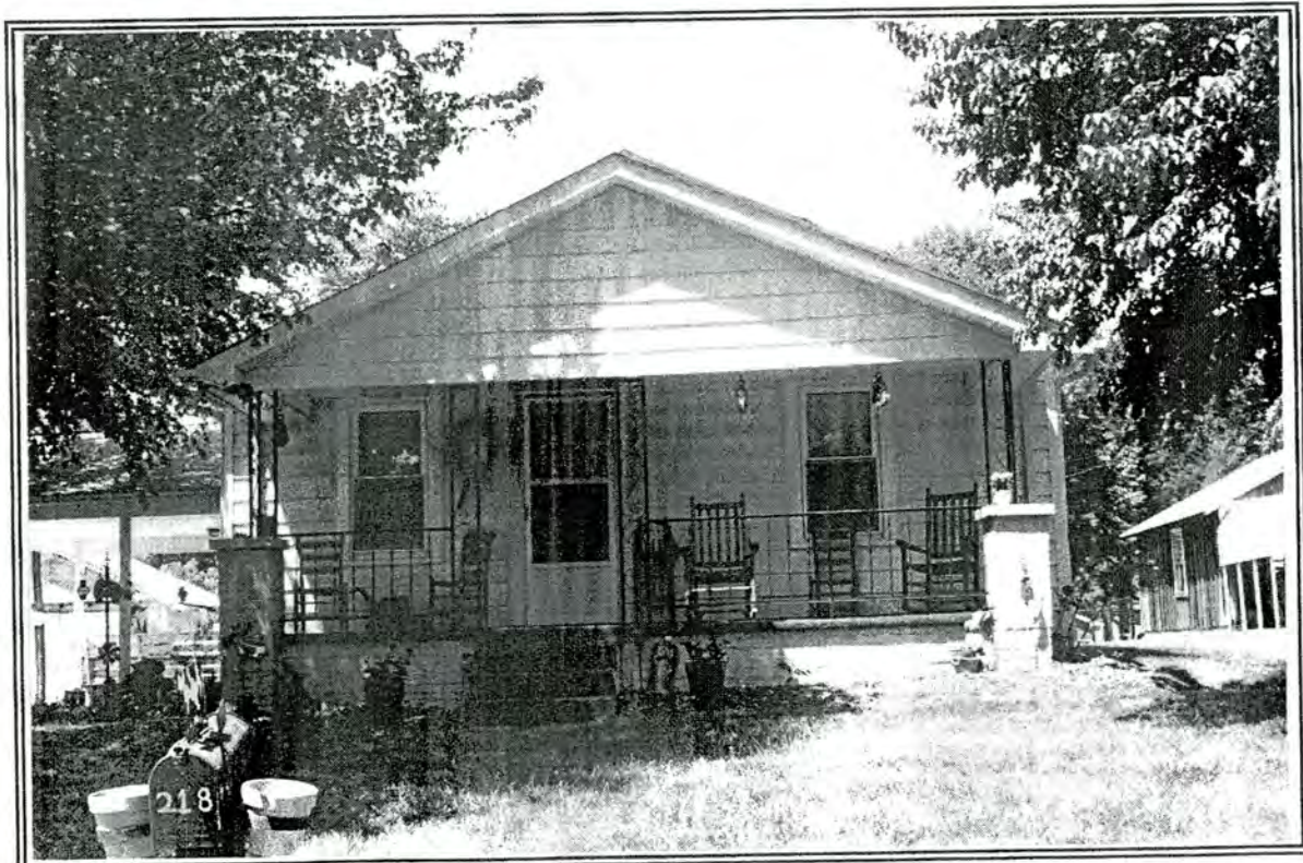
40. House, 218 Maynard Drive
