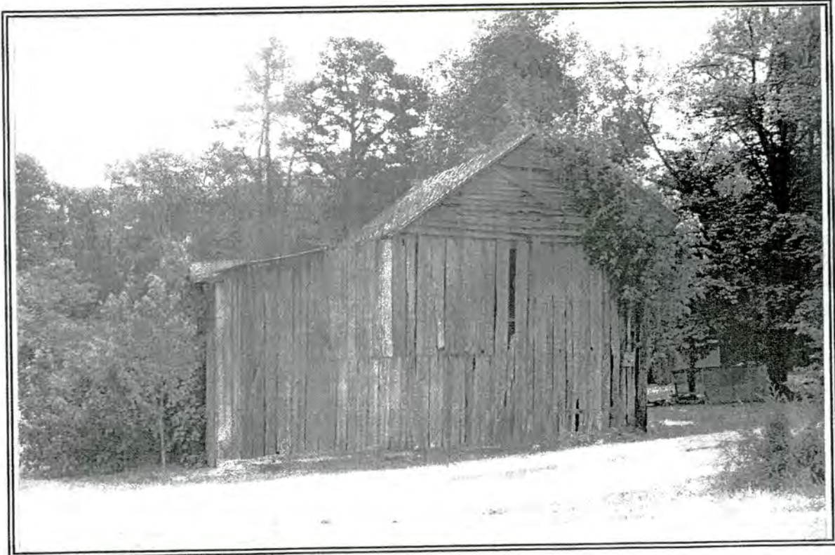
3. Barn, 3811 Hastings Road
