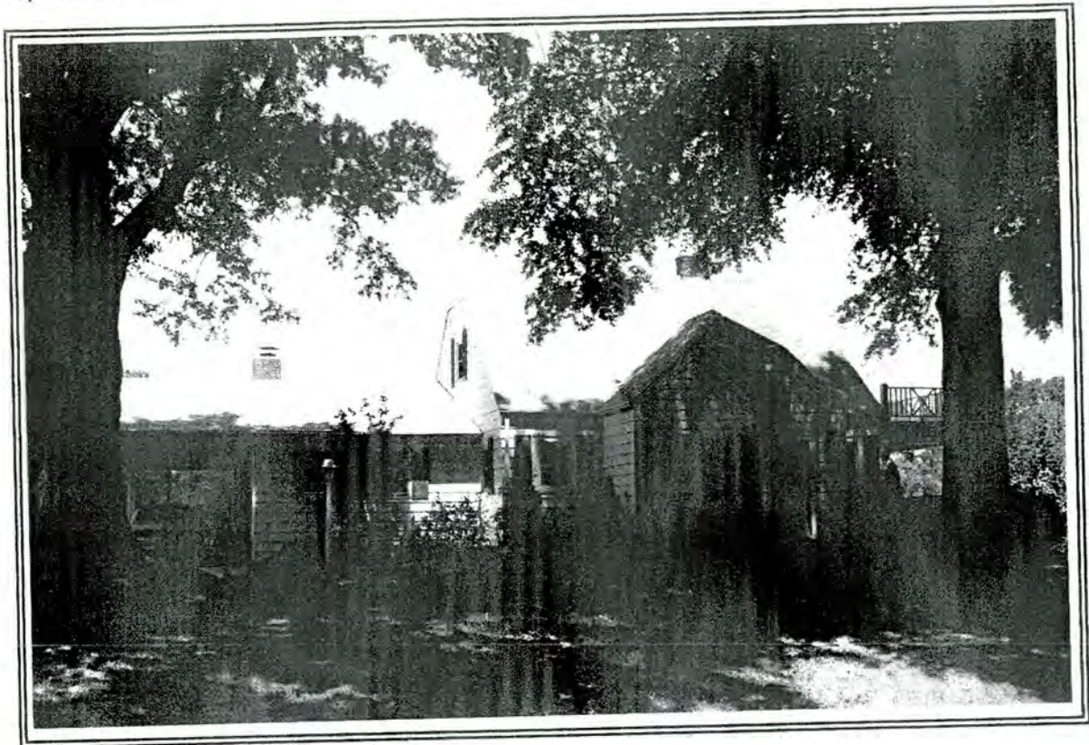
56. House, 4425 Old Winston Road
