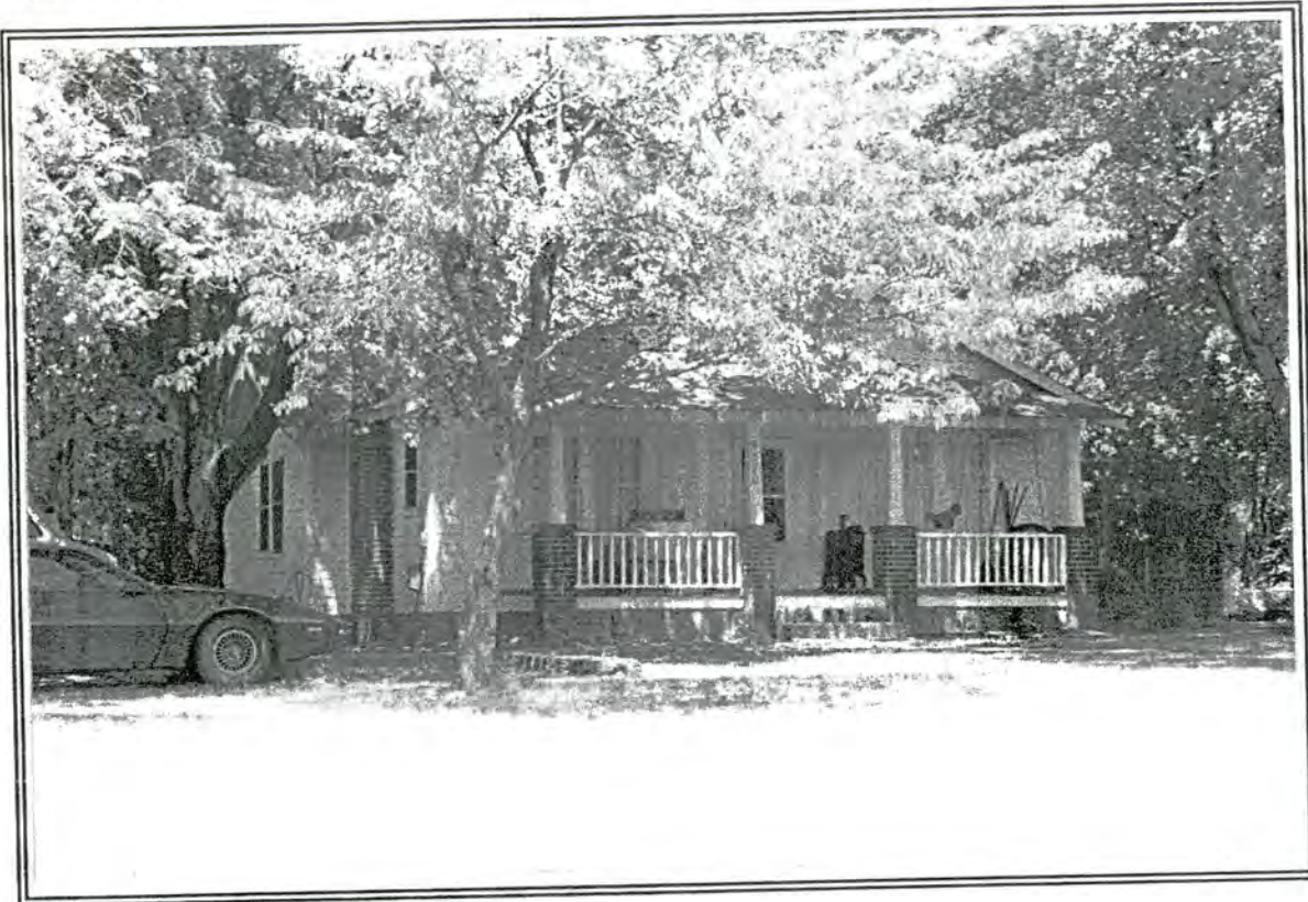
52. House, 4270 Old Winston Road
