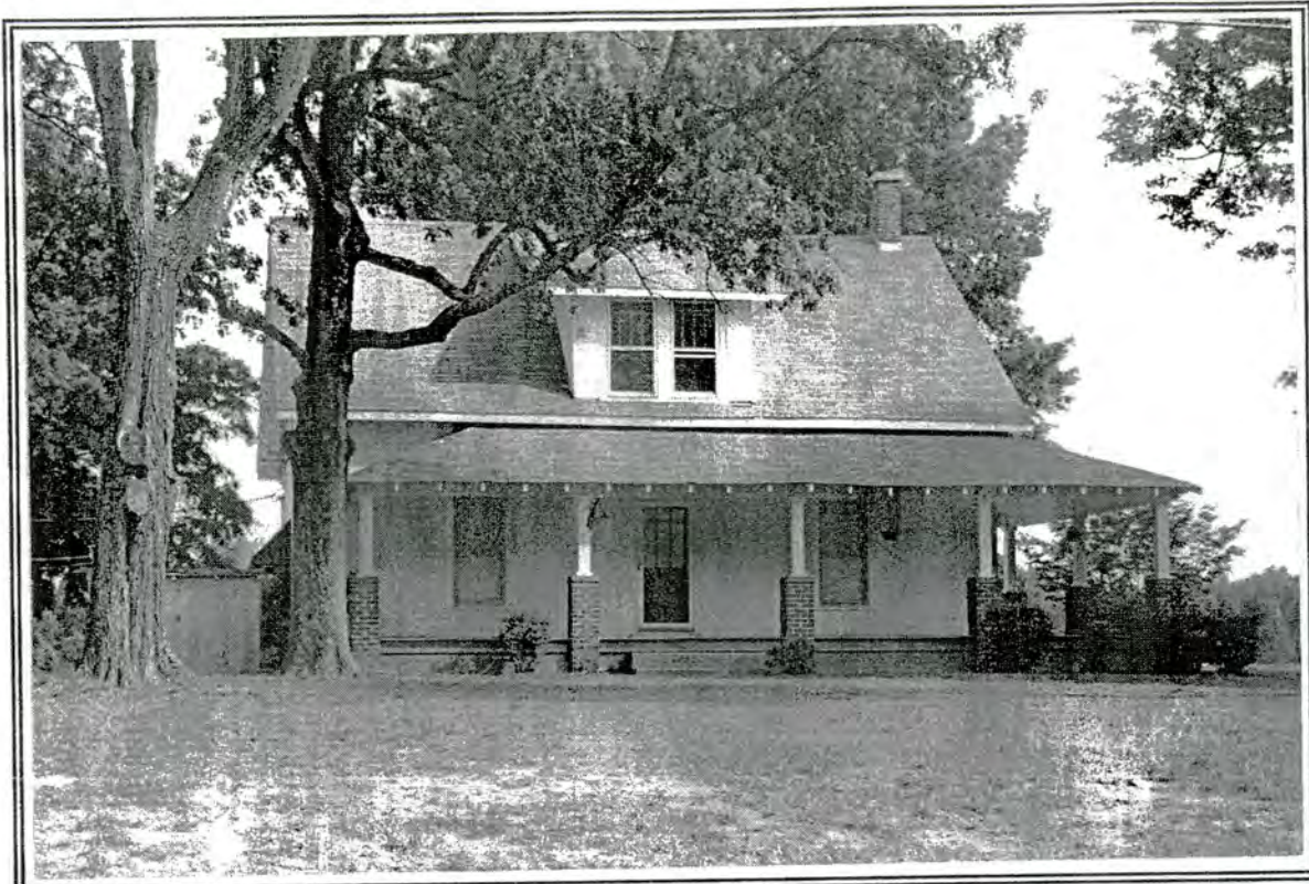
6. House and outbuildings, 1890 Union Cross Road
