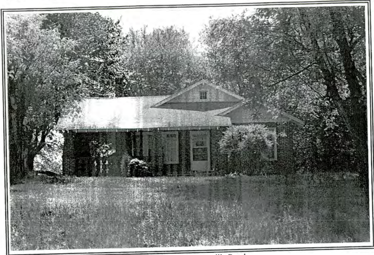
50. House, SW corner, Sedge Garden Road and Kernersville Road
