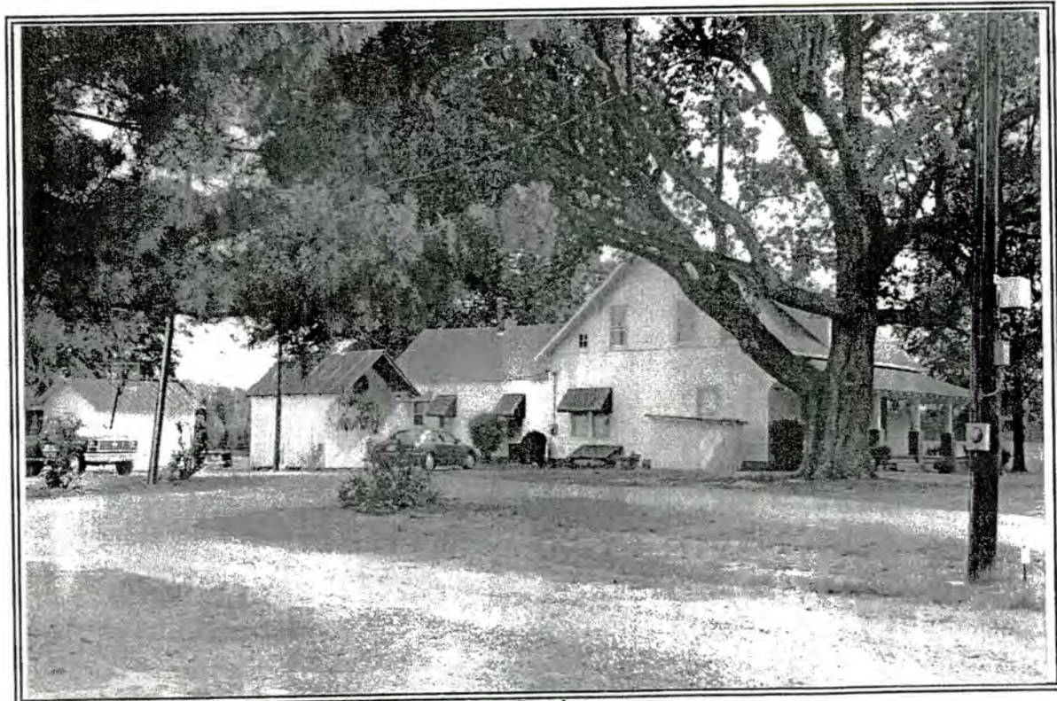
6. House and outbuildings, 1890 Union Cross Road
