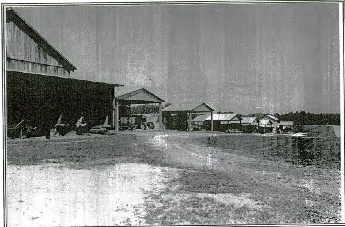
20. House and outbuildings, 4073 Glenn Hi Road
