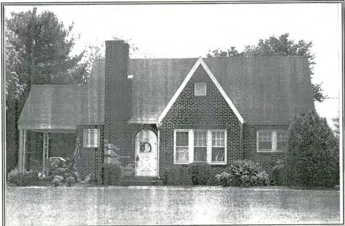
65. House, 4412 Kernersville Road
