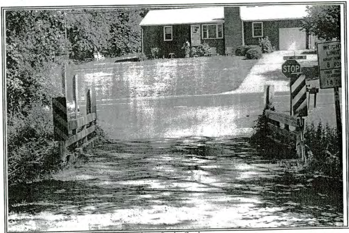
15. Bridge (B6) on Swaim Creek Road over Swaim Creek
