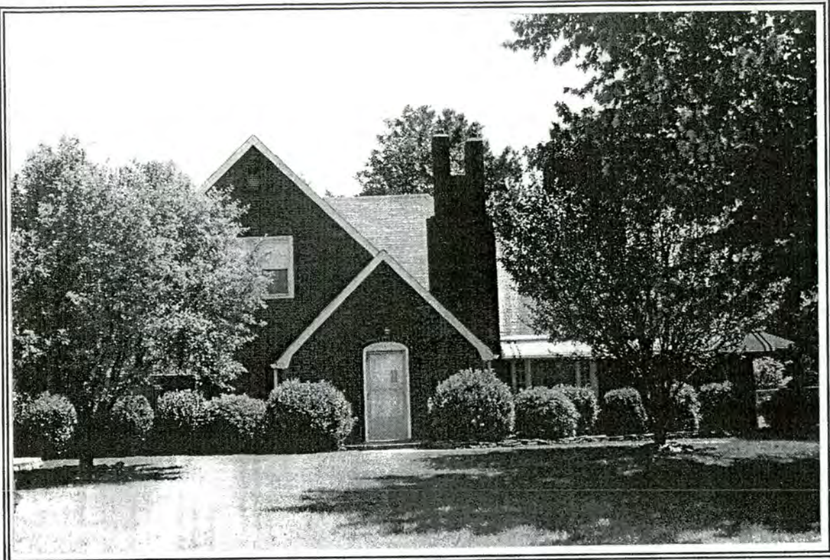
35. House, 117 Maynard Drive
