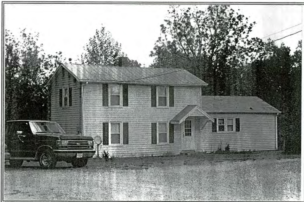
67. House, 459 Hastings Mill Road
