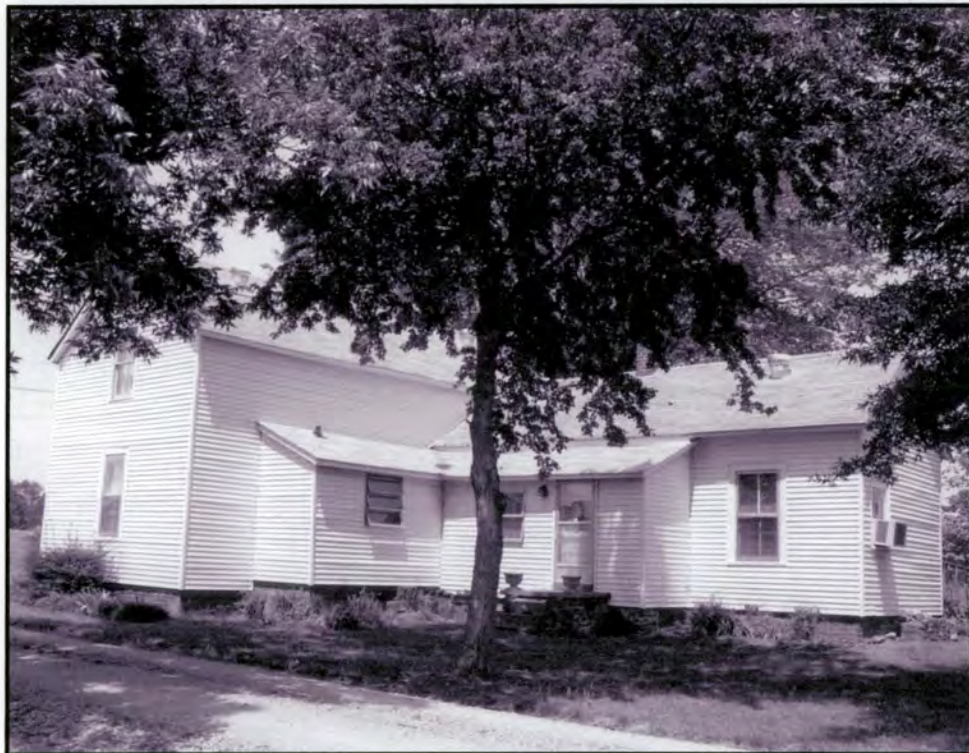
Southwest Corner of House (Facing NE)
