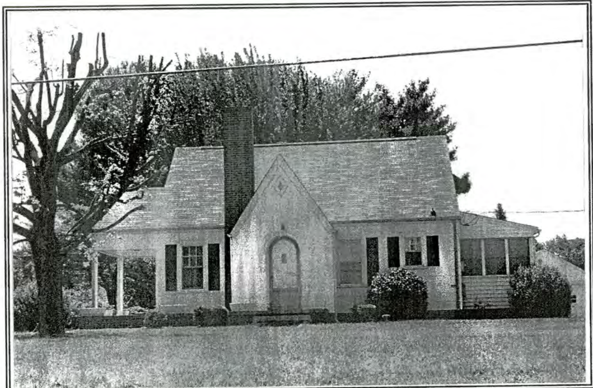
30. House, 4244 Kernersville Road
