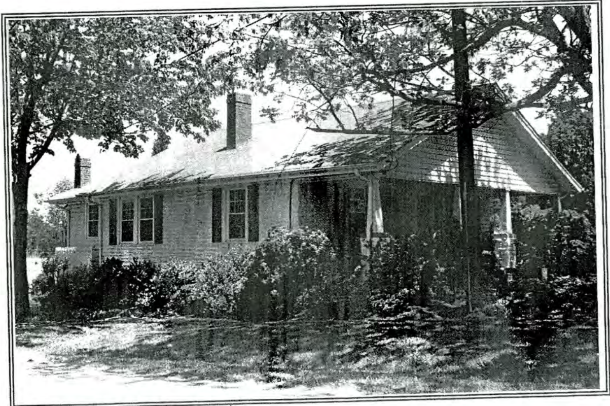
57. House, 4465 Old Winston Road
