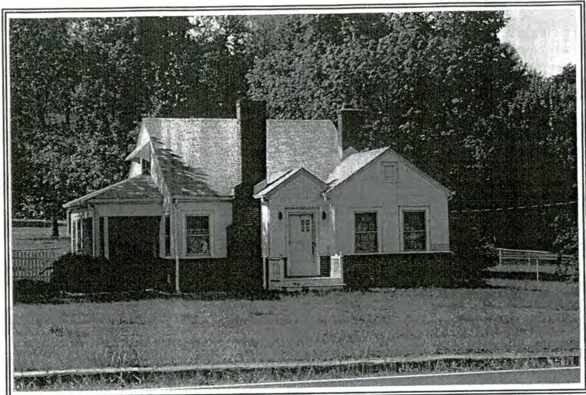
12. House, 4258 High Point Road
