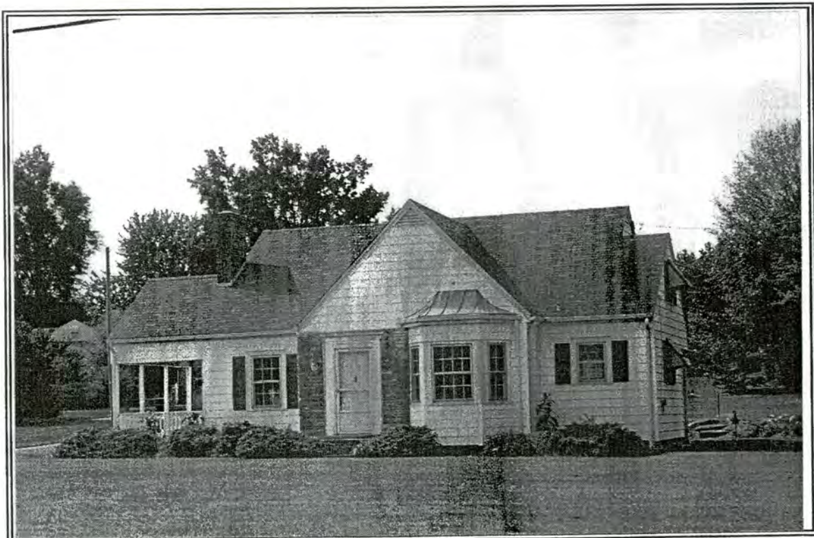
11. House, 4272 High Point Road
