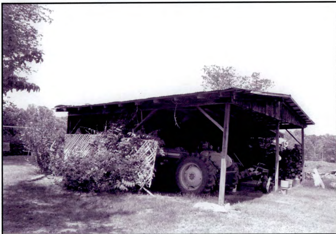
Tractor Shed (Facing ENE)
