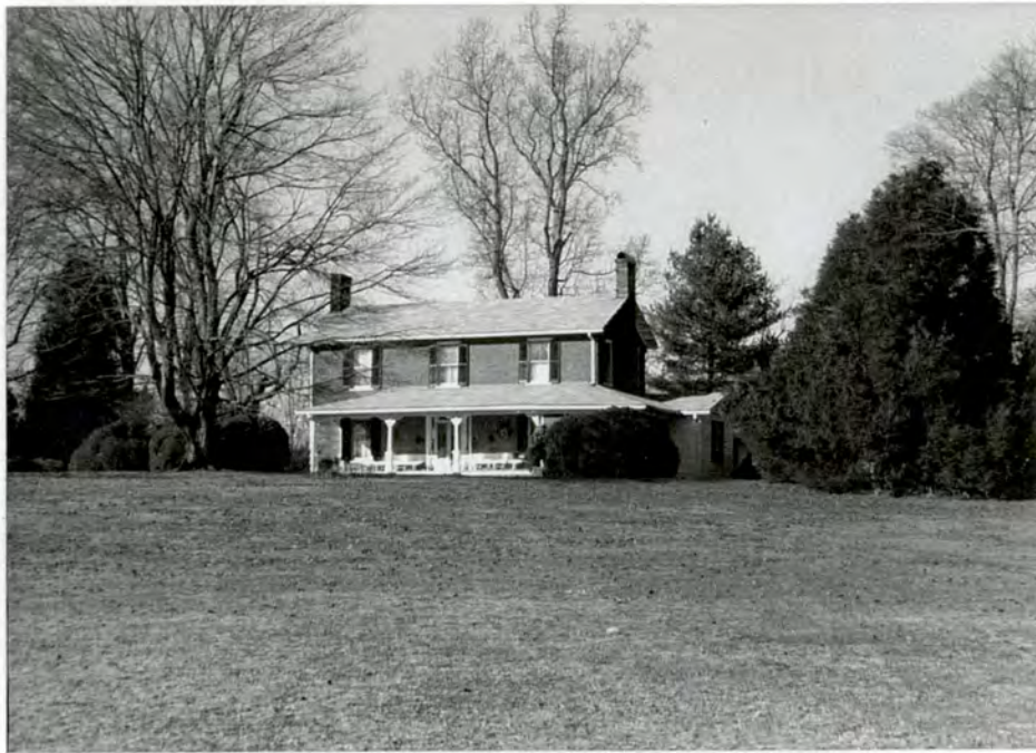
Figure 7: Matthew Clayton Brick House
