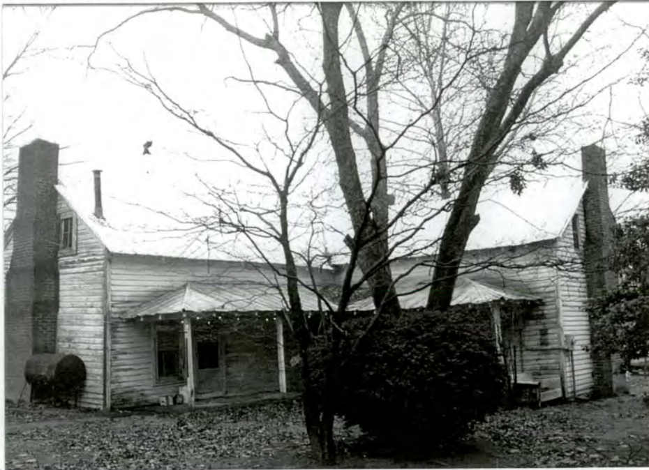
Figure 52. Frank Dillon House
