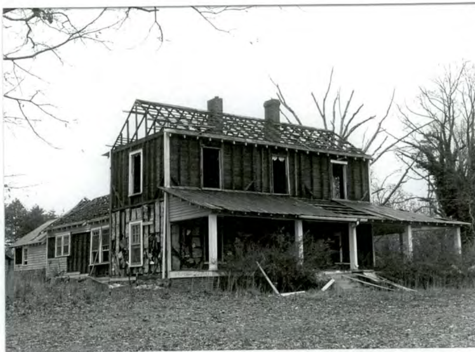
Figure 24. C. C. Stoltz House in process of demolition in 1994
