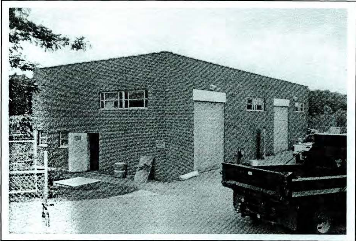
Figure 4.72. Cowans Ford Development; view of warehouse; looking west-northwest.
