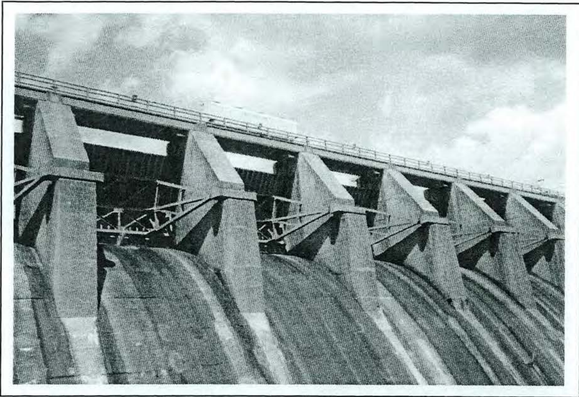
Figure 4.64. Cowans Ford Development; view of spillway gates; looking north-northeast.
