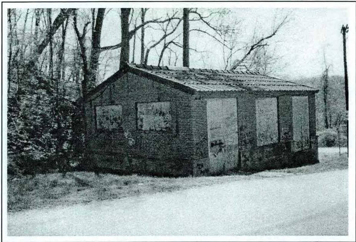
Figure 4.58. Lookout Shoals Development; view of warehouse; looking south-southwest.
