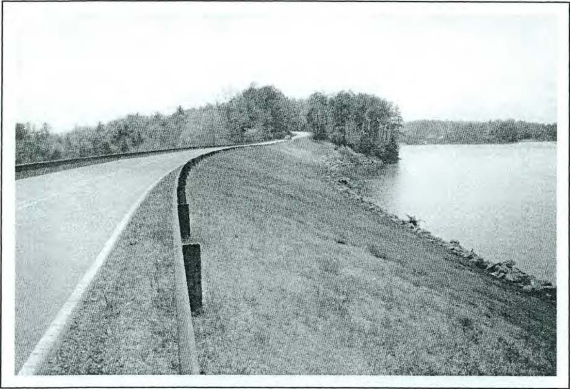
Figure 4.6. Bridgewater Development, Paddy Creek Dam, west side; looking southwest.
