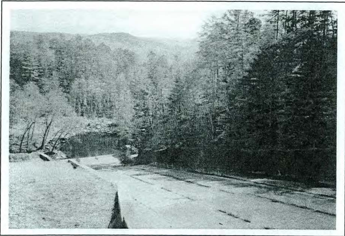
Figure 4.8. Bridgewater Development, Paddy Creek spillway; looking southeast.
