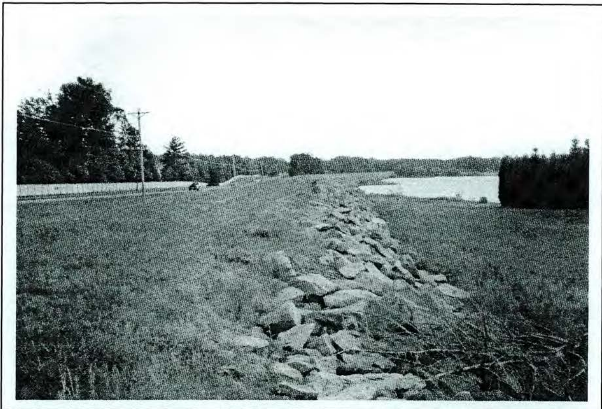
Figure 4.79. Cowans Ford Development; view of Hicks Cross Roads Dike; looking southwest.
