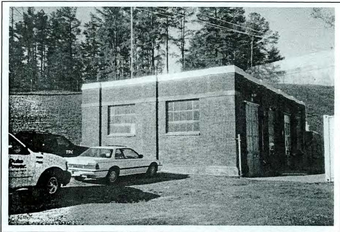
Figure 4.42. Oxford Development; view of warehouse; looking west-southwest.
