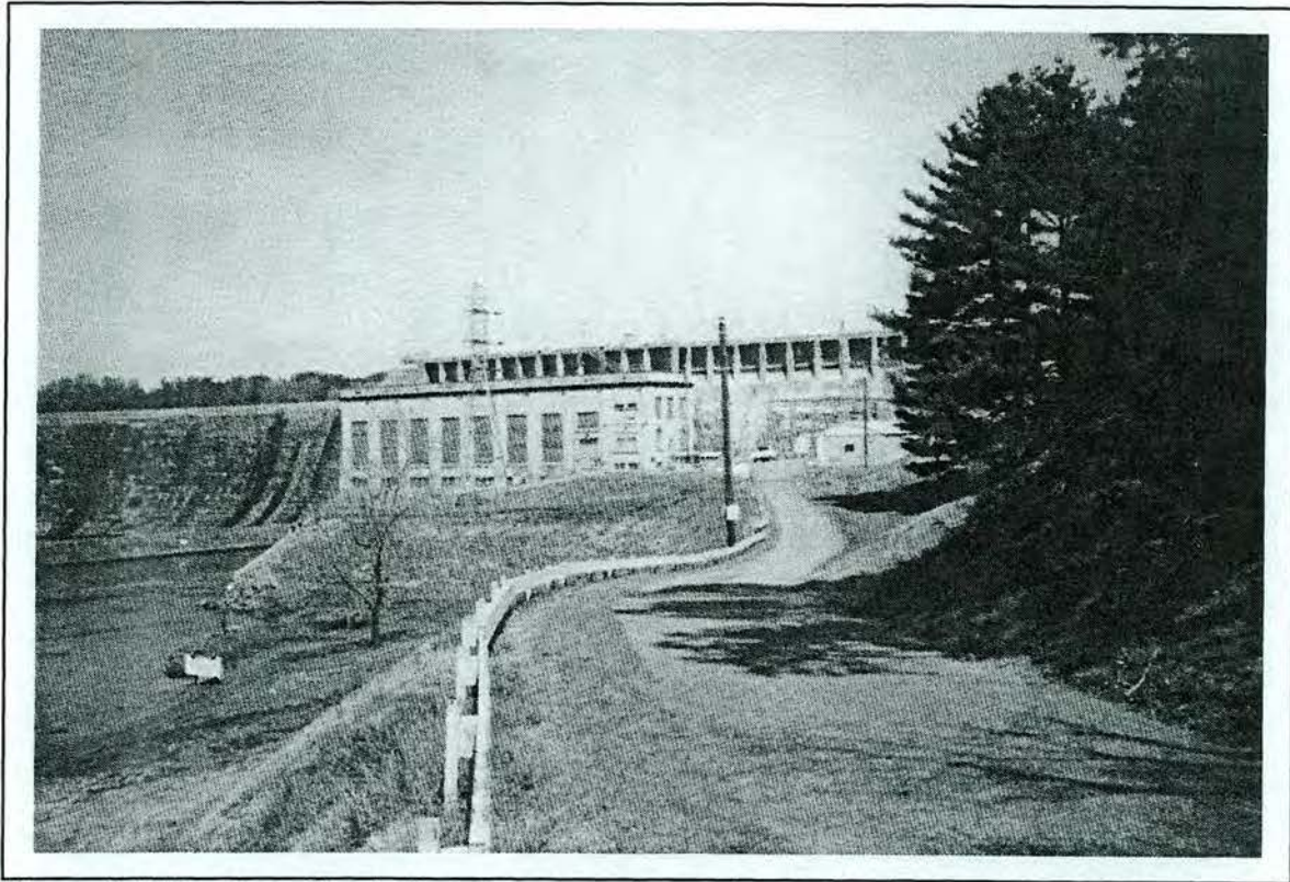
Figure 4.47. Lookout Shoals Development; view of dam, powerhouse, substation, and prefabricated building; looking northwest.
