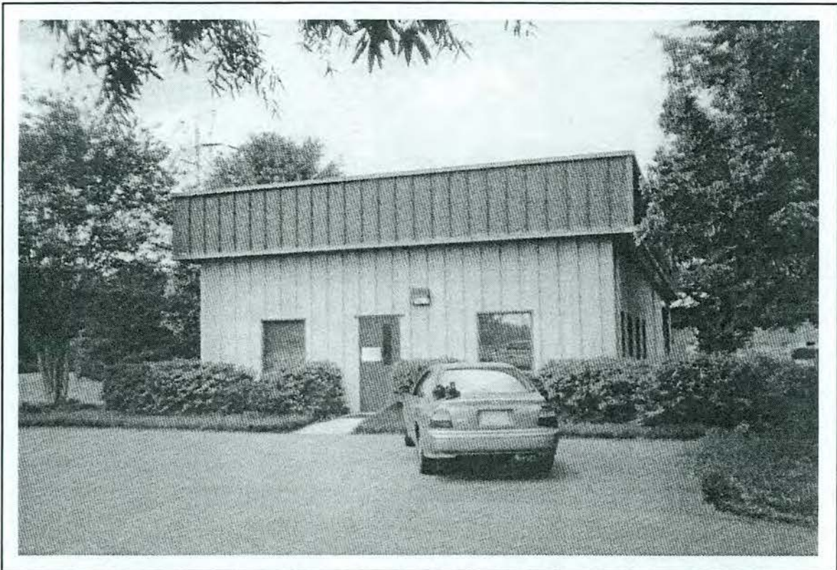
Figure 4.71. Cowans Ford Development; view of office building; looking northwest.
