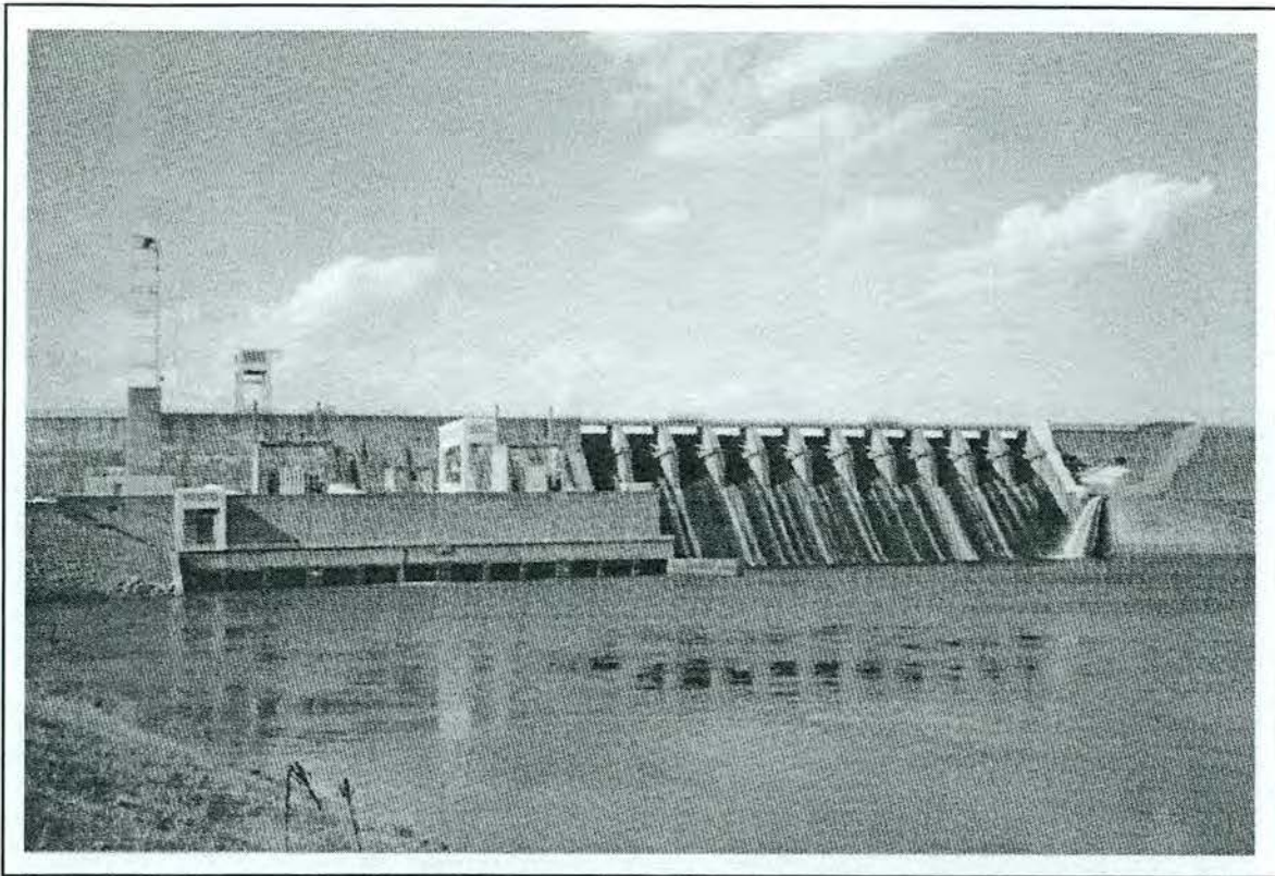
Figure 4.62. Cowans Ford Development; view of dam, powerhouse, and spillway; looking north-northeast.
