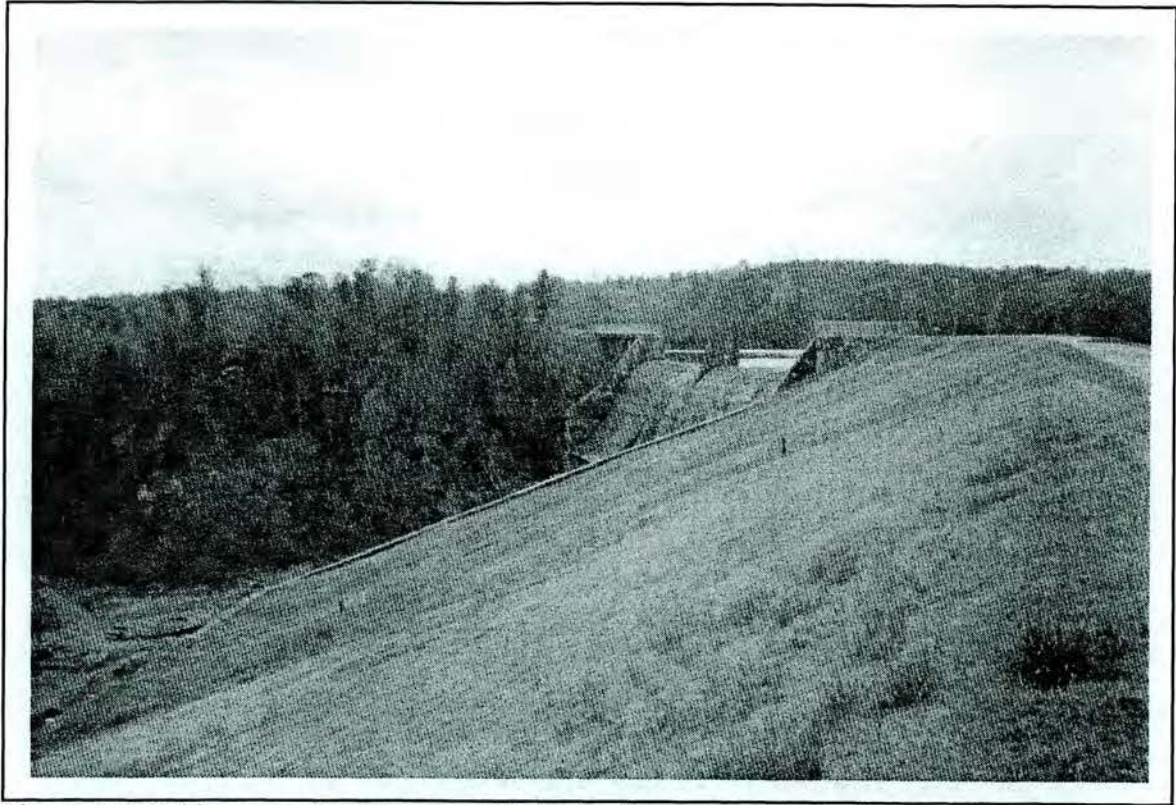
Figure 4.4. Bridgewater Development, Catawba Dam, east side; looking southwest.
