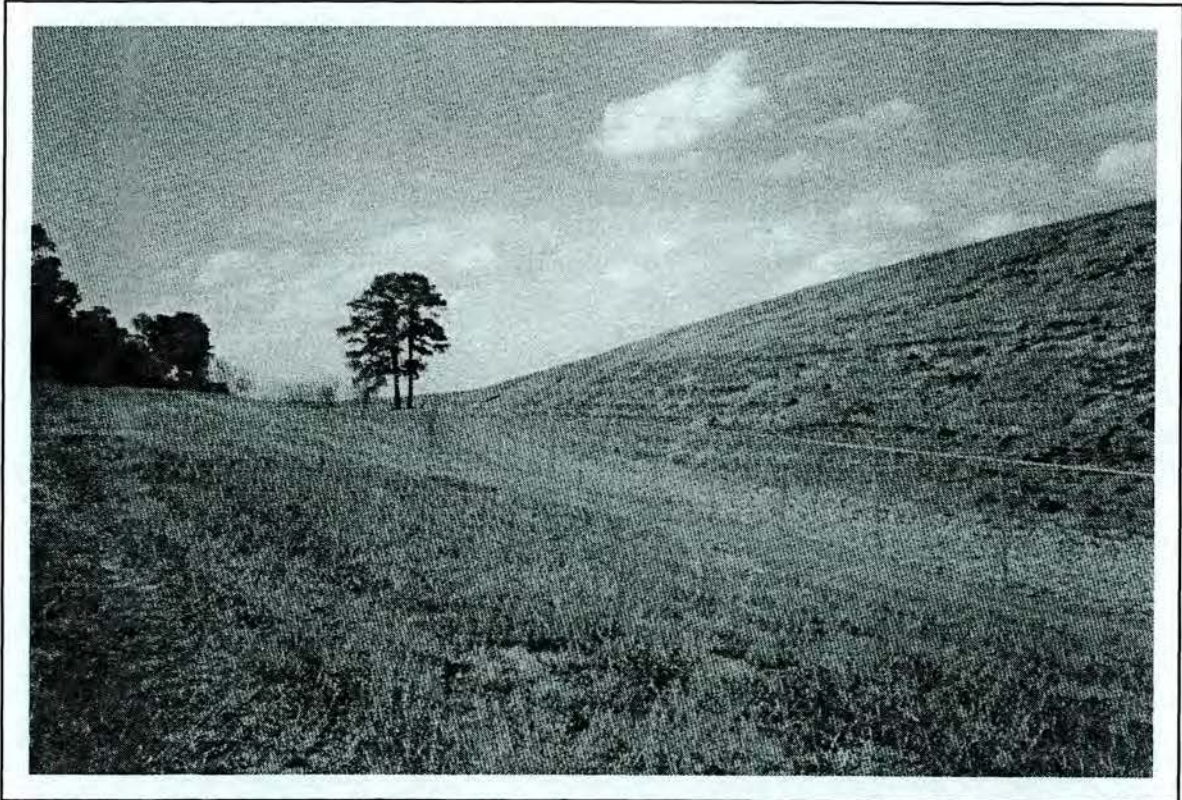
Figure 4.78. Cowans Ford Development; view of west embankment; looking north-northeast.
