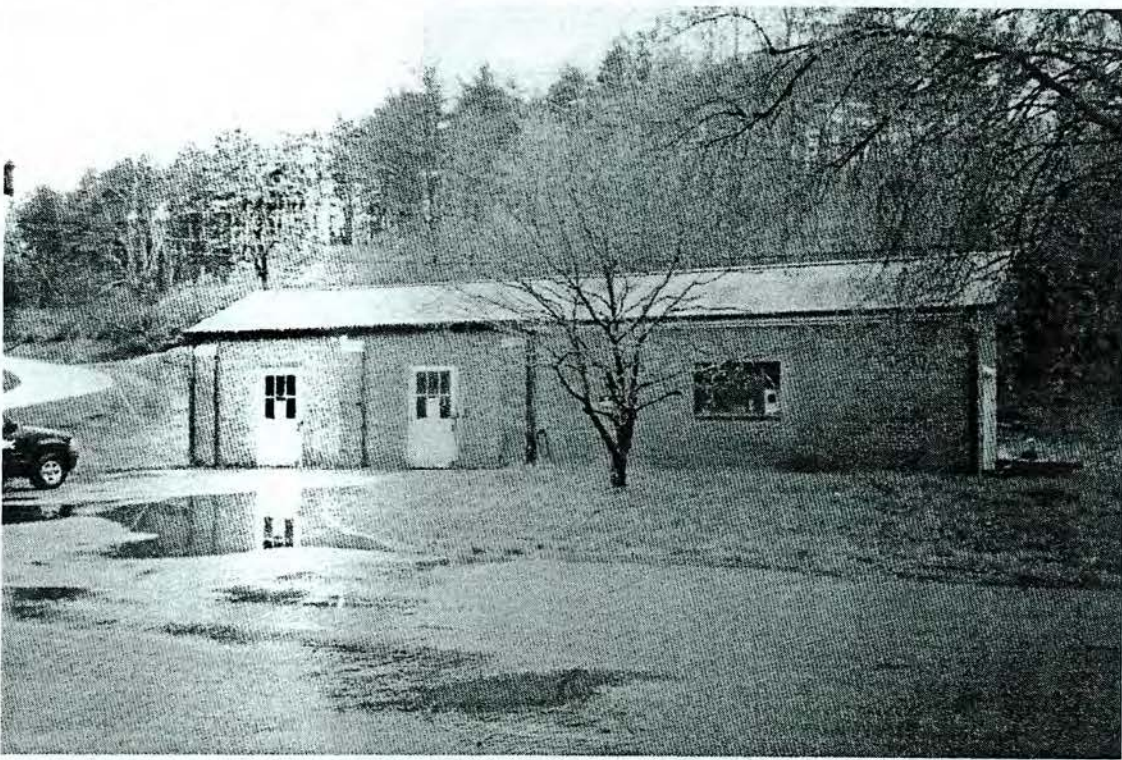
Figure 4.19. Bridgewater Development, Linville Powerhouse; view of warehouse; looking west.
