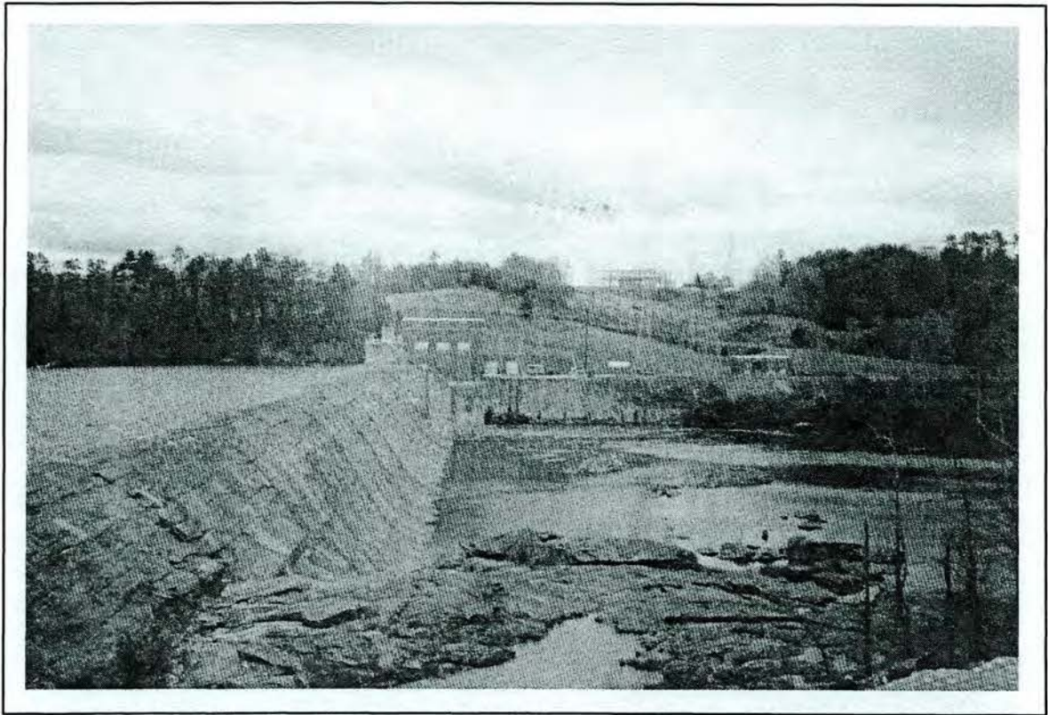
Figure 4.25. Rhodhiss Development; view of dam, powerhouse, substation, and warehouse; looking north.
