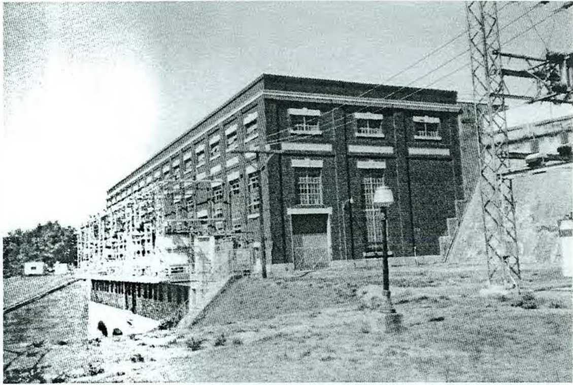
Figure 4.84. Mountain Island Development; Mountain Island Powerhouse; looking west.
