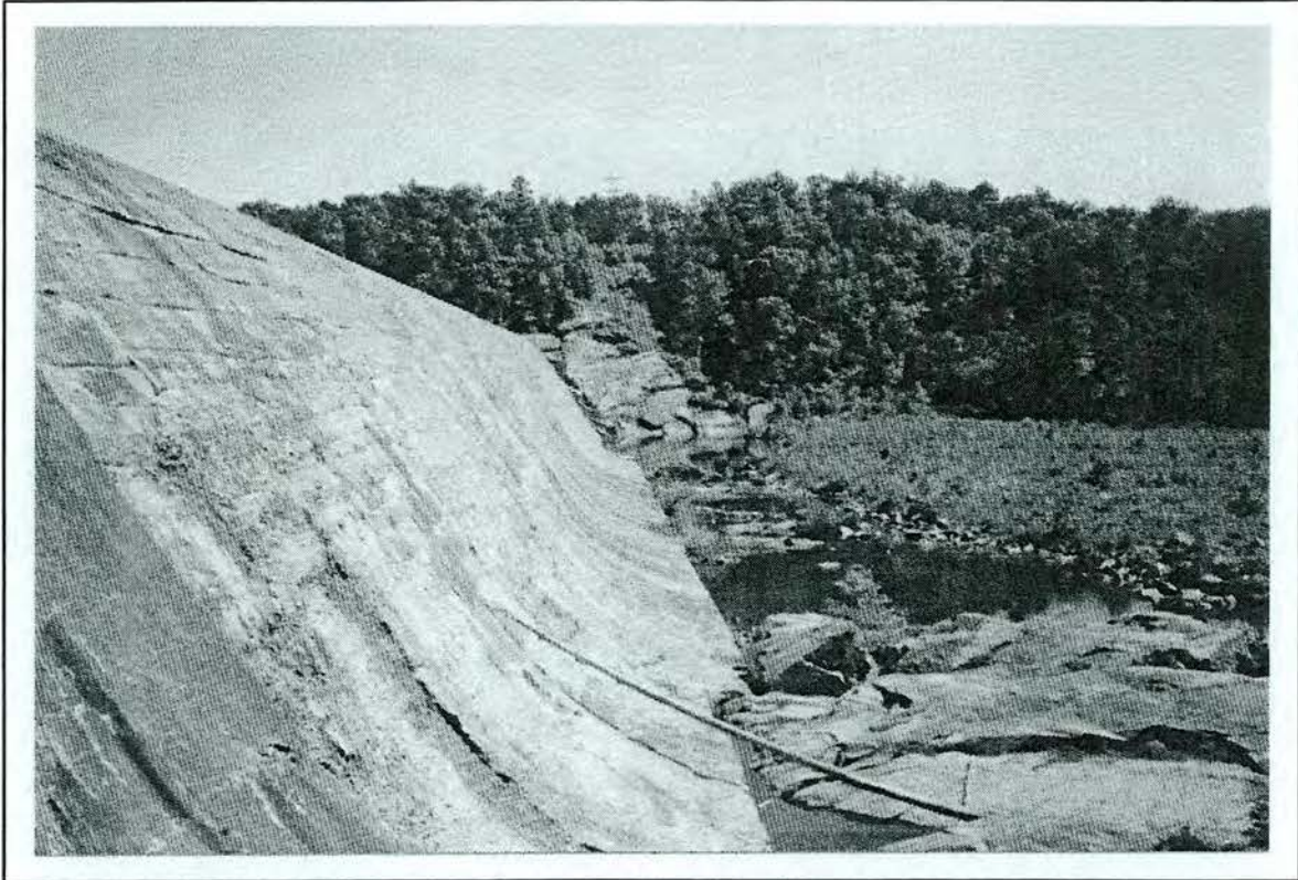
Figure 4.86. Mountain Island Development; view of spillway; looking northeast.
