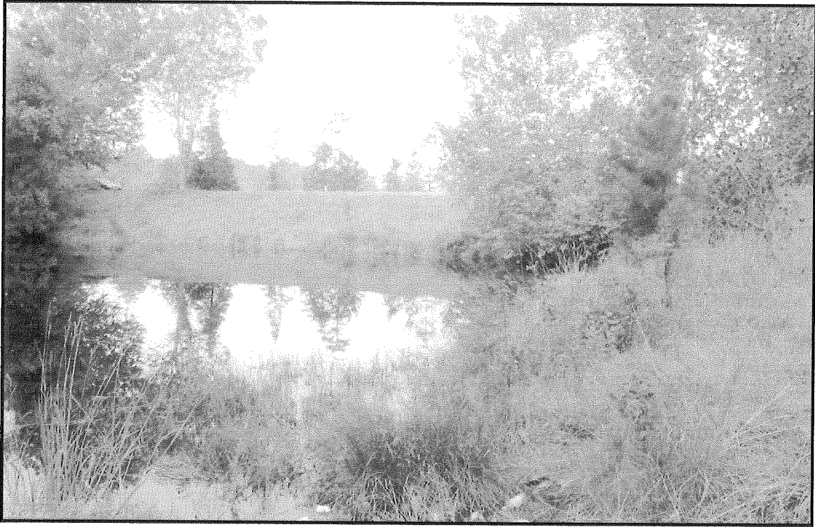
Figure 14. Earth embankment impounding pond at X-Way. View to southwest.
