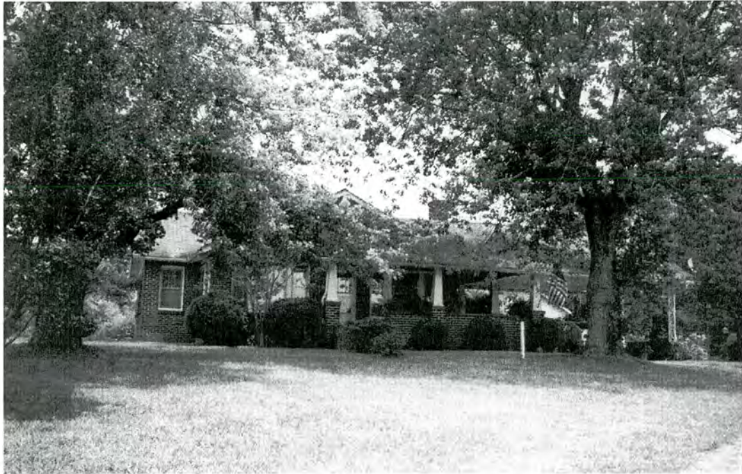
Figure 39. Property No. 25. House. The property has been determined not eligible for the National Register because it is neither historically nor architecturally significant. Photographed July 21, 2003.
