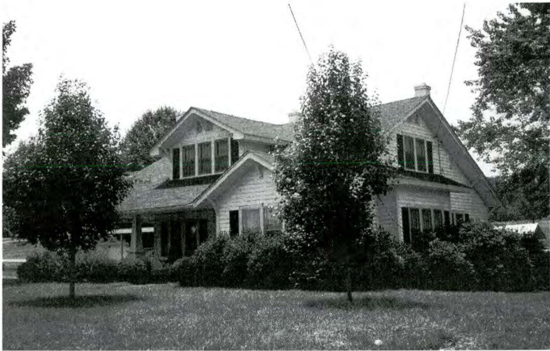
Figure 31. Property No. 17 - House. The property has been determined not eligible for the National Register because it is neither historically nor architecturally significant. Photographed July 21, 2003.
