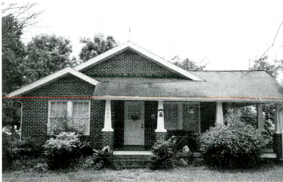
Figure 77. Property No. 62 - House. The property has been determined not eligible for the National Register because it is neither historically nor architecturally significant. Photographed July 21, 2003.
