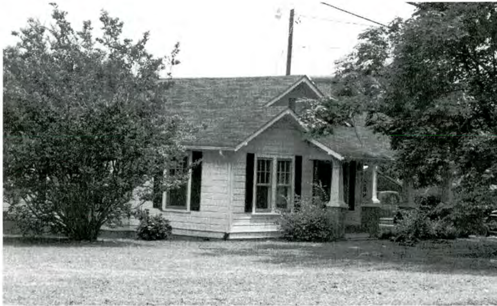
Figure 65. Property No. 51 - House. The property has been determined not eligible for the National Register because it is neither historically nor architecturally significant. Photographed July 21, 2003.
