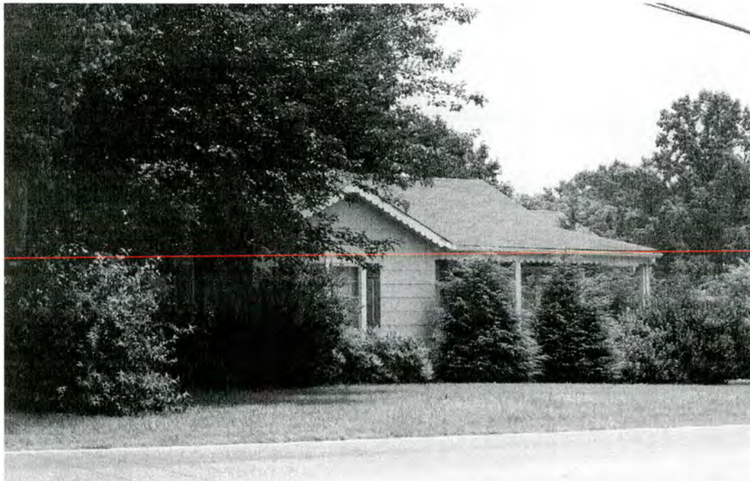
Figure 42. Property No. 28. House. The property has been determined not eligible for the National Register because it is neither historically nor architecturally significant. Photographed July 21, 2003.
