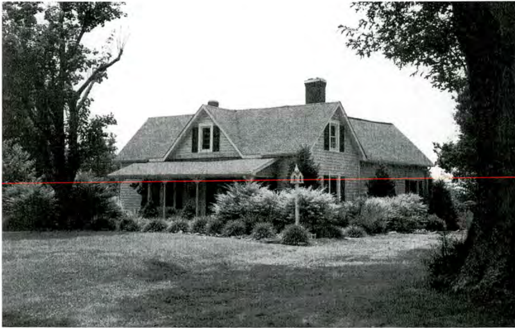
Figure 60. Property No. 46 - House. The property has been determined not eligible for the National Register because it is neither historically nor architecturally significant. Photographed July 21, 2003.
