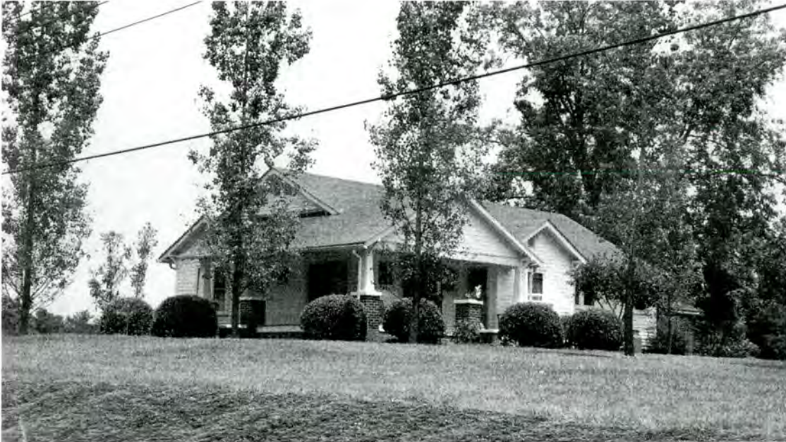
Figure 30. Property No. 16 - House and Barn. The property has been determined not eligible for the National Register because it is neither historically nor architecturally significant. Photographed July 21, 2003.
