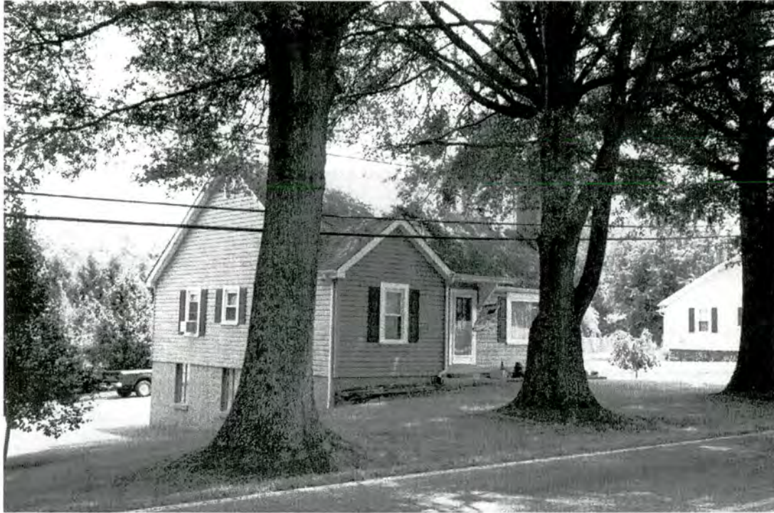
Figure 47. Property No. 33 - House. The property has been determined not eligible for the National Register because it is neither historically nor architecturally significant. Photographed July 21, 2003.
