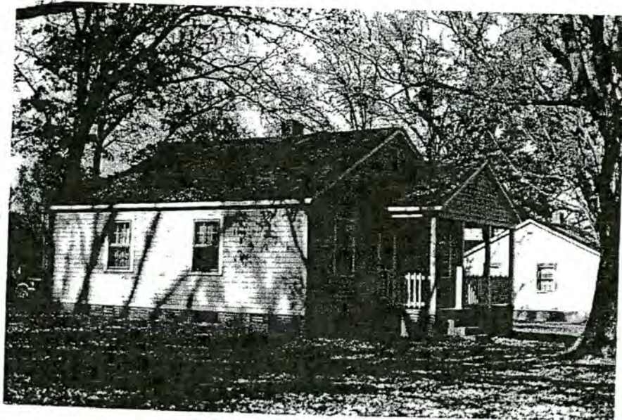
Plate 18. B.H.H.D., Recommended Boundary Expansion, Staff Cottages South of I-40, Gable-Front Model, Looking North Along Enola Road.
