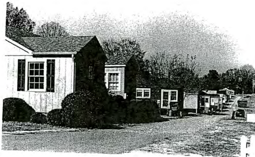
Plate 20. B.H.H.D., Recommended Boundary Expansion, Staff Cottages South of I-40, Rear Elevations, Looking North Along East Side Of Enola Road.
