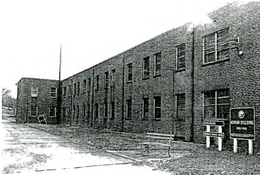
Plate 9. B.H.H.D., Recommended Boundary Expansion, Moran Building, East Elevation, Looking North.
