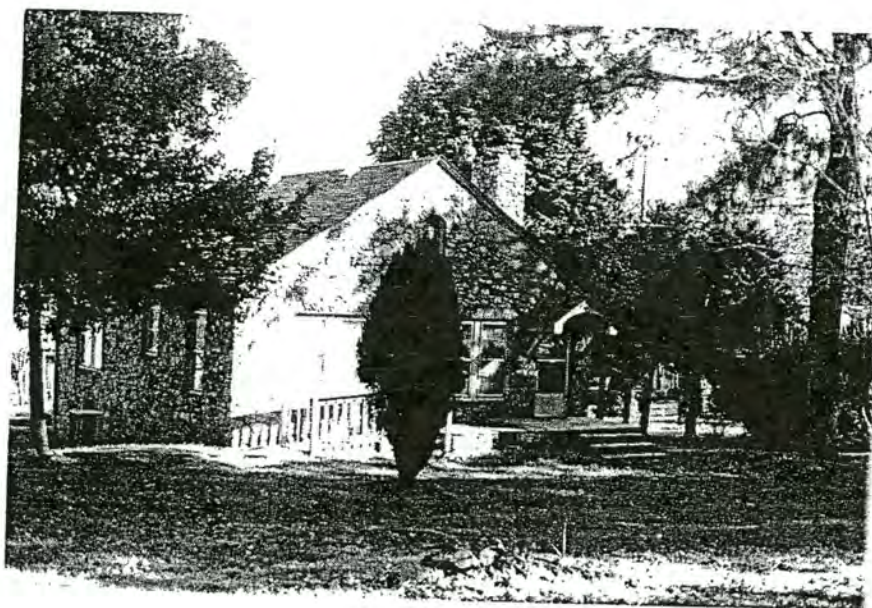
Plate 41. Mull's Store and House, House Facade and North Elevation, Looking Southeast.
