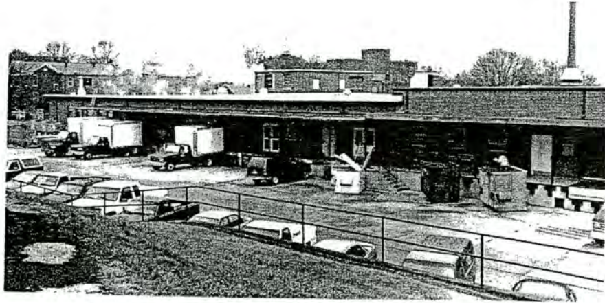
Plate 7. B.H.H.D., Recommended Boundary Expansion, Hooper Building, South Elevation, Looking North.
