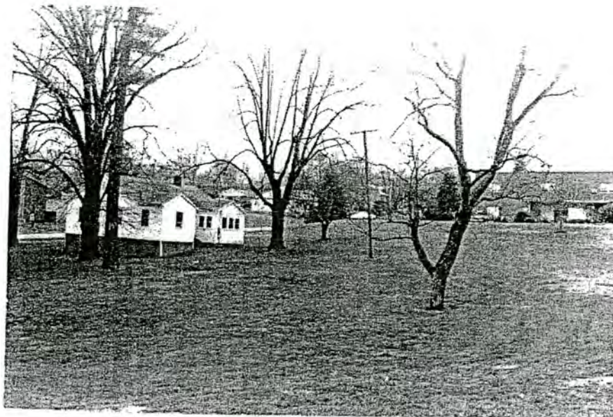
Plate 12. B.H.H.D., Recommended Boundary Expansion, Staff Cottage, Rear Elevation, Looking South.
