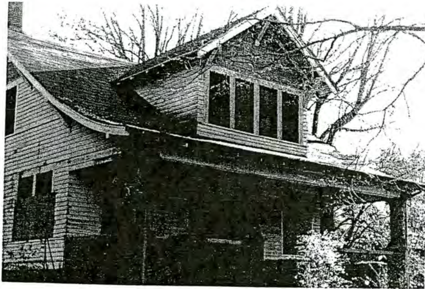
Plate 30. U.S.B. Dale's Market, Dale House, Facade, Looking Southeast.
