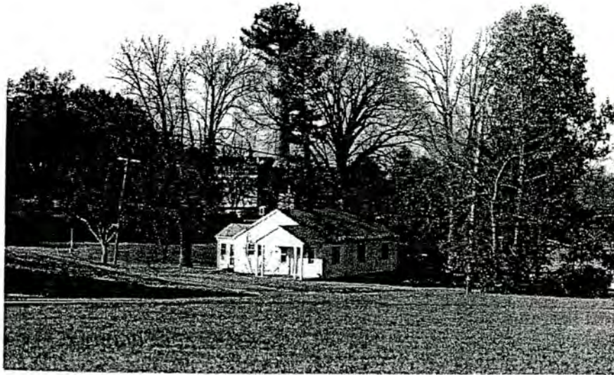
Plate 11. B.H.H.D., Recommended Boundary Expansion, Staff Cottage, Looking North.
