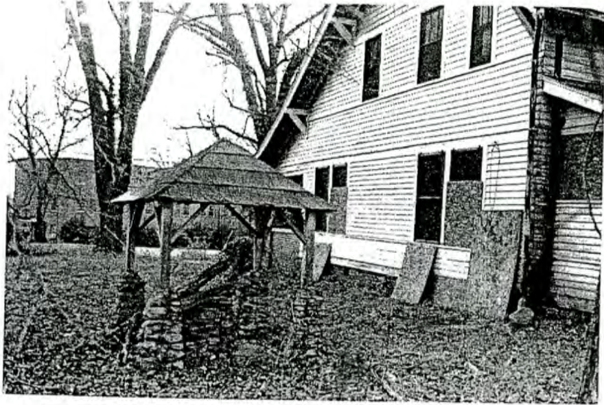
Plate 33. U.S.B. Dale's Market, Dale House, South Elevation and Well, Looking Northwest.
