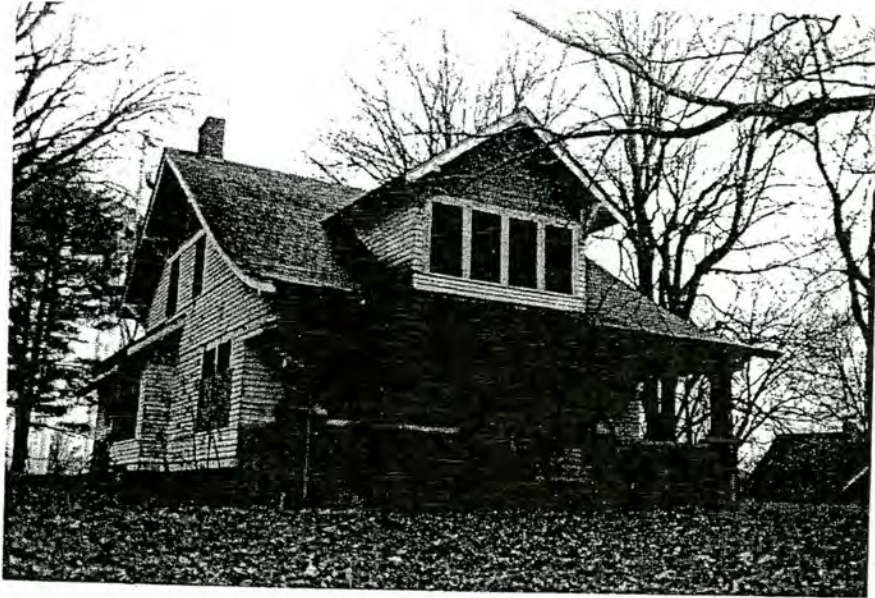
Plate 29. U.S.B. Dale's Market, Dale House, Facade and North Elevation, Looking Southeast.
