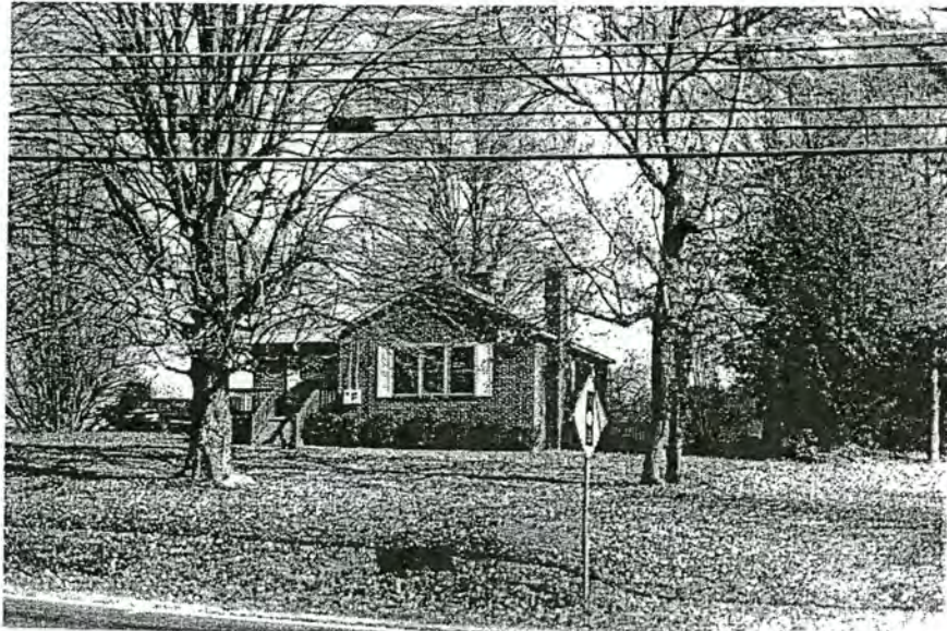
Plate 25. B.H.H.D., Recommended Boundary Expansion, Staff Cottages South of I-40, Mid-Twentieth Century, Brick Dwelling Located Outside District, Looking East.
