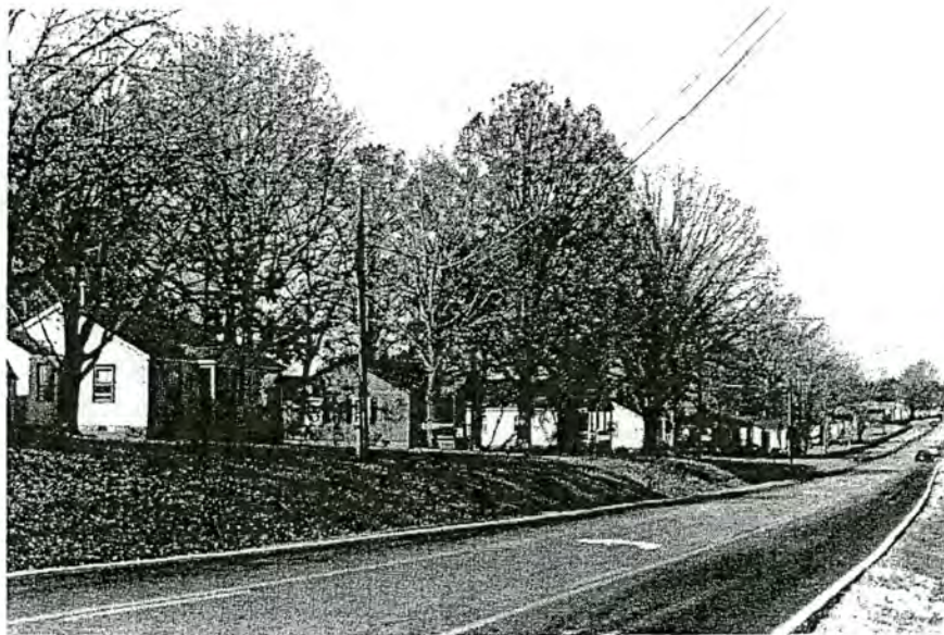
Plate 14. B.H.H.D., Recommended Boundary Expansion, Staff Cottages South of I-40, Looking North Along West Side Of Enola Road.
