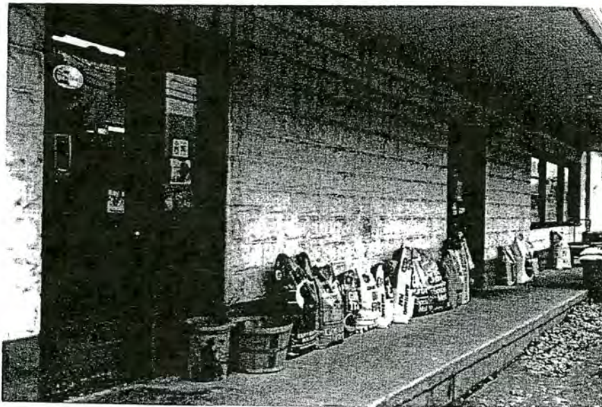
Plate 37. Mull's Store and House, Entrance Detail of Store.
