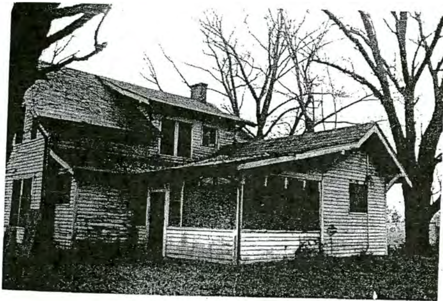
Plate 32. U.S.B. Dale's Market, Dale House, Rear Ell, Looking Northwest.
