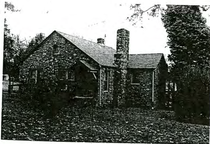
Plate 40. Mull Store and House, Mull House, Facade and South Elevation Looking East.
