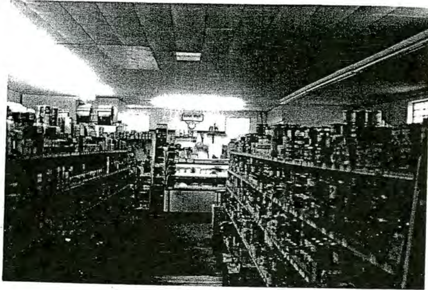
Plate 38. Mull Store and House, Interior of Original Store, Looking North.
