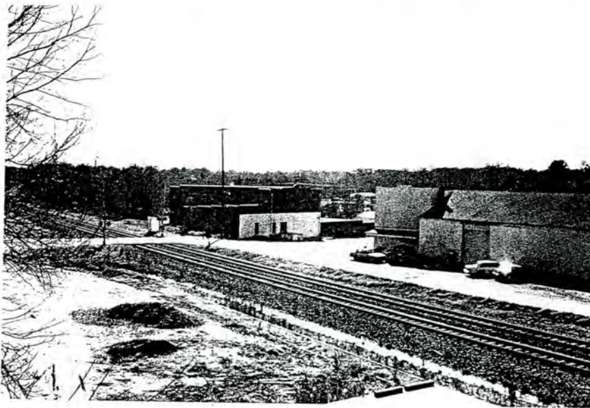
Plate 11. Looking North Towards Bridge No. 266 From Corban Avenue.
