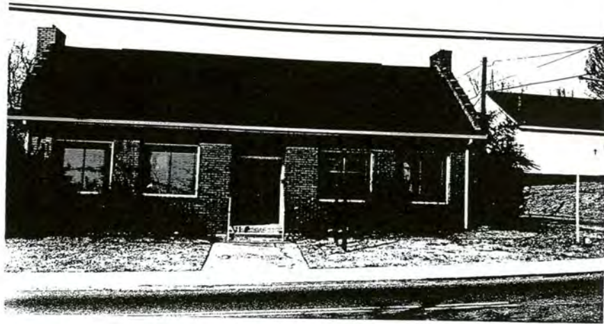
Plate 5. Modern Office Building, Cabarrus Avenue West, North Side.
