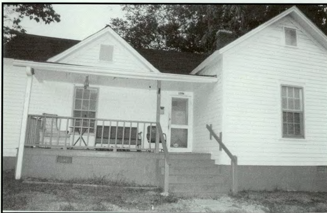
Golden Belt Historic District—House, 1206 Wall Street
