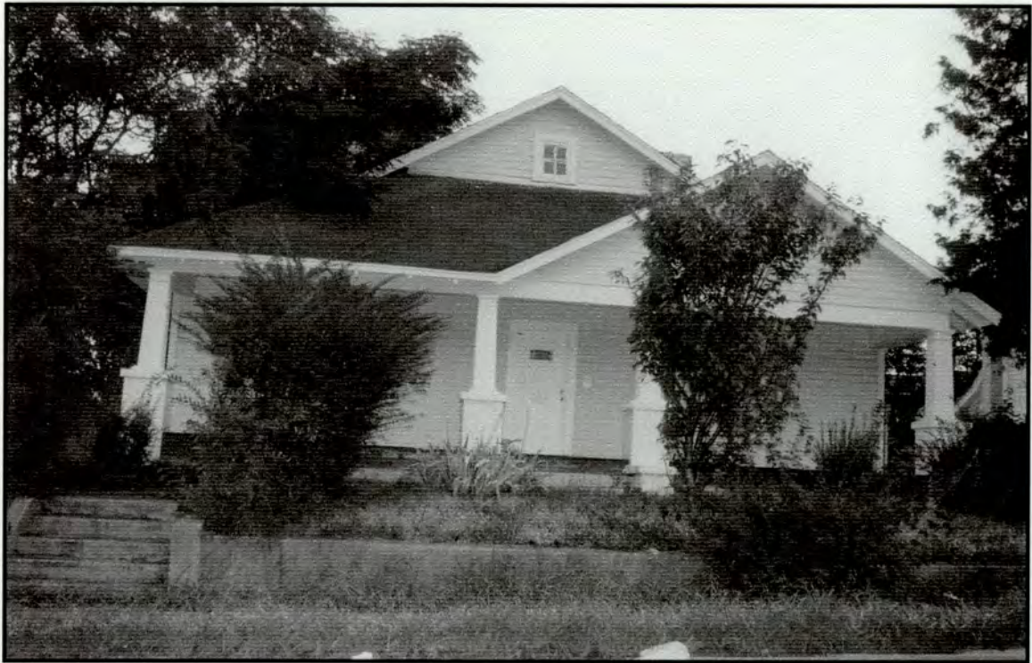
14, 209 South Alston Avenue
