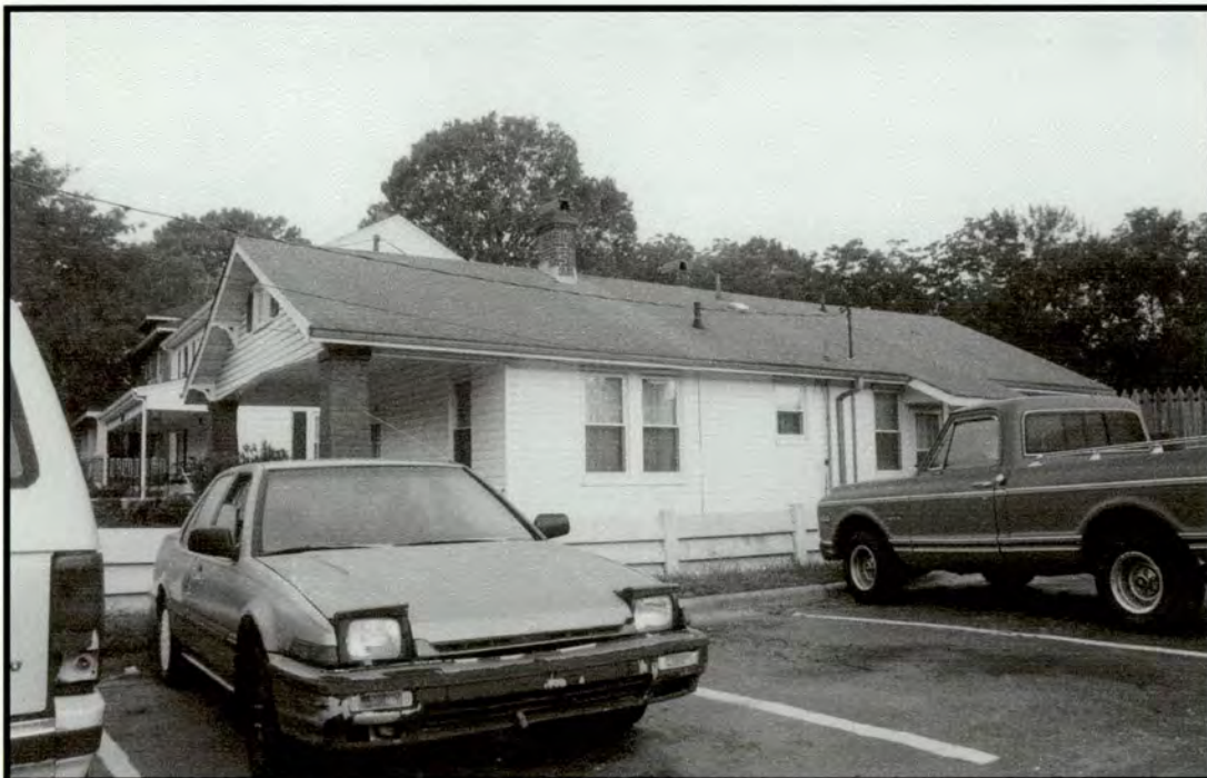
809 Holloway Street (northeasternmost property in Study Listed Holloway Street Historic District boundary expansion)
