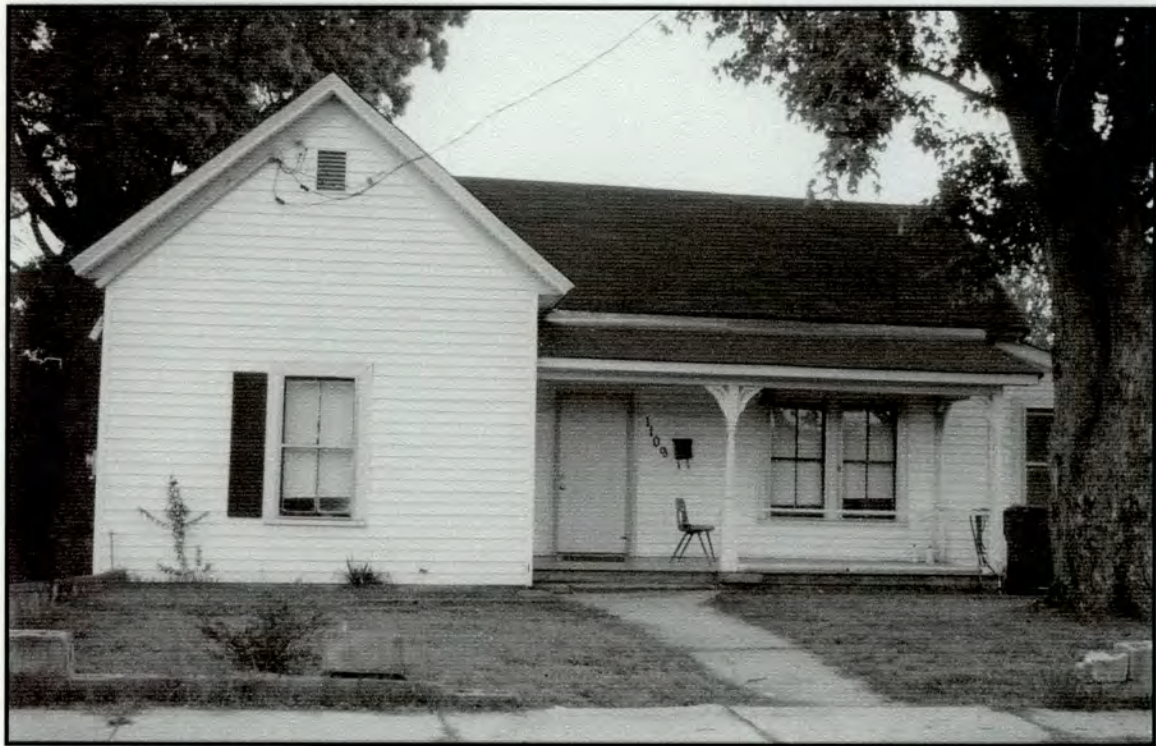
16. House, 1109 Angier Avenue
