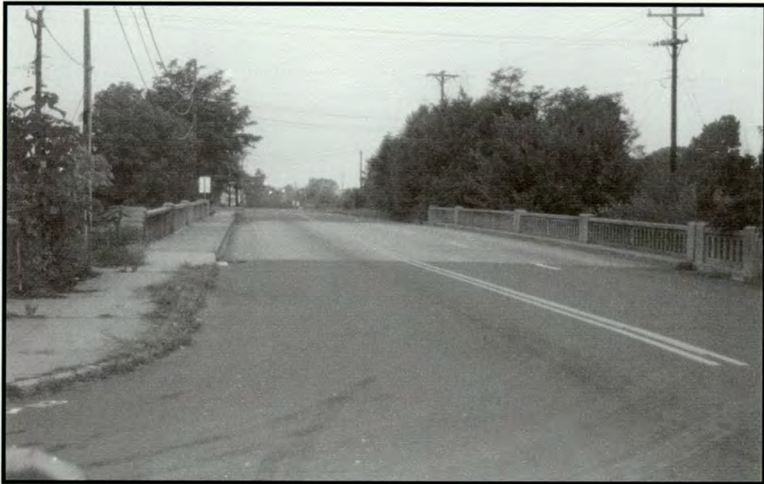
Pettigrew Street Bridge over Alston Avenue
