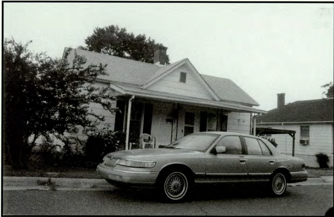
Golden Belt Historic District—House, 1203 Wall Street
