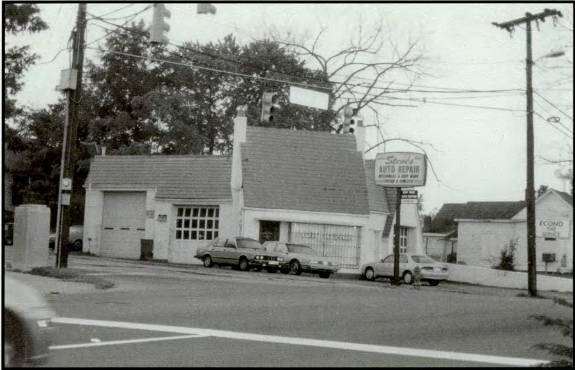
Pure Oil Filling Station, 1200 East Main Street
