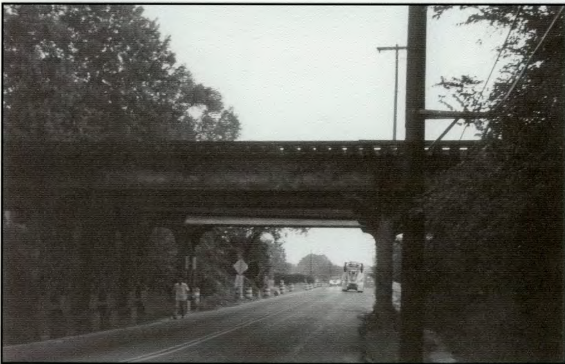
7., 8., and 9. Riveted plate-girder railroad bridges
