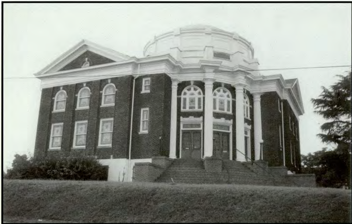
Branson Methodist Church, 201 South Alston Avenue
