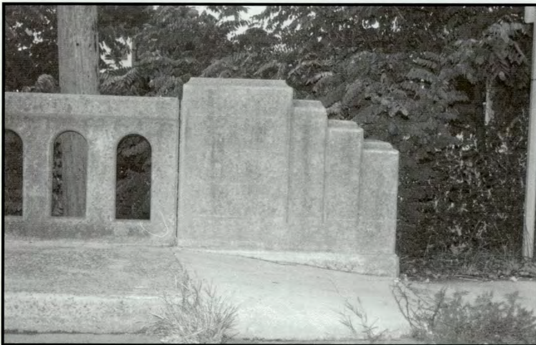
Railing endpost of Pettigrew Street Bridge over Alston Avenue
