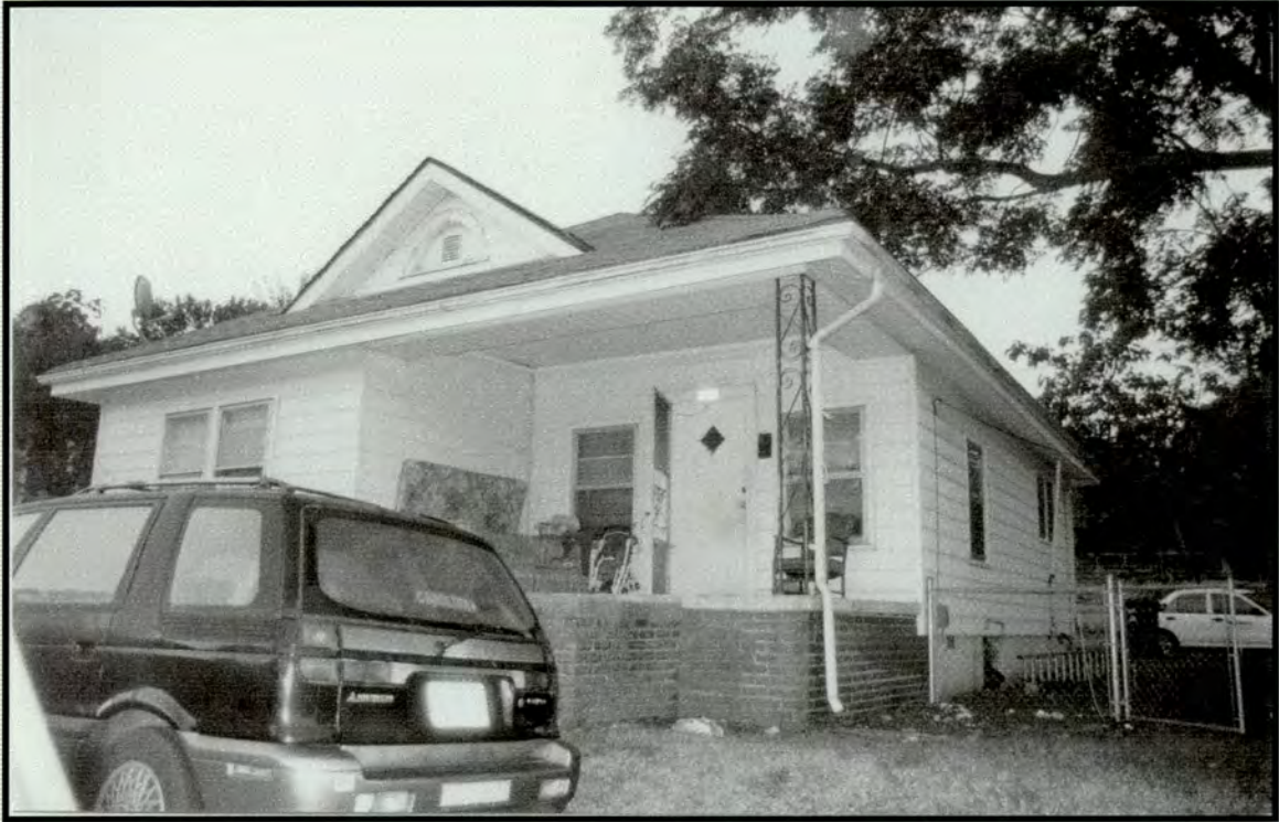
Golden Belt Historic District—House, 1208 Wall Street
