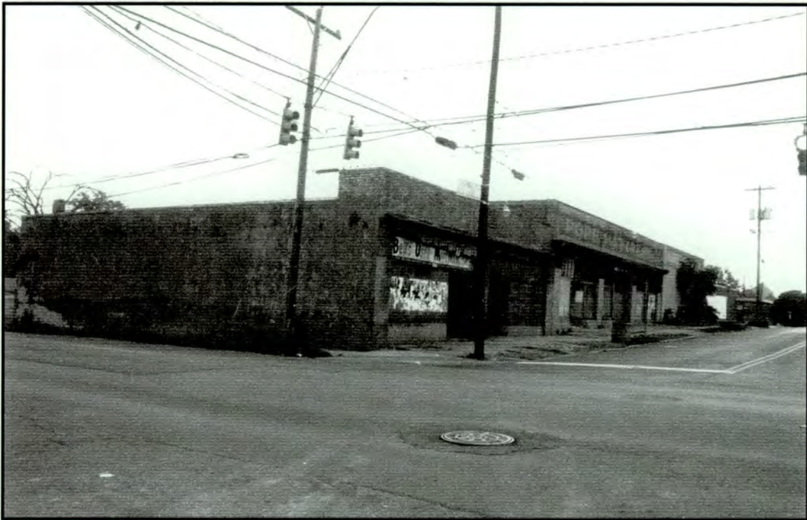
17., 18., 19. Commercial buildings, 1201-1211 Angier Avenue
