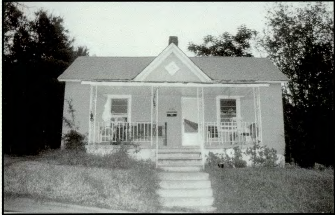
Golden Belt Historic District—House, 1111 Wall Street
