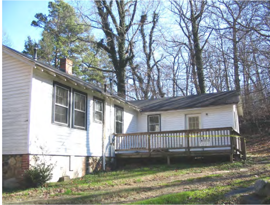
Tenant House, Rear Ell, Jake Long Dairy Barn, Looking East.
