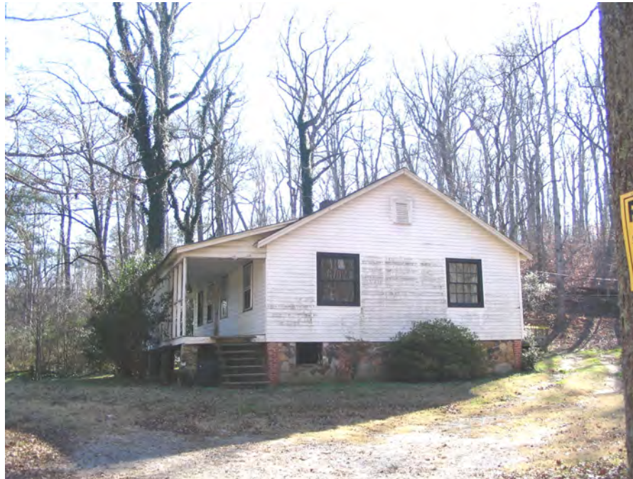
Tenant House, Jake Long Dairy Barn, Looking East.
