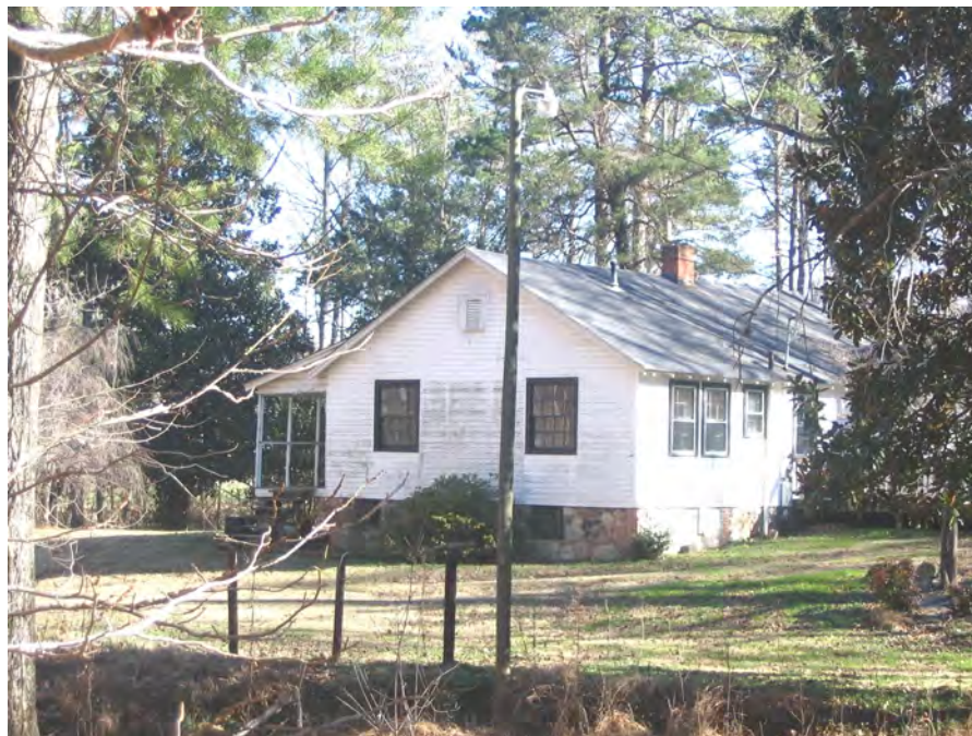
Tenant House, Jake Long Dairy Barn, Looking Northeast.
