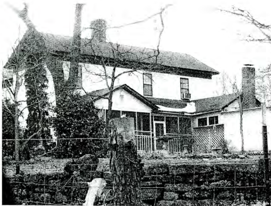
No. 48 Falls House
