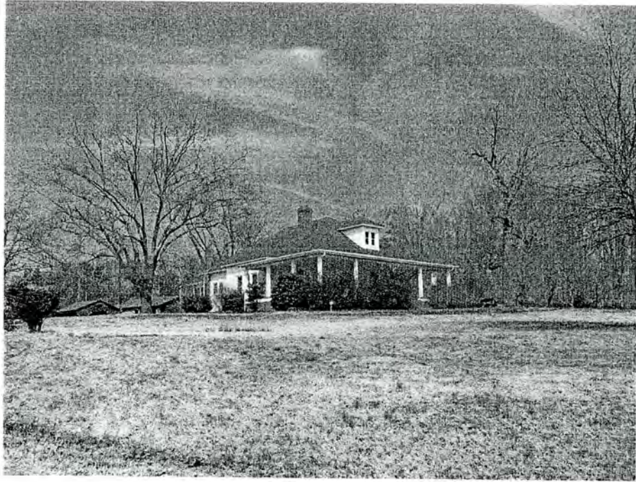
No. 56. Stowe Dairy Farm
