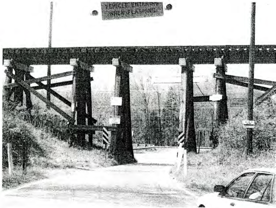
No. 43. Railroad Trestle Bridge
