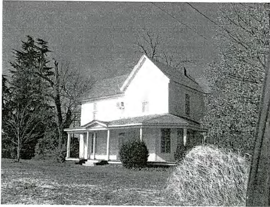
No. 4 Hayes-Byrum House and Store (National Register, Local Landmark)
