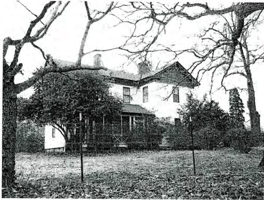
No. 48 Falls House
