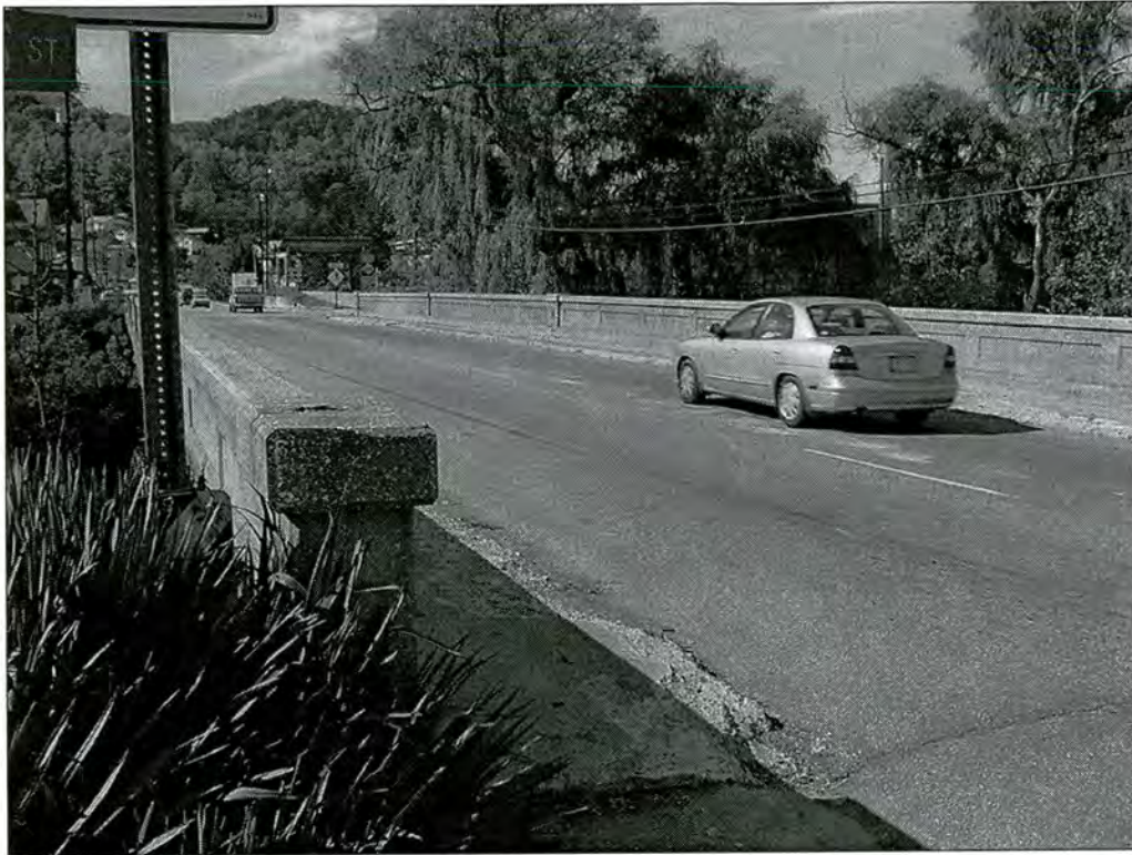
Pigeon River Bridge – view to west
