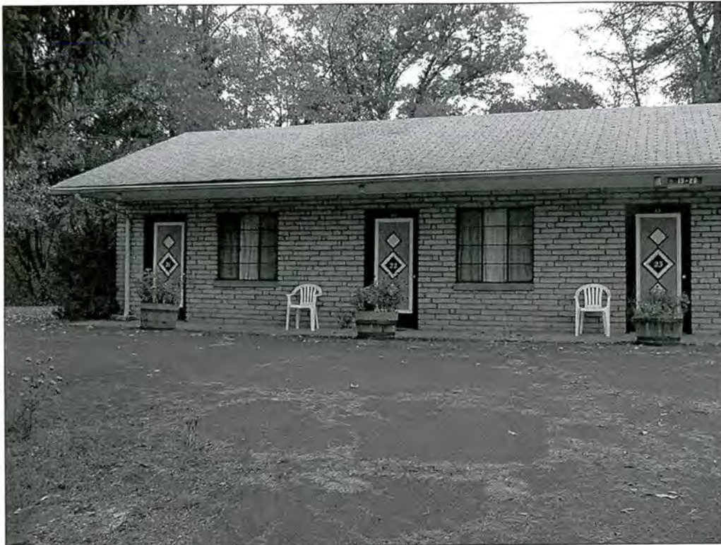
Plantation Motel – detached block of rooms, west end
