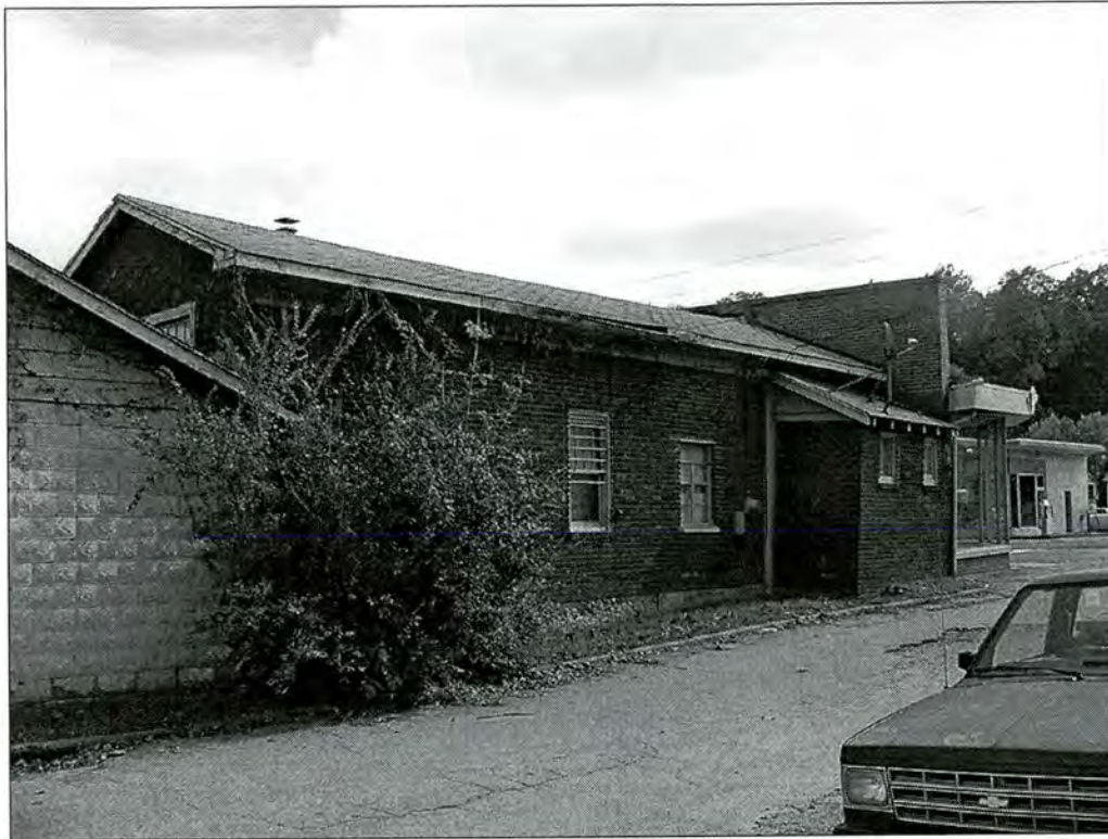
Champion Motor Company – west side elevation (view to southeast)
