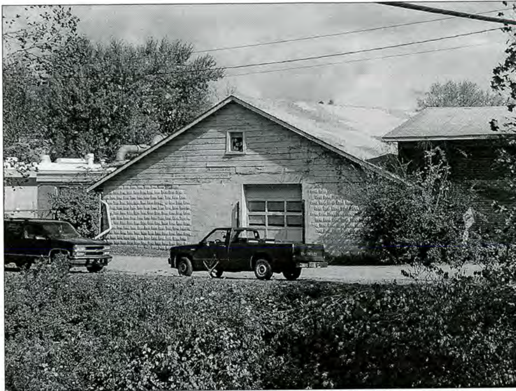
Champion Motor Company – rear west side elevation (original garage)
