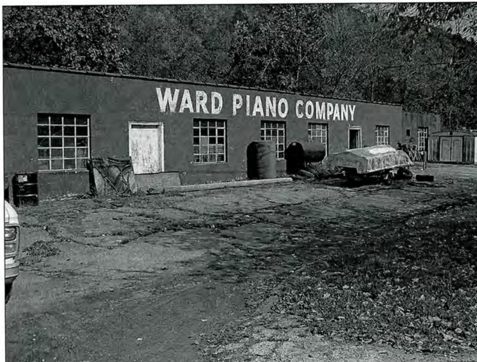
Ward Piano Company (#66) – built 1953; view from southwest
