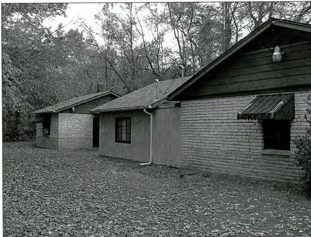
Plantation Motel – detached block of rooms, rear section
