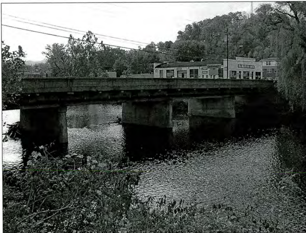
Pigeon River Bridge – view to southeast
