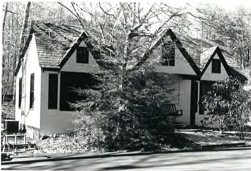
Plate 6. Duvall House and Restaurant Complex, Cottage, Looking West.
