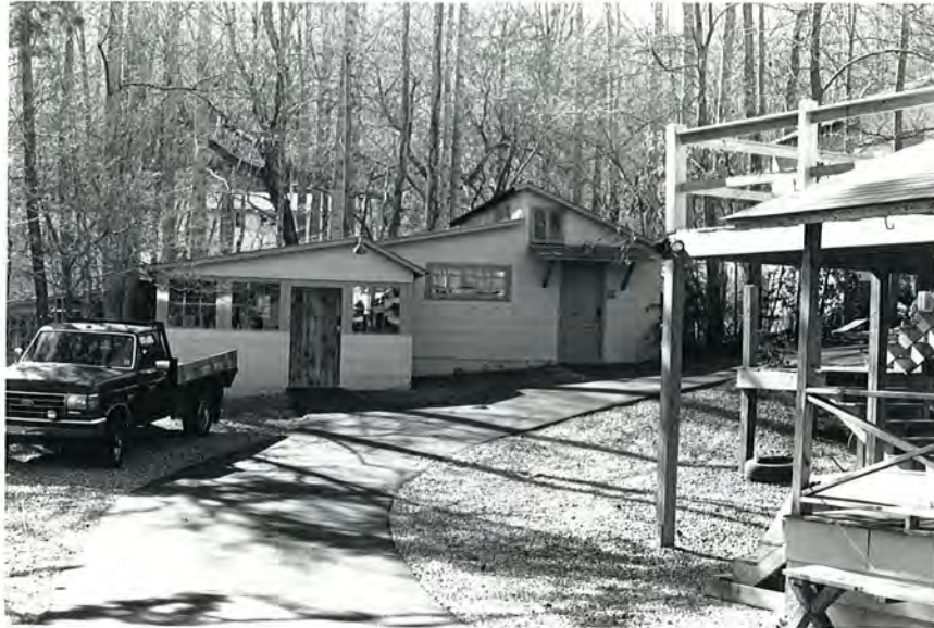
Plate 5. Duvall House and Restaurant Complex, Workshop, Looking West.
