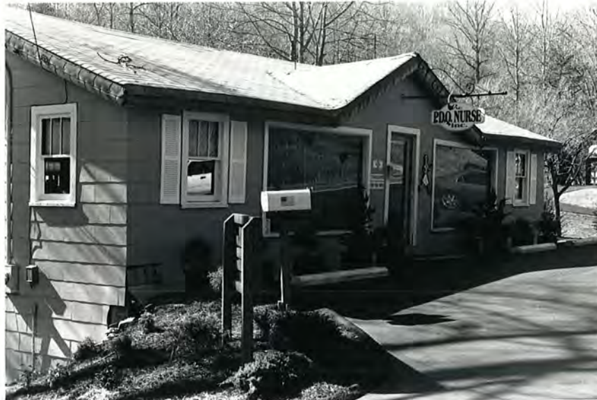
Plate 2. Duvall House and Restaurant Complex, Restaurant, Looking Northwest.
