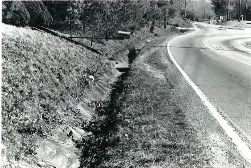
Plate 17. Civilian Conservation Corps, Stone Drainage Ditch System, Segment on the East Side of N.C. 28, North of the Junction with S.R. 1323.
