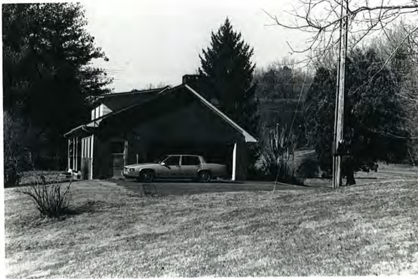
Plate 9. Calloway Farm, Modern House, South Elevation, Looking North.
