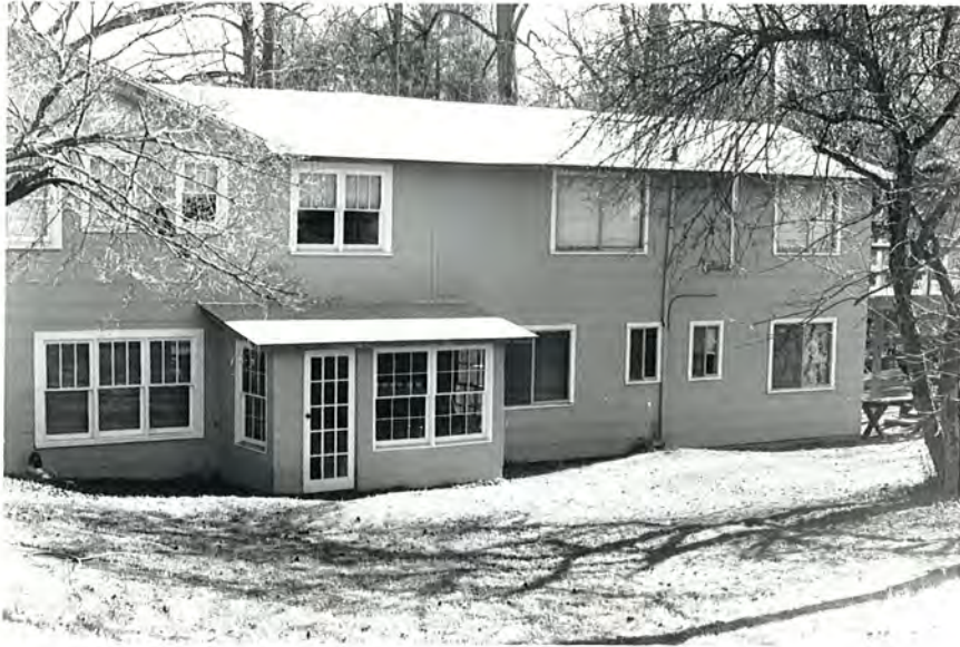
Plate 3. Duvall House and Restaurant Complex, Restaurant, North Elevation (Ell), Looking South.
