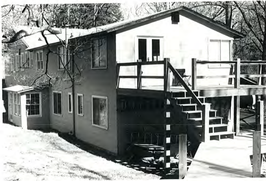
Plate 4. Duvall House and Restaurant Complex, Restaurant, Ell, Looking East.
