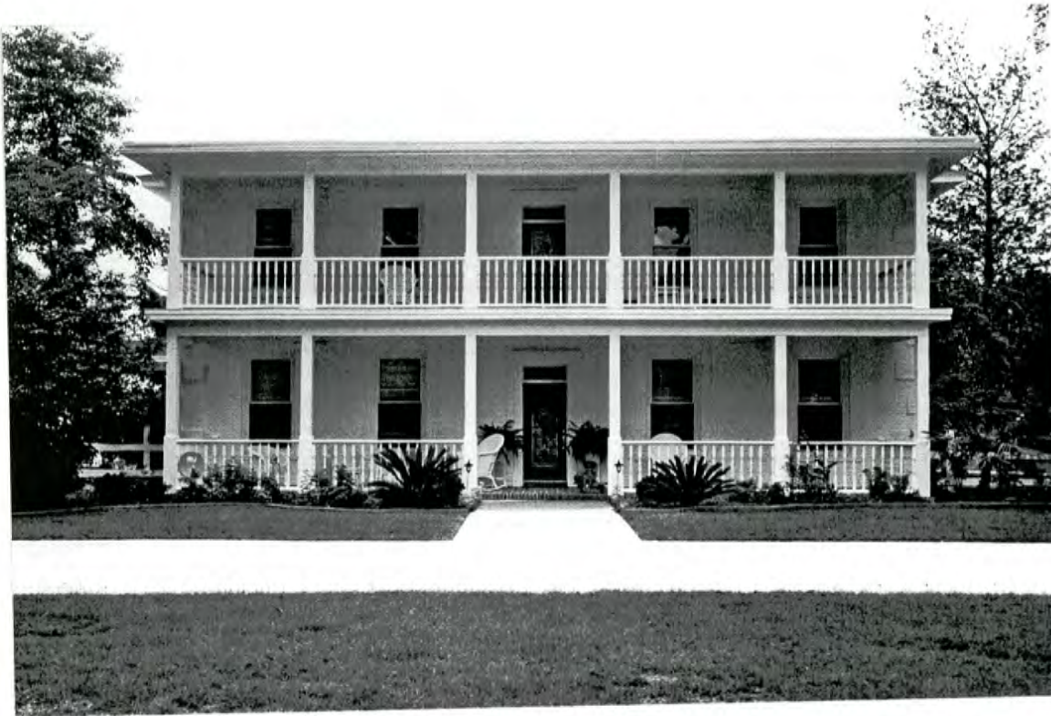
Plate 46: Jackson Brothers Lumber Company Office – west front elevation
