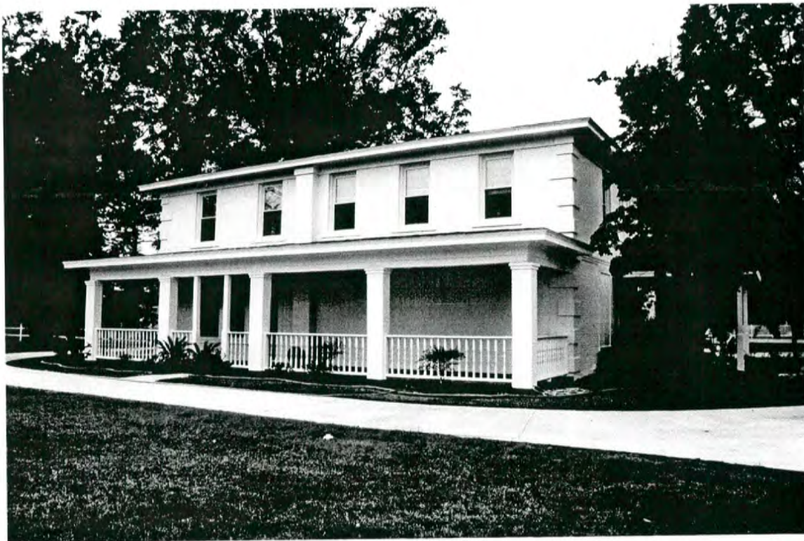
Plate 49: Jackson Brothers Lumber Company Office – east rear and north side elevations
