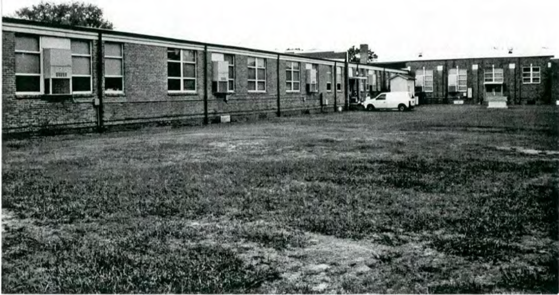
Plate 8: Old Dock Elementary School – rear of 1946 block at left, 1936 auditorium at right, looking northwest
