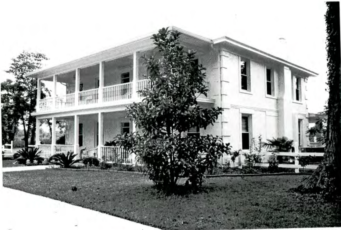
Plate 47: Jackson Brothers Lumber Company Office – west front and south side elevations
