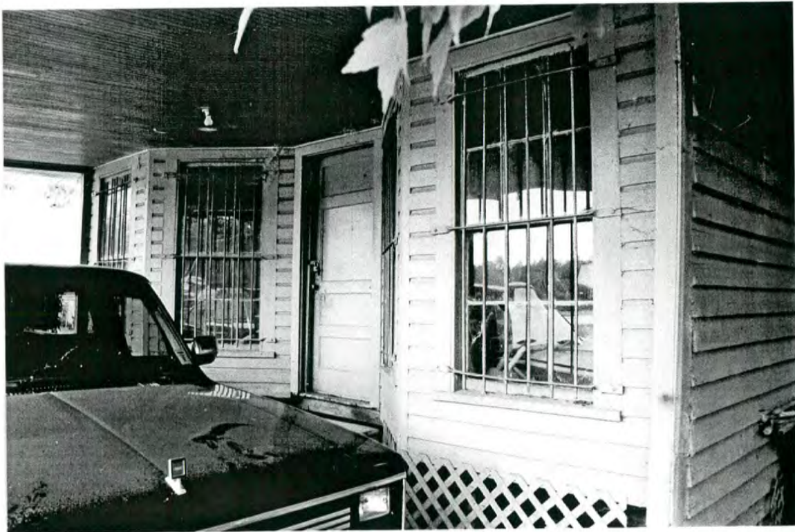
Plate 14: Hill General Store –detail of west front elevation
