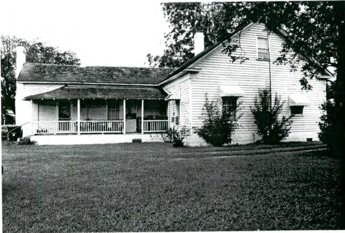
Plate 43: Sasser House— house at right and ell at left, looking north
