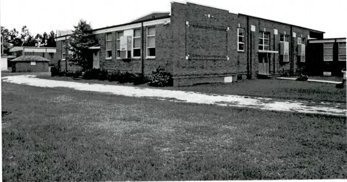
Plate 4: Old Dock Elementary School – auditorium of 1936 block, looking southwest; early brick service building at far left
