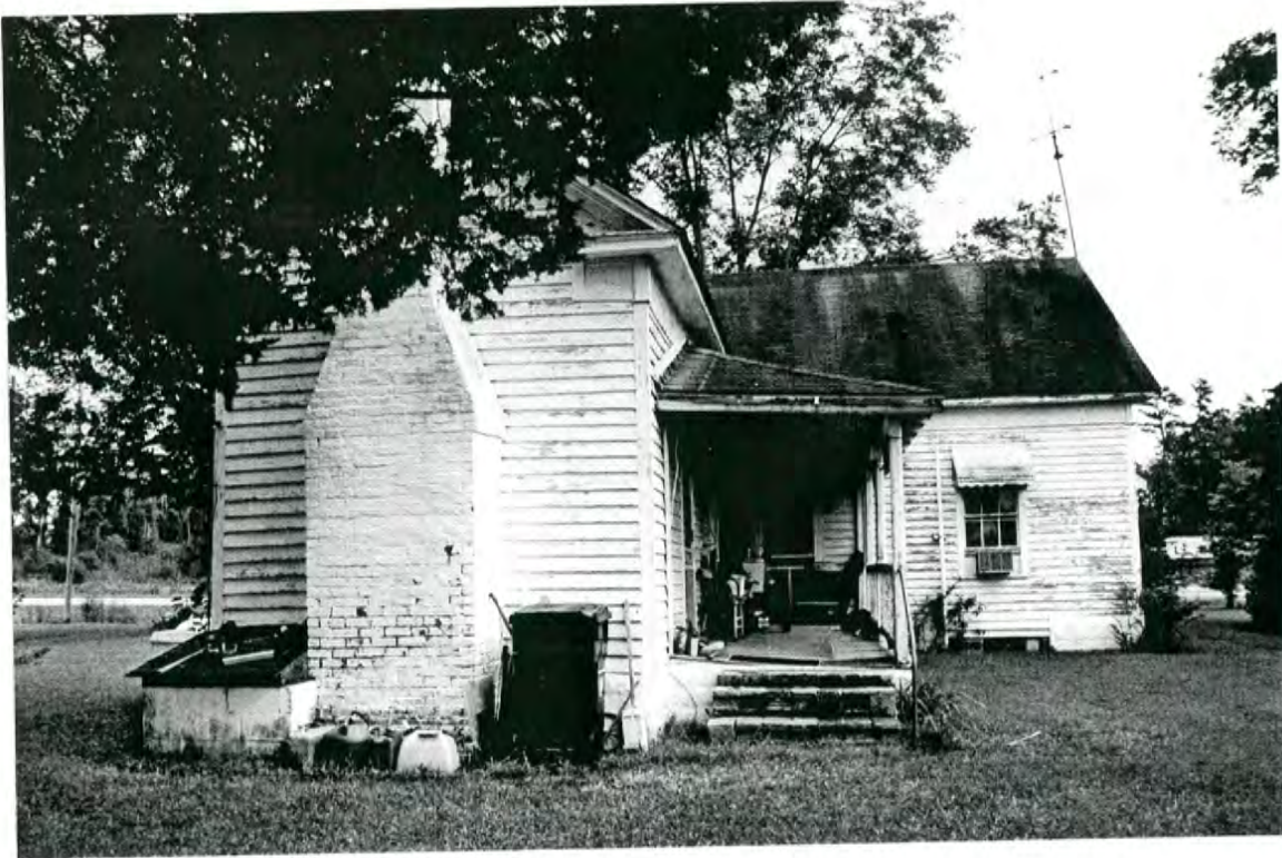
Plate 44: Sasser House— west elevation of ell at left and house at right, looking east
