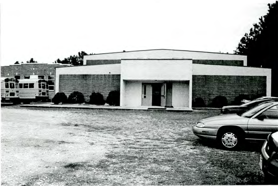
Plate 10: Old Dock Elementary School –west front elevation of 1984 gymnasium at center and 1946 block at far left
