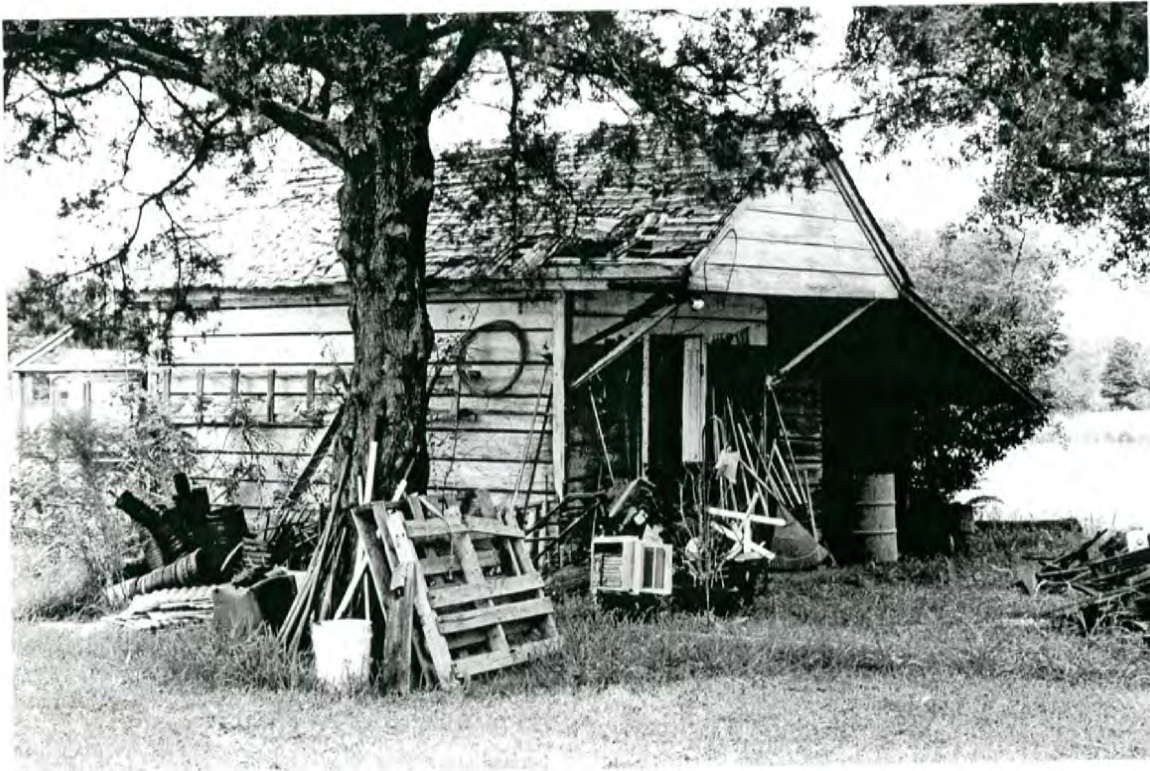
Plate 45: Sasser House— shed, looking northwest
