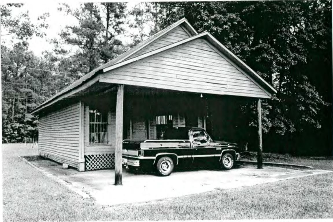
Plate 11: Hill General Store – west front and north side elevations
