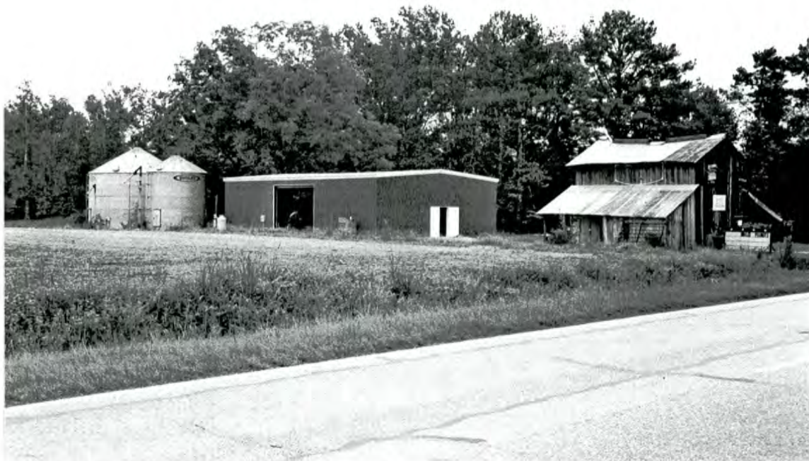
Plate 39: Calvin C. Gore House - grain bins at left, peanut building at center, and tobacco barn at right, looking southeast from NC 130
