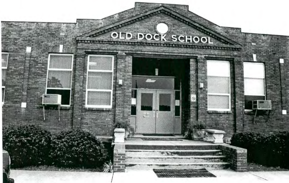
Plate 3: Old Dock Elementary School – main entry, 1936 block
