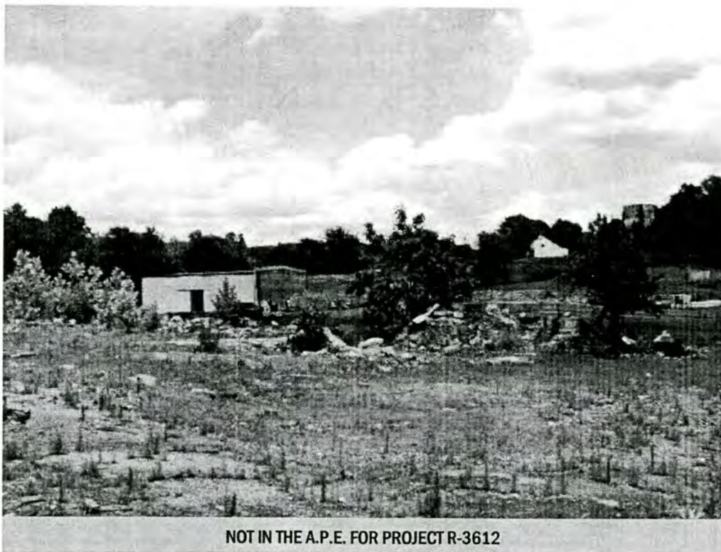
Section V. / Fig. 5: Site of Henrietta Mill No. 1 (demolished) Henrietta, NC
